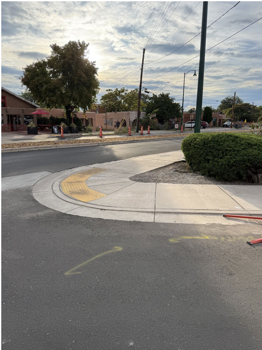
Johnson St crossing looking west:
