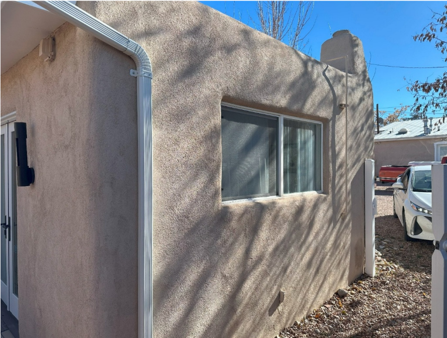
View from North looking West Elevation. Note chimney is at South end of this elevation. This chimney is also seen on left side of South elevation.
