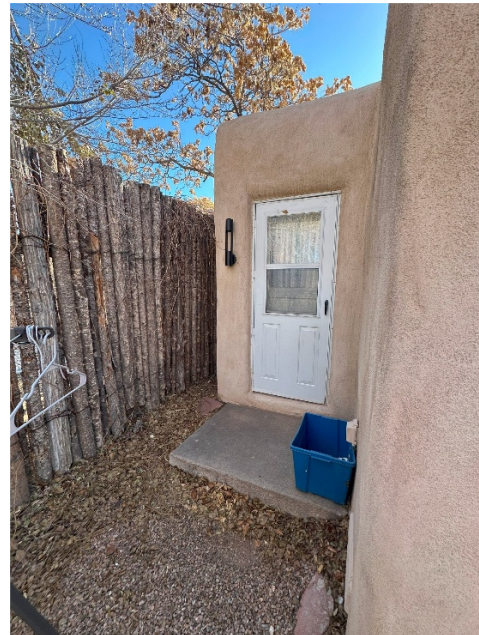
View of REMAINDER NORTH ELEVATION
