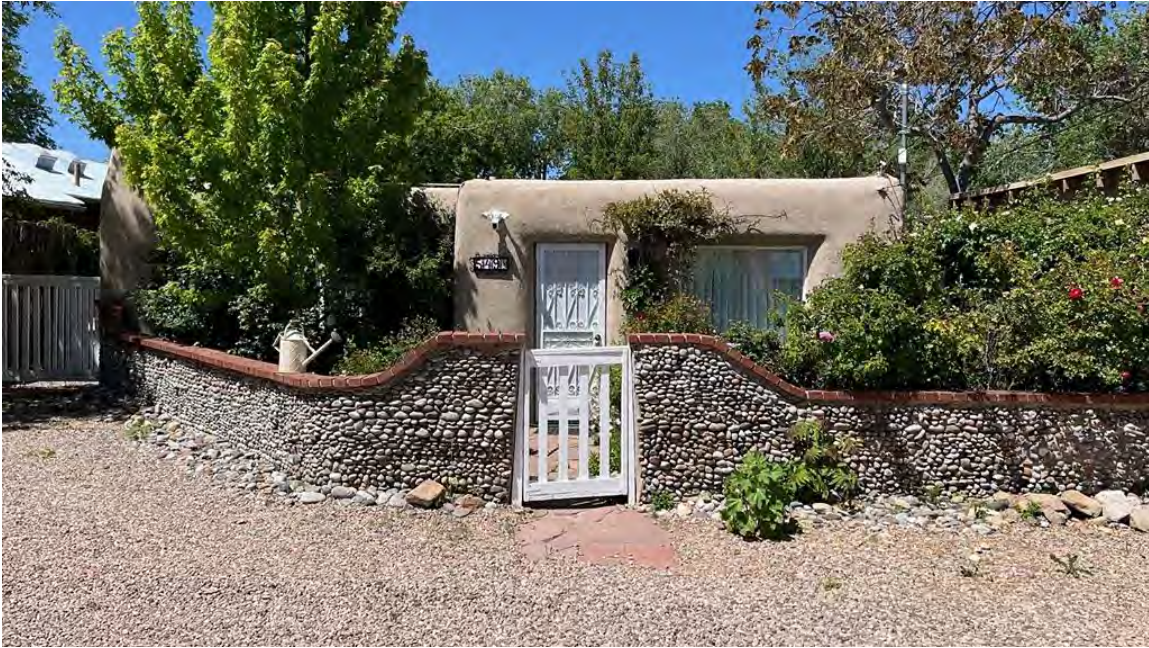
Photo 4: Subject dwelling and context. Camera facing north.
