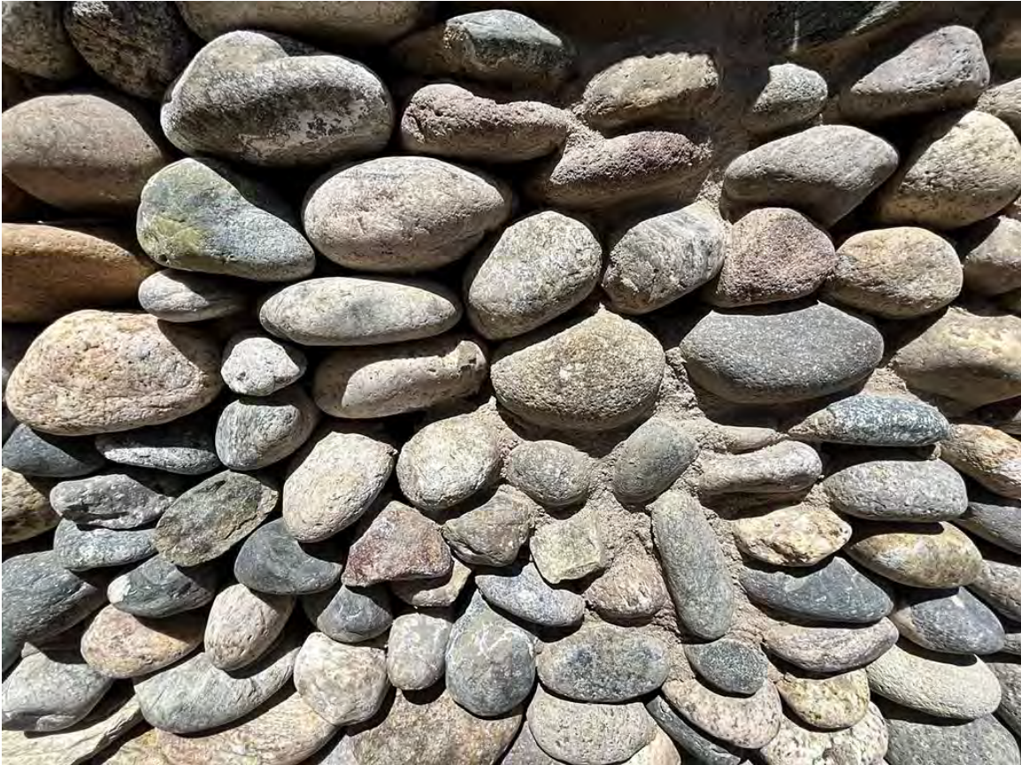
Photo 14: Front Garden Wall. Detail of masonry. Camera facing north.
