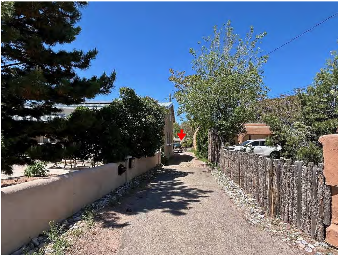
Photo 2: View of Hesch-Gonzales Cottage (arrow) from north side on Agua Fria Street. Camera facing north.
