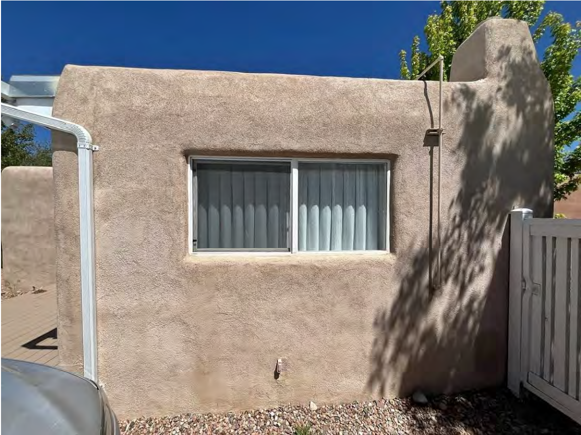
Photo 7: West elevation. Window in 1960s addition. Camera facing east.
