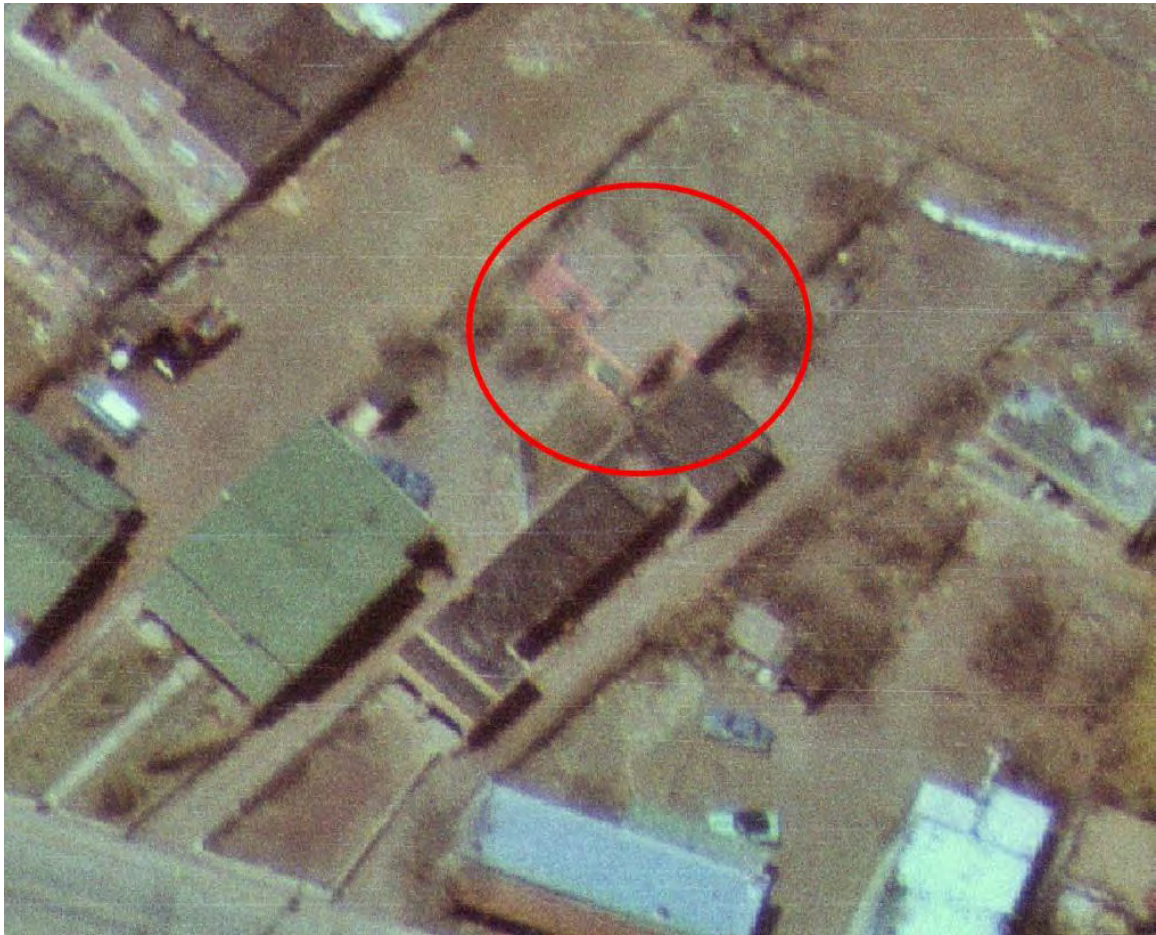
Figure 6: February 27, 1969, aerial photograph. Former garage has expanded to the west with an addition reflecting its use during the Maude Gonzales period.
