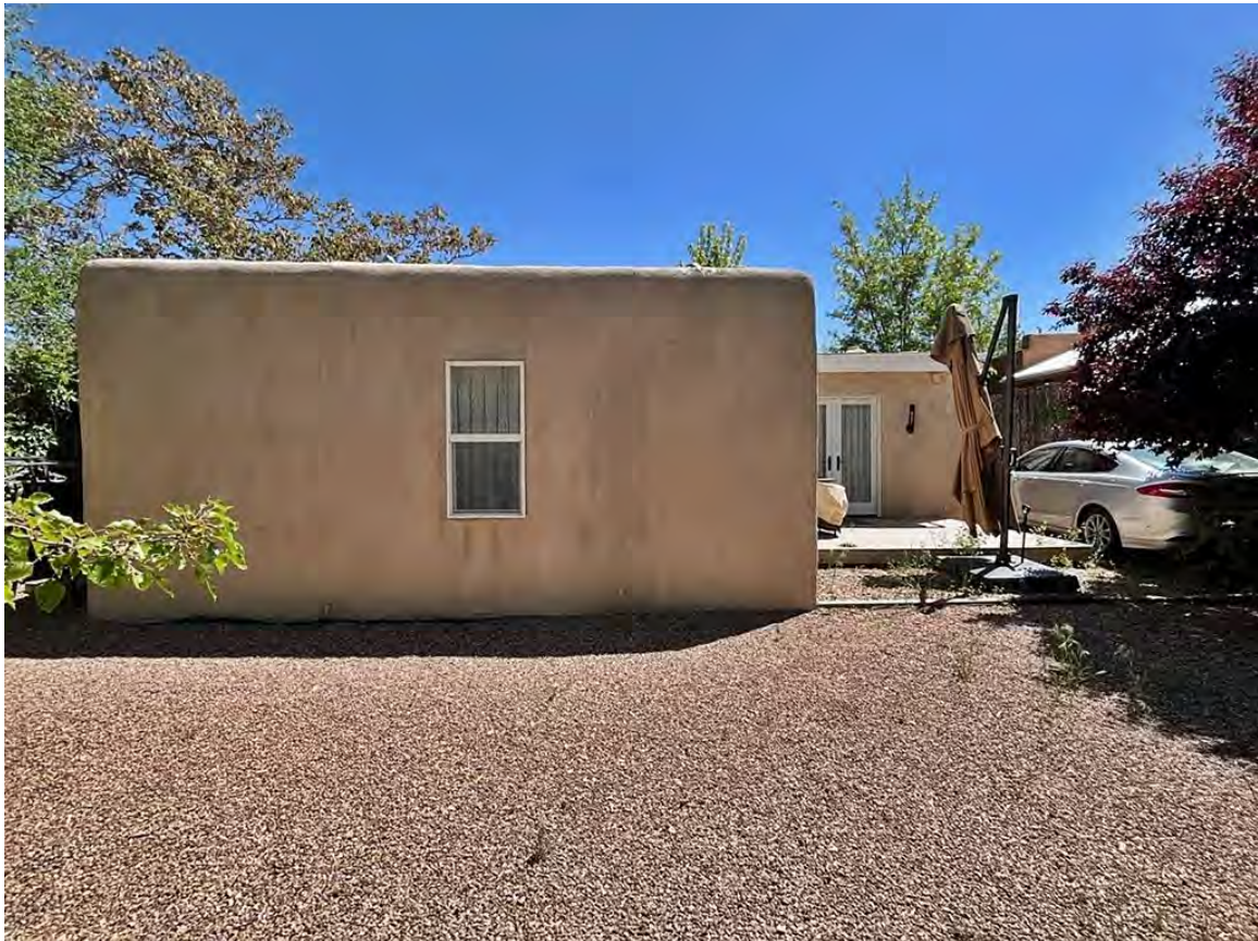
Photo 9: North elevation. Camera facing south.
