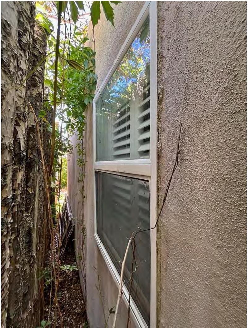
Photo 13: East elevation. Window in 1940s addition. Camera facing southwest.
