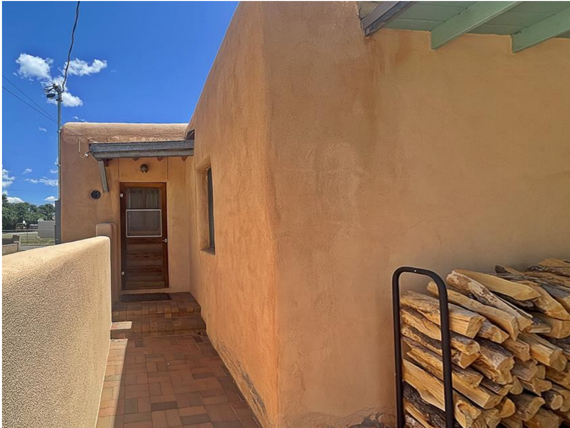
Photo 8: West elevation. Laundry room. Camera facing east.
