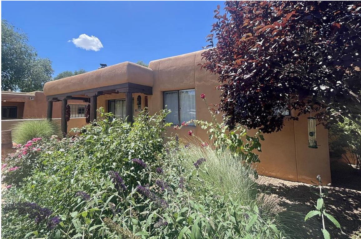
Photo 5: East (front) façade. Camera facing southwest.
