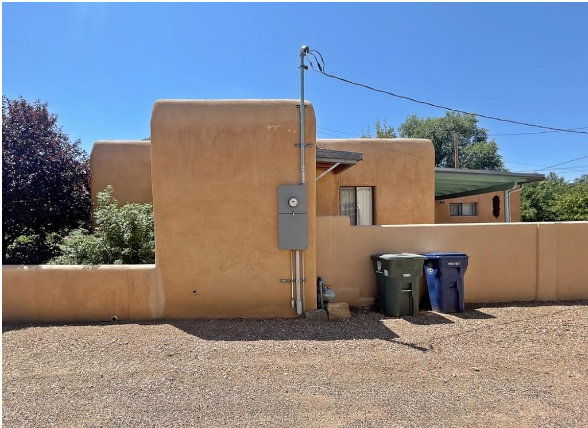
Photo 7: North elevation. Camera facing south.
