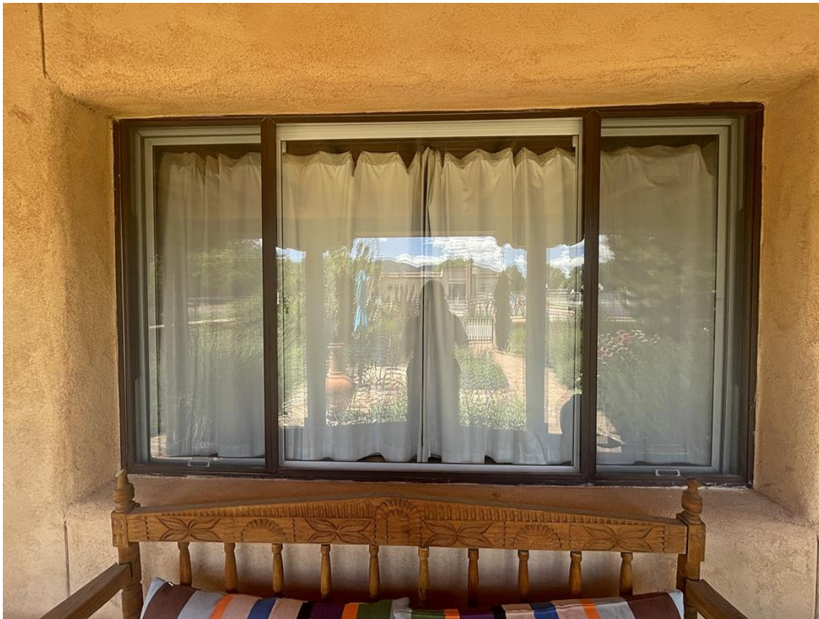
Photo 3: East (front) façade. Replaced window at portal. Camera facing west.
