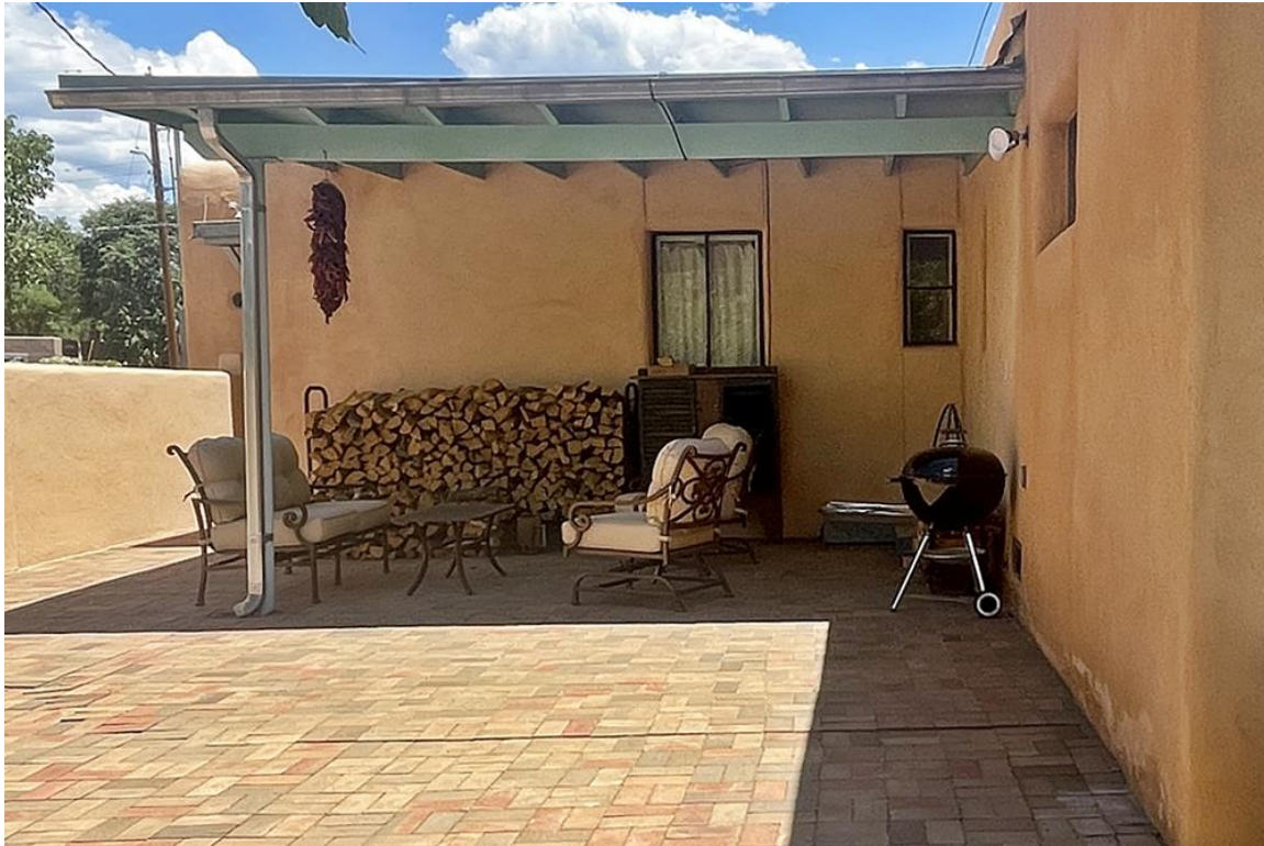
Photo 10: West elevation. Original section. Camera facing east.
