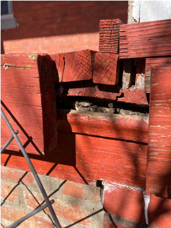
Item #3: safety replacement of deck. Exhibit 3A and 3B
