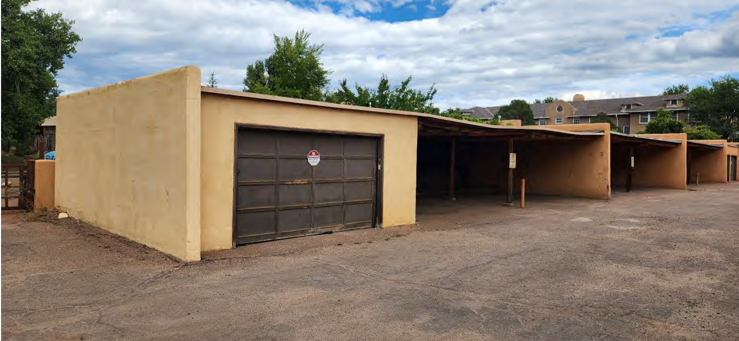
South Elevation (Garage & Carport)
