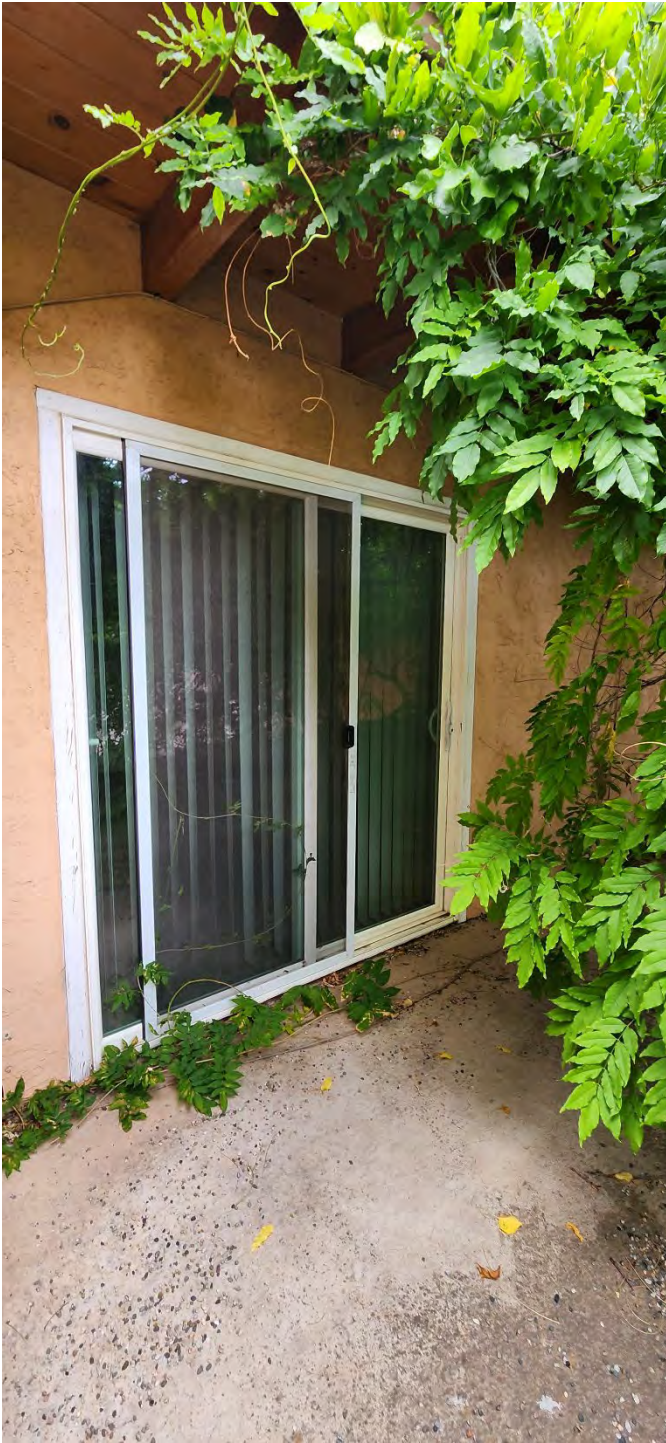
South Elevation (West end)
