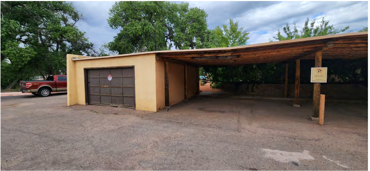
South Elevation (Garage & Carport)
