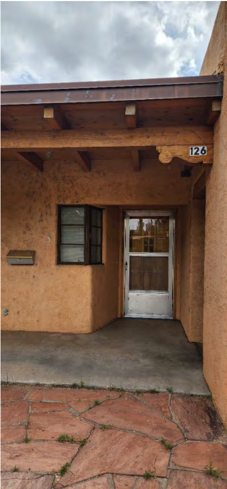
North Elevation (West entry door at Portal)
