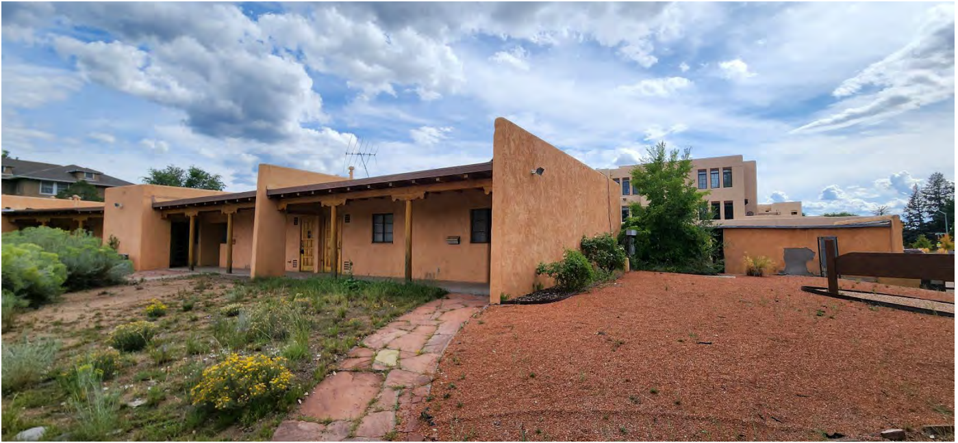
North Elevation (Looking Southeast and End Wall)
