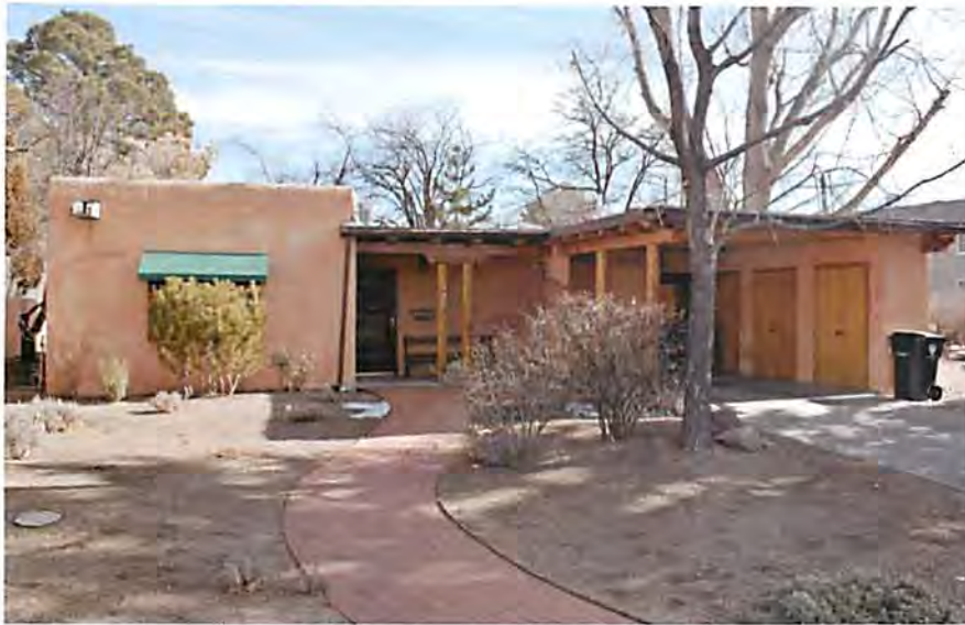
Figure 12: 120 Camino Santiago, constructed in c. 1971.
