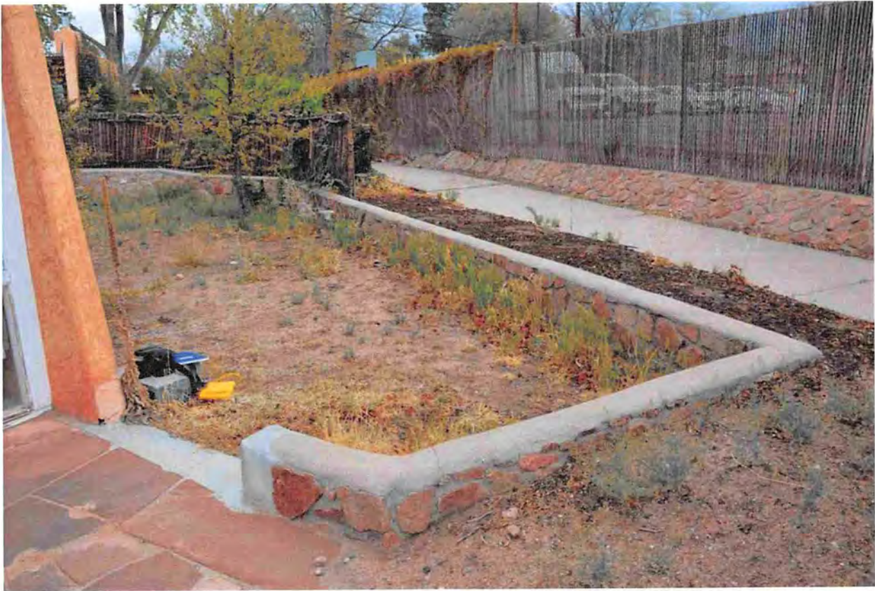
Figure 2: 124 Camino Santiago, rear retaining wall, May 3, 2018.
