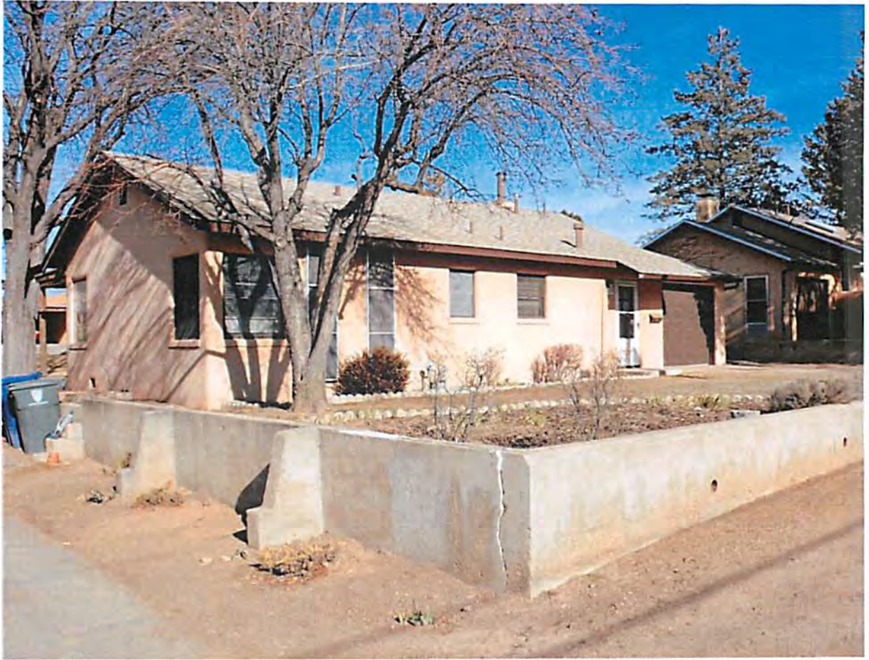
Figure 3: c.1950 concrete retaining in front of 107 Camino Matias. January 18, 2018.
