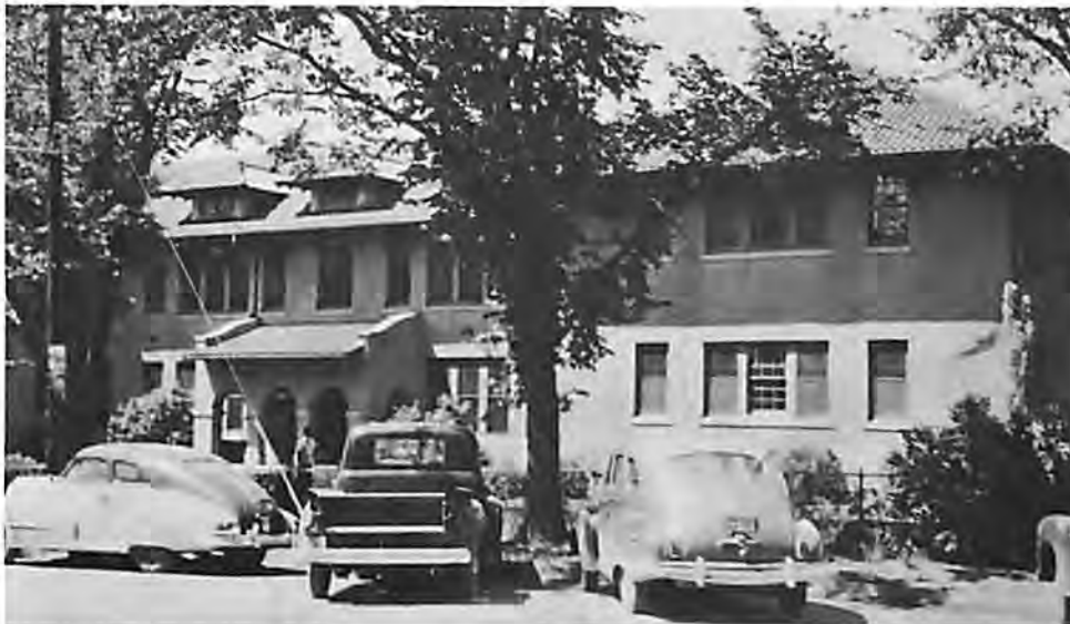
Figure 2: The Margaret Olivia Sage Hall, demolished in 1960 to construct Plaza del Monte. Source: Atkins, 1983.
