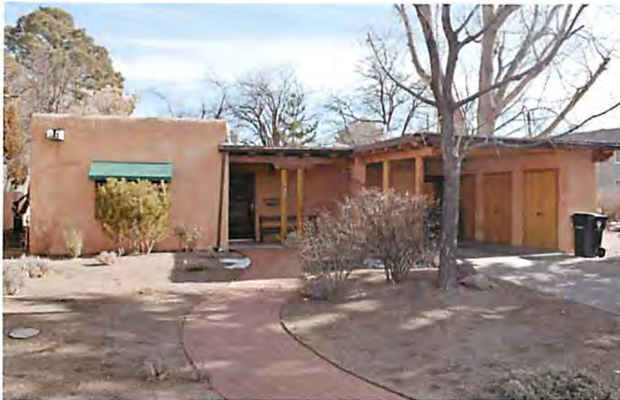
Figure 12: 120 Camino Santiago, constructed in c. 1971.
