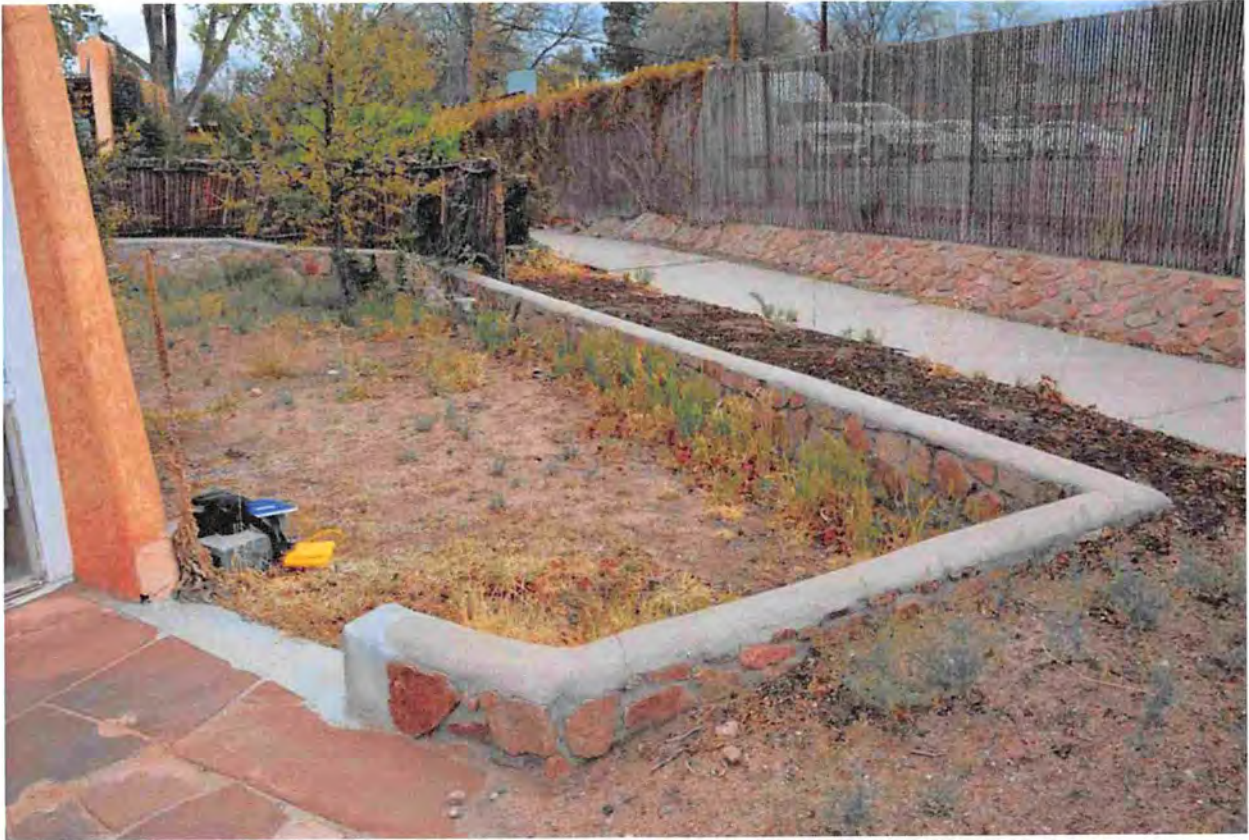
Figure 2: 124 Camino Santiago, rear retaining wall, May 3, 2018.
