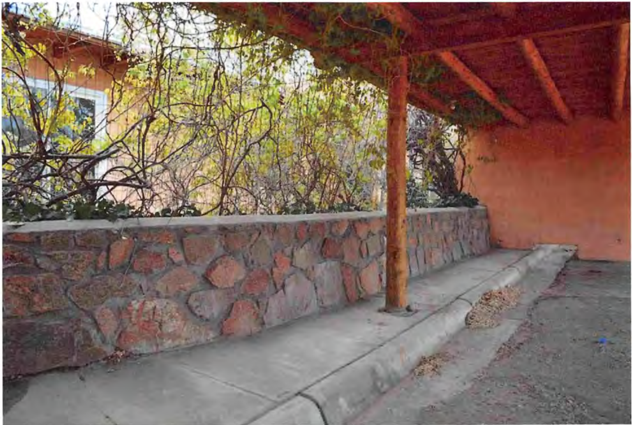
Photo 4: Retaining wall between apartment and parking structure, facing northeast. May 3, 2018.
