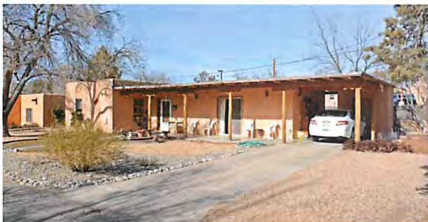
Figure 7: 111 Camino Santiago, an example of Philippe Register's transitional work.
