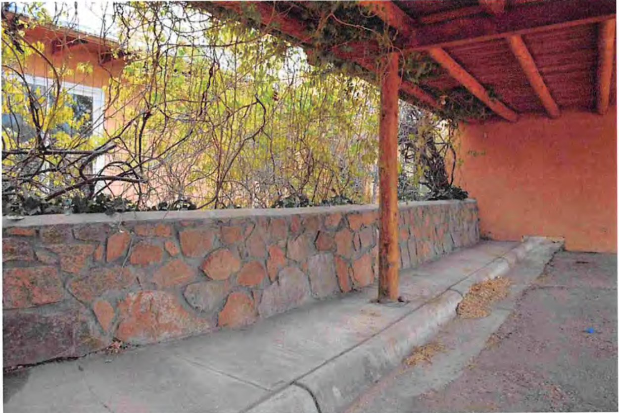
Figure 1: 126 A Camino Santiago, Garage/Carpport Structure, retaining wall, May 3, 2018.
