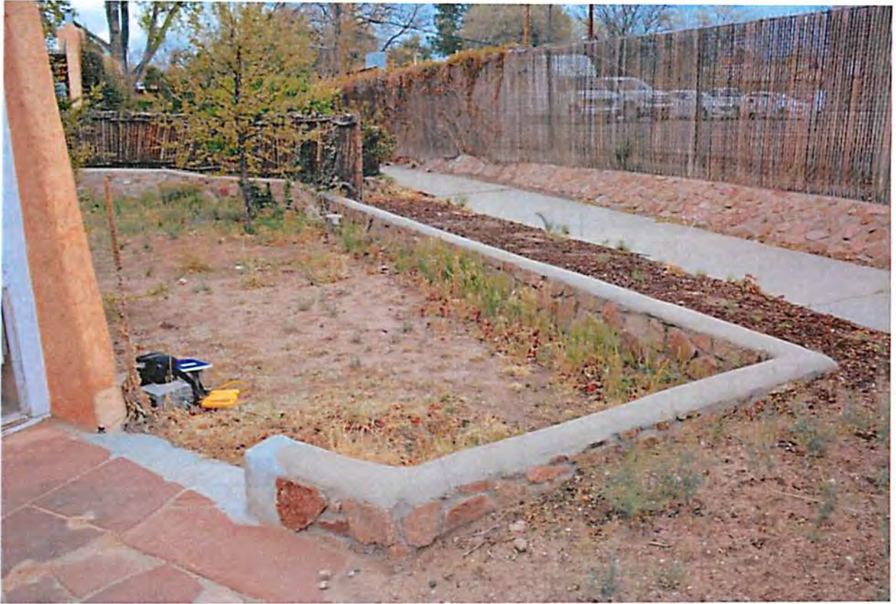
Figure 2: 124 Camino Santiago, rear retaining wall, May 3, 2018.
