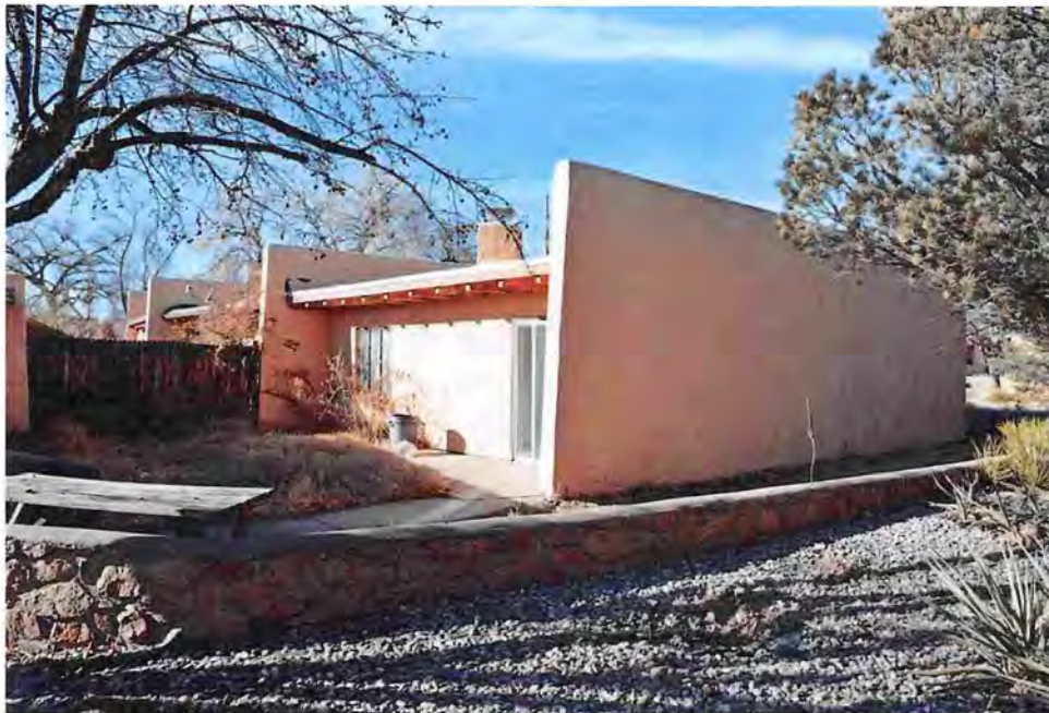
Photo 2: East and south elevations, facing northwest. Low wall in foreground.
