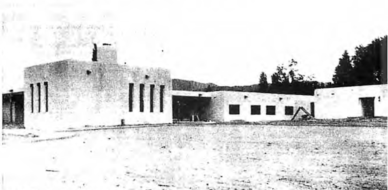
Figure 3: Casa Grande under construction, showing original south façade, May 1961. Courtesy San Fe New Mexican .
