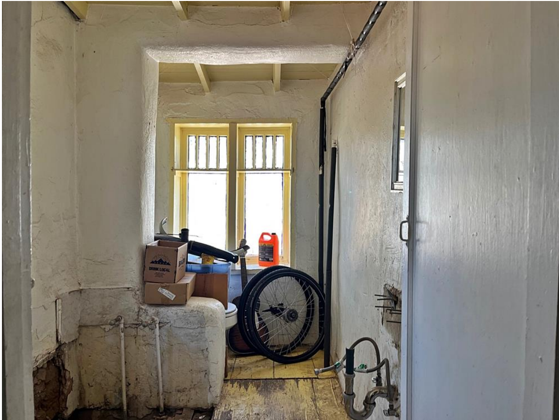
Photo 20: Building #1. Interior of bathroom hall. Camera facing north.
