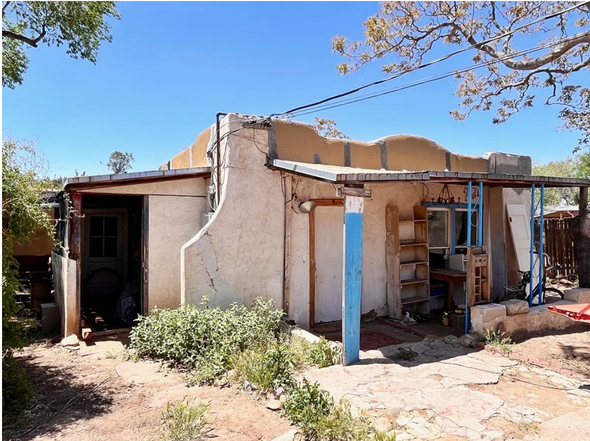
Photo 29: Building #3. East elevation. Camera facing northwest.
