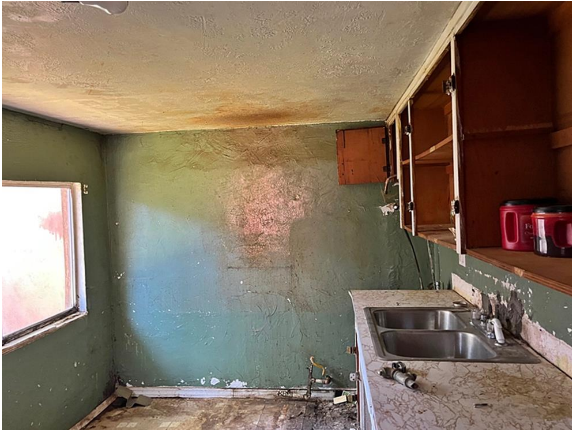
Photo 43: Building #3. Interior of kitchen. Camera facing west.
