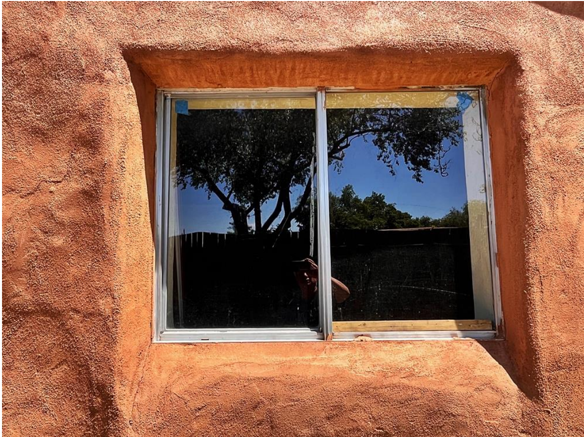
Photo 13: Building #1. West elevation. South window. Camera facing east.
