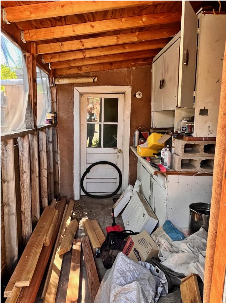
Photo 33: Building #3. East elevation. Outdoor kitchen addition. Camera facing west.
