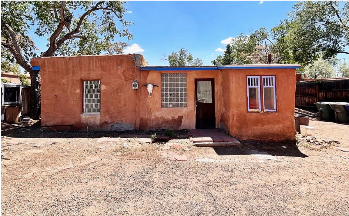
Photo 7: Building #1. North elevation. Camera facing south.
