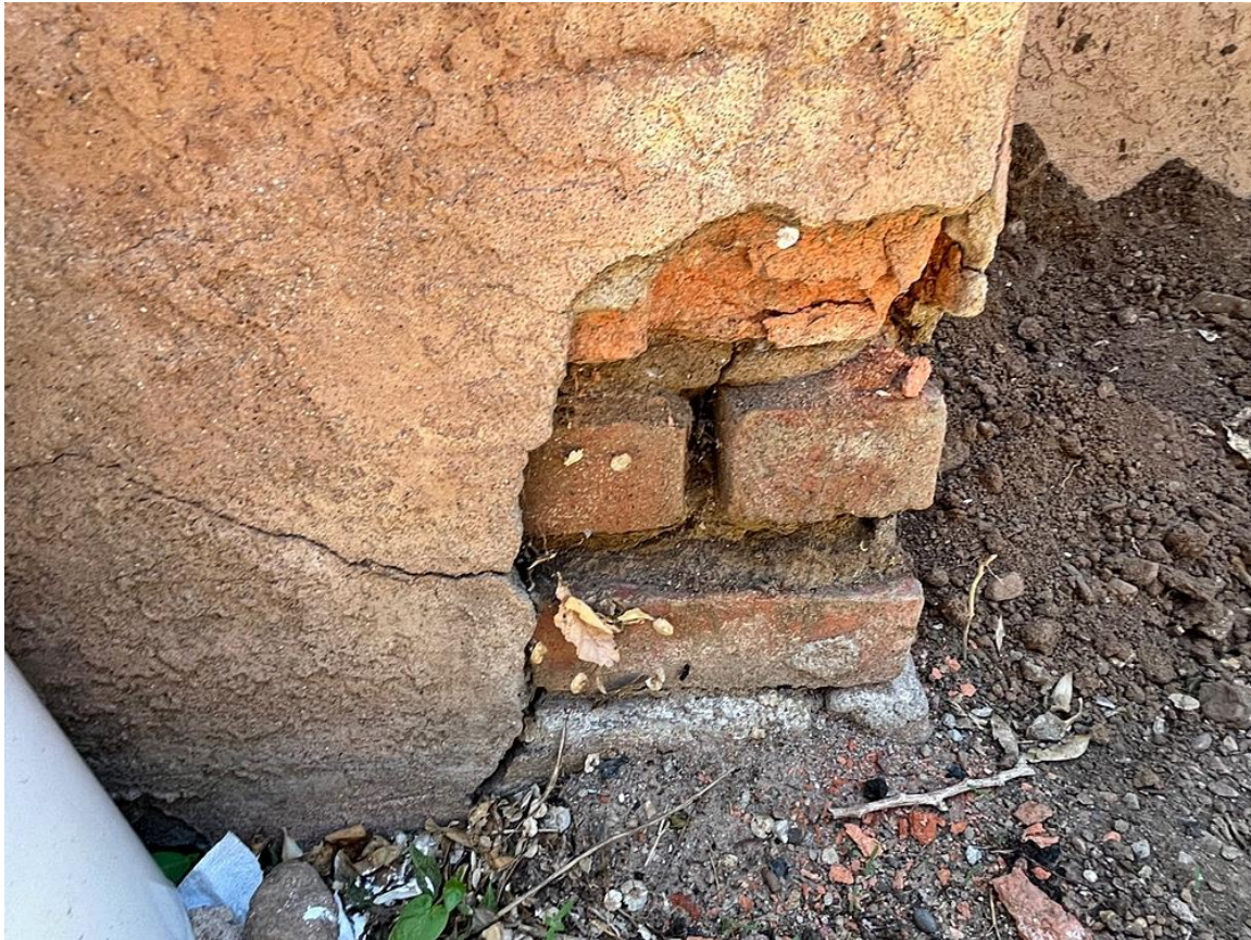
Photo 35: Building #3. North elevation. Exposed brick at chimney. Camera facing down.
