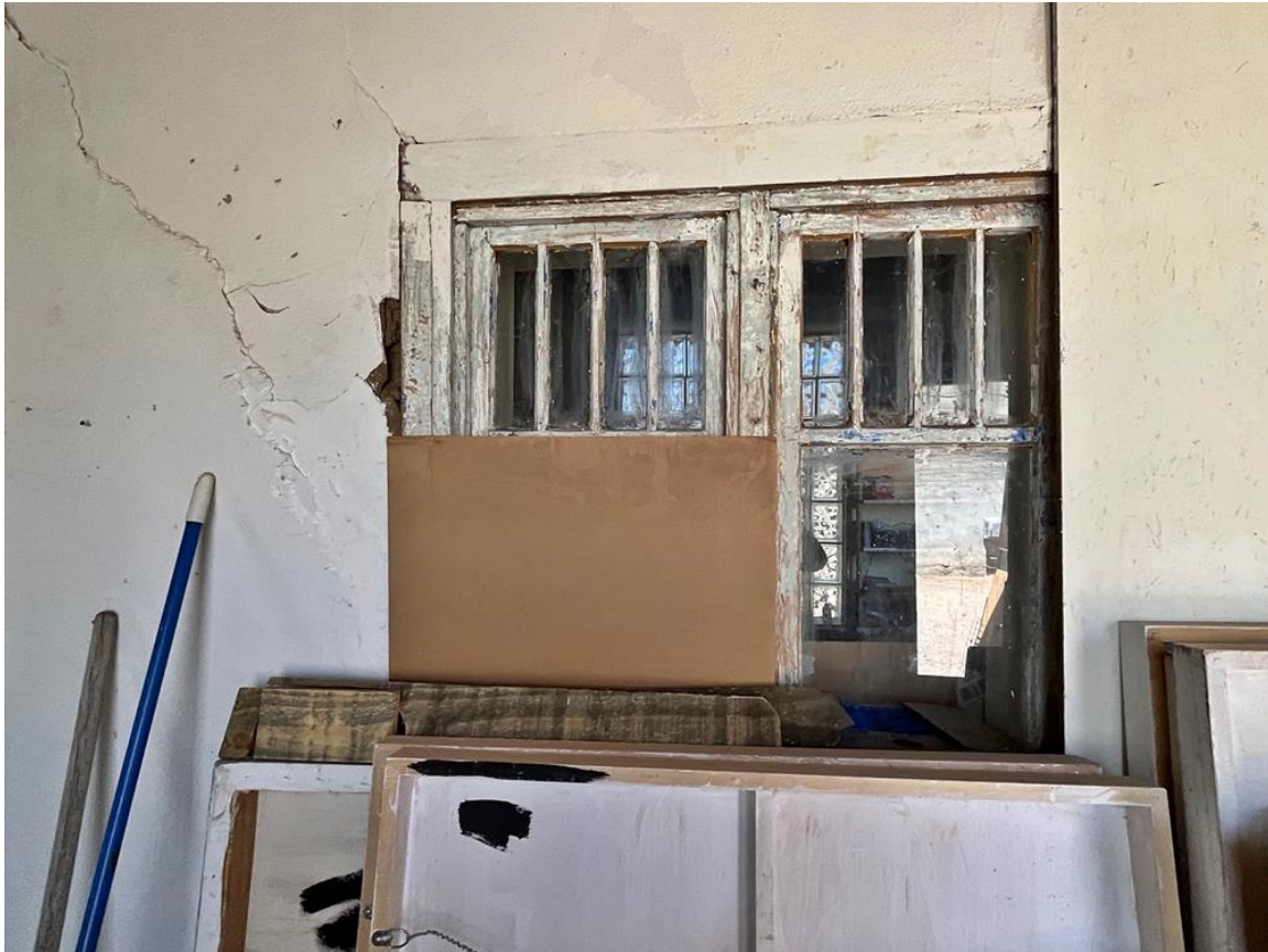
Photo 16: Building #1. Interior of enclosed porch. Camera facing south.
