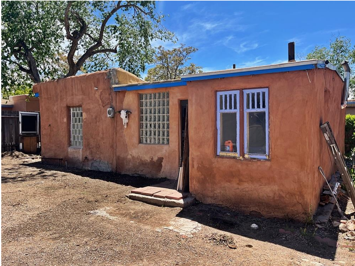
Photo 9: Building #1. North elevation. Bathroom addition on the right. Camera facing northeast.
