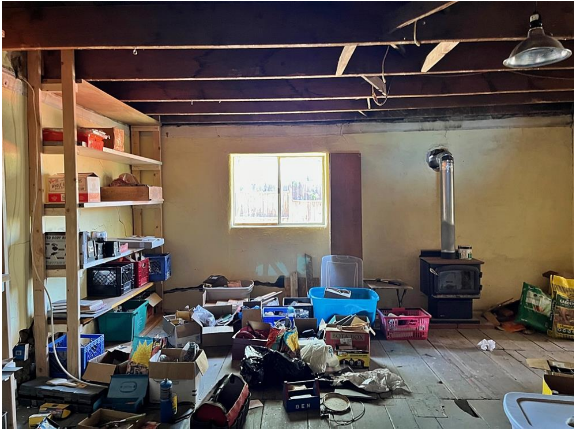
Photo 17: Building #1. Interior of southwest room. Camera facing west.
