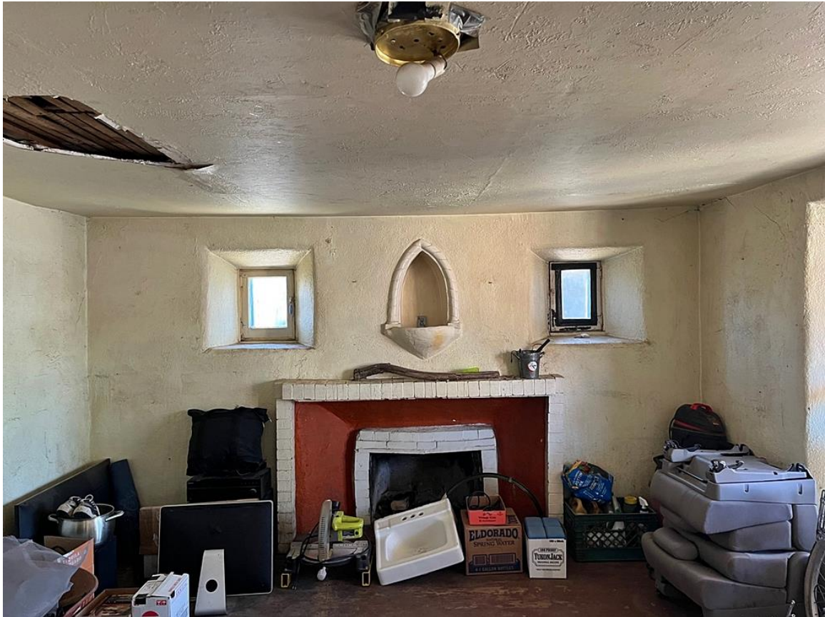
Photo 40: Building #3. Interior of living room. Camera facing north.
