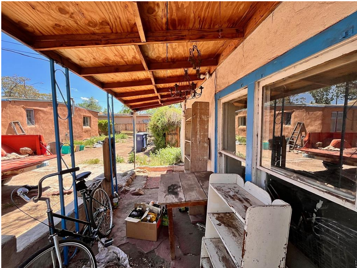
Photo 30: Building #3. East elevation. Porch. Camera facing south.
