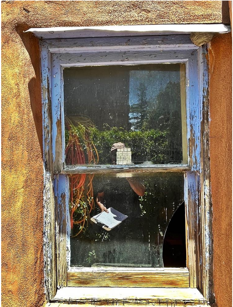
Photo 15: Building #1. South elevation. East window. Camera facing north.
