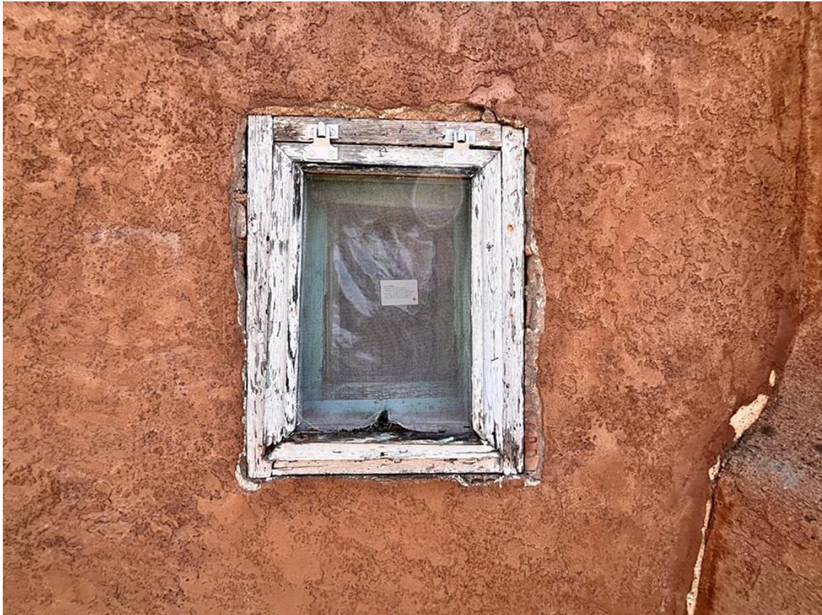
Photo 36: Building #3. North elevation. Window east of chimney. Camera facing south.
