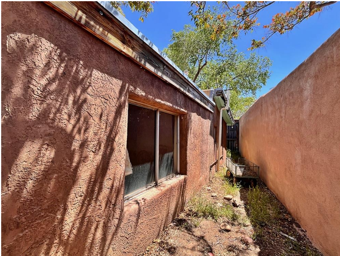
Photo 38: Building #3. West elevation. Camera facing south.
