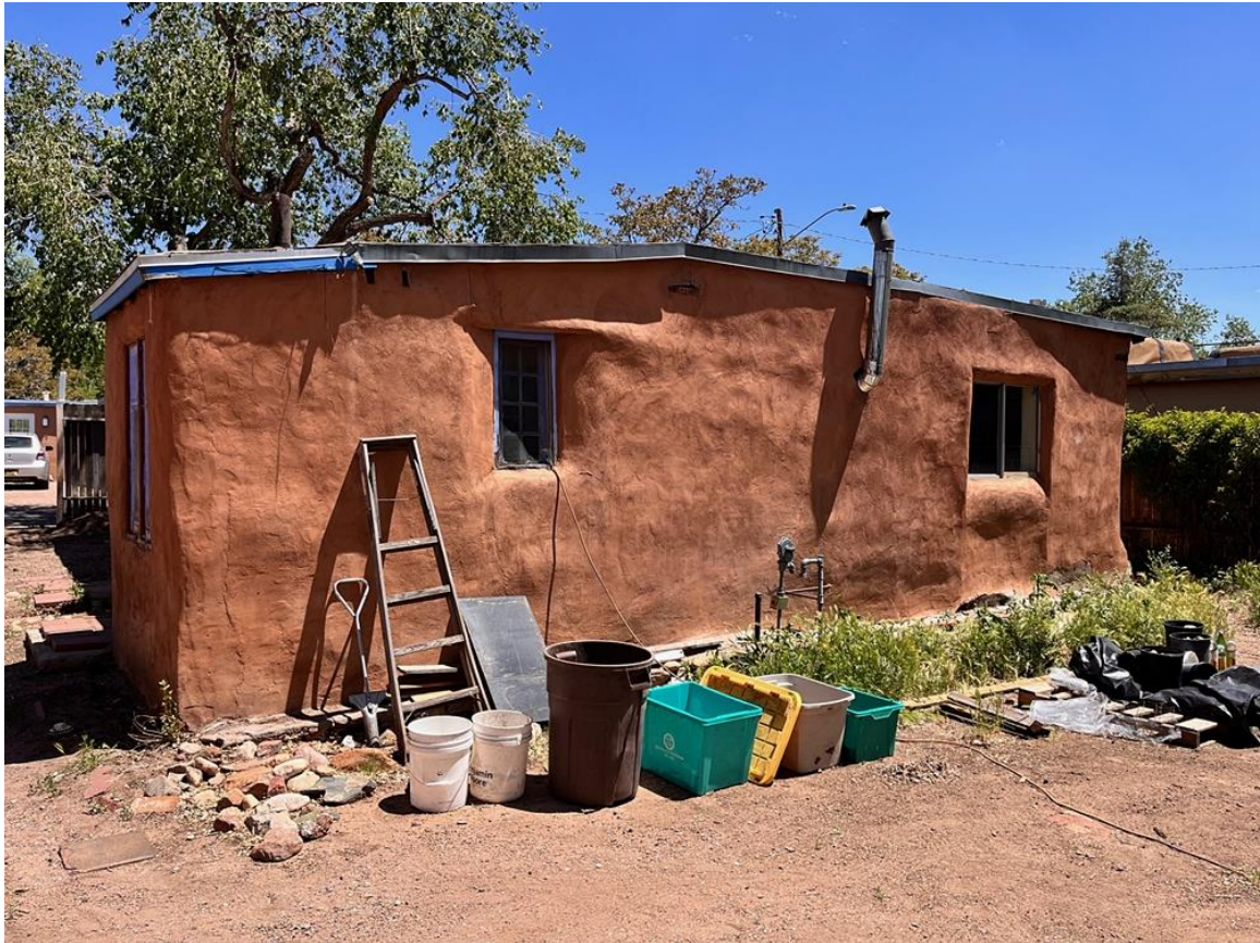
Photo 11: Building #1. West elevation. Camera facing northeast.
