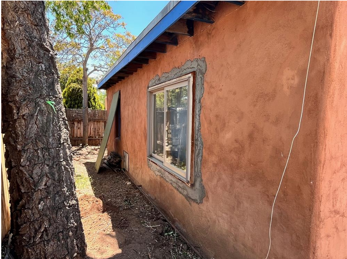
Photo 3: Building #1. East elevation. Camera facing southeast.
