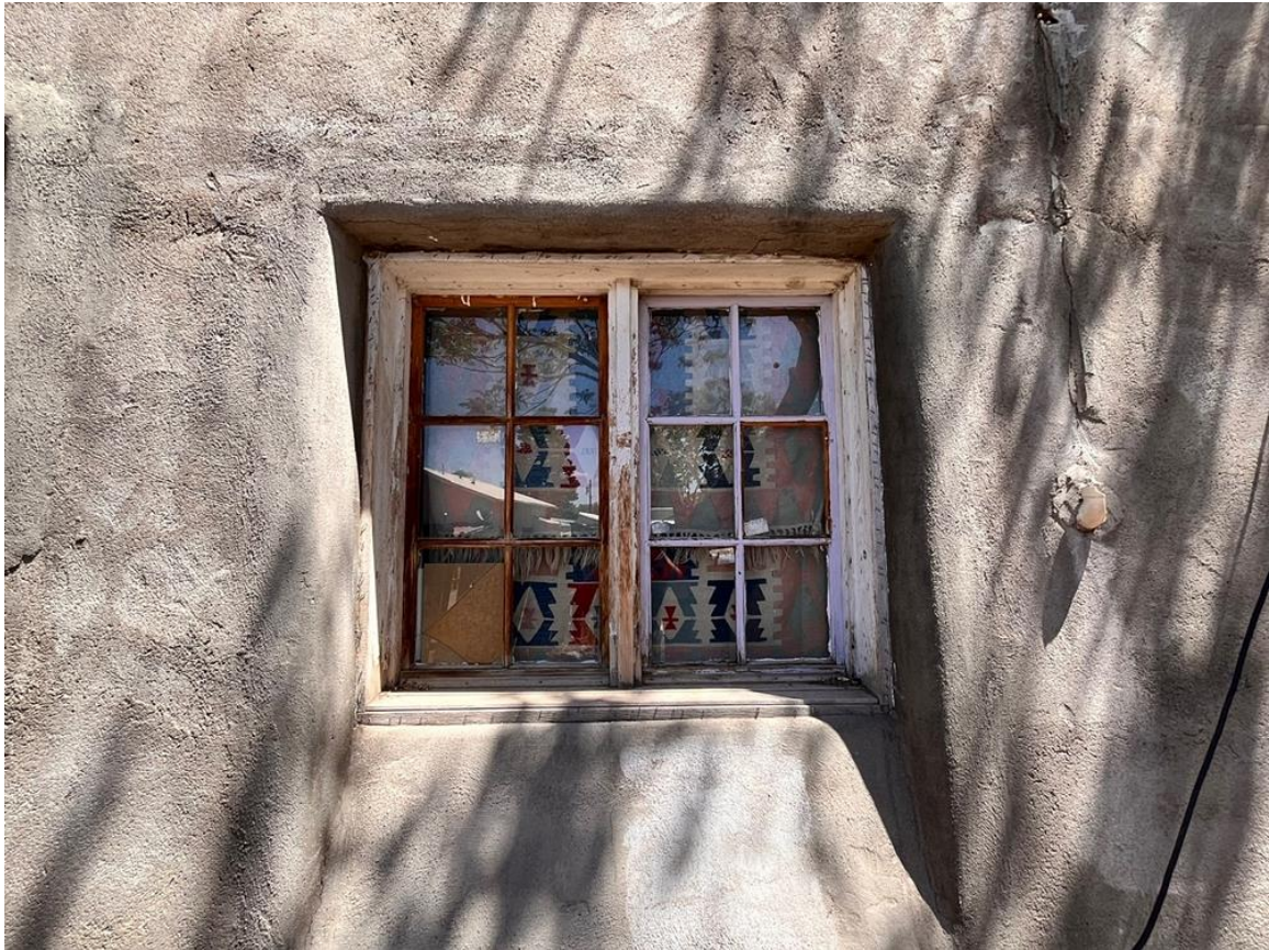
Photo 27: Building #2. West elevation. South window. Camera facing east.
