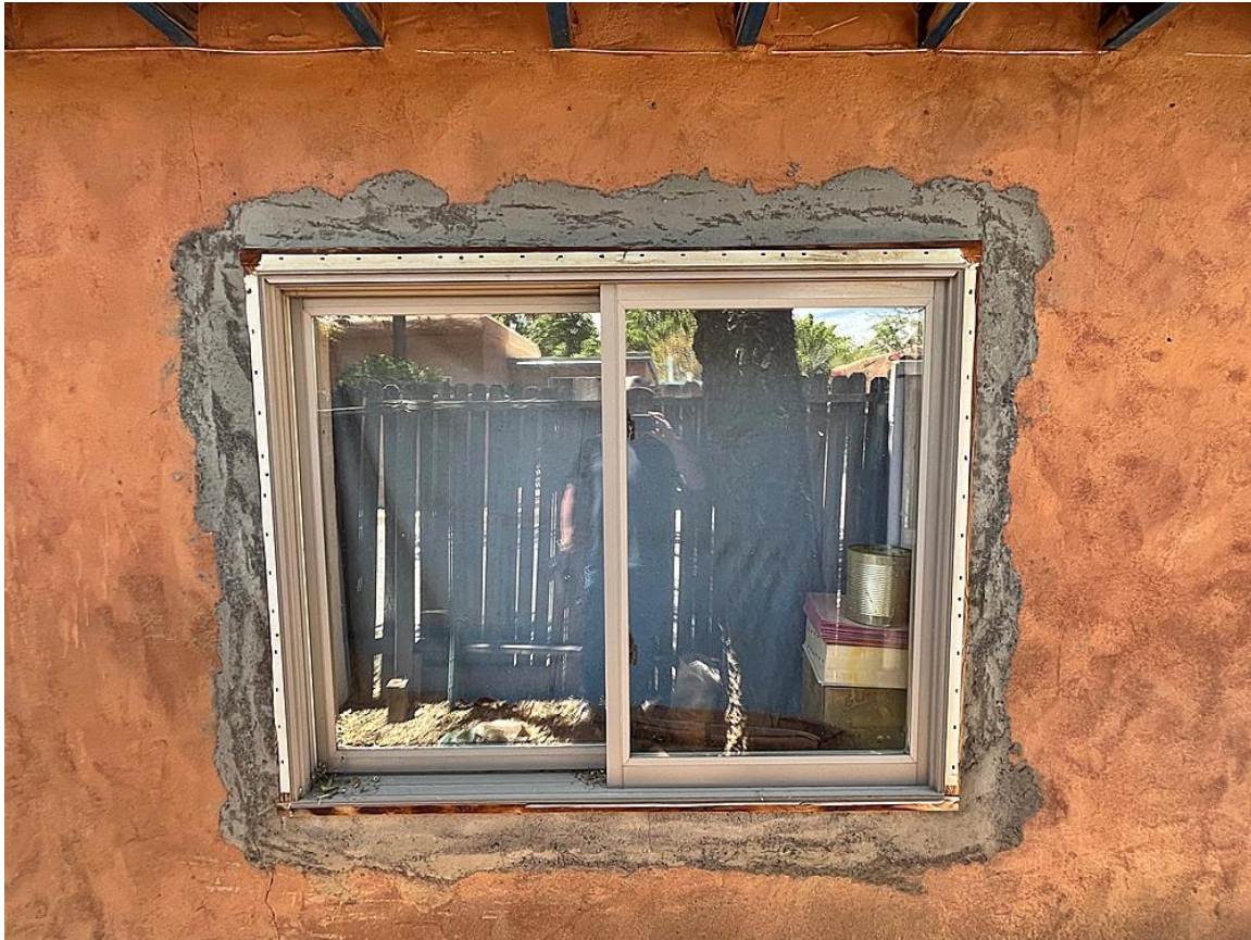
Photo 5: Building #1. East elevation. North window. Camera facing west.
