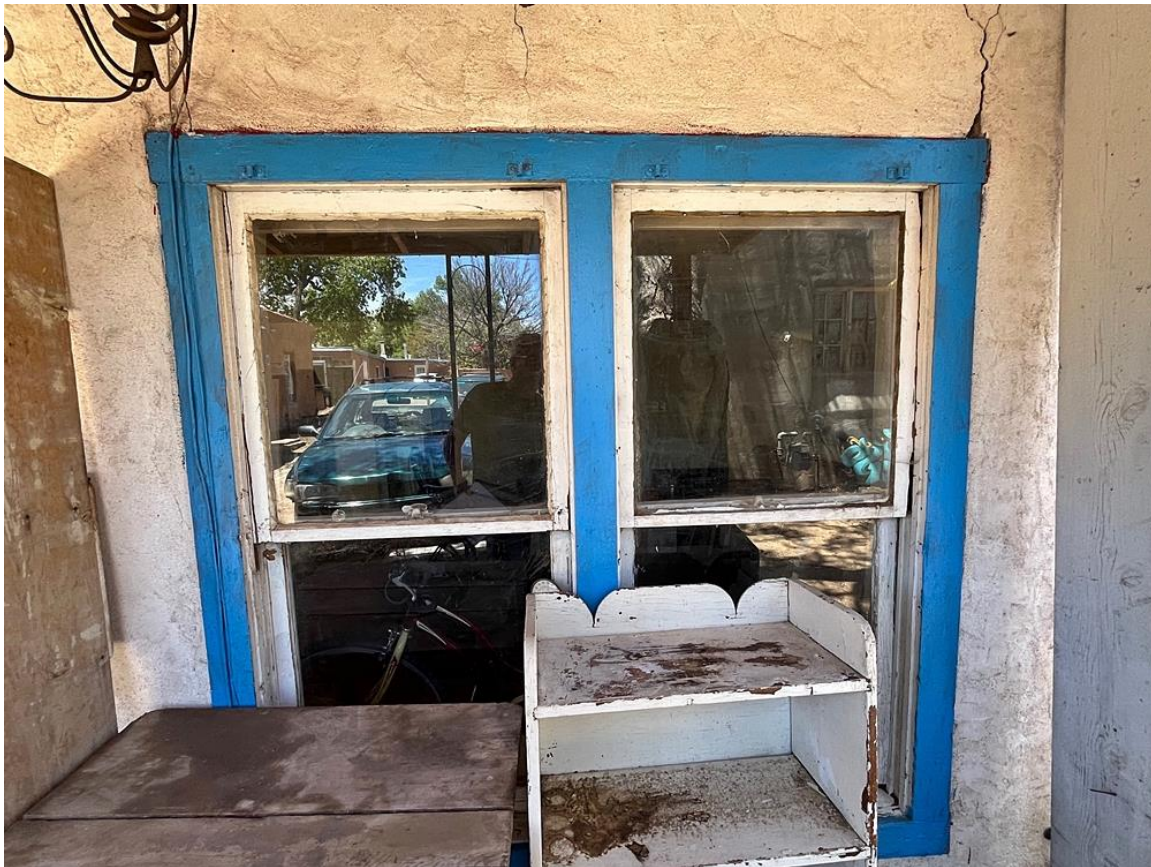
Photo 32: Building #3. East elevation. Window. Camera facing west.
