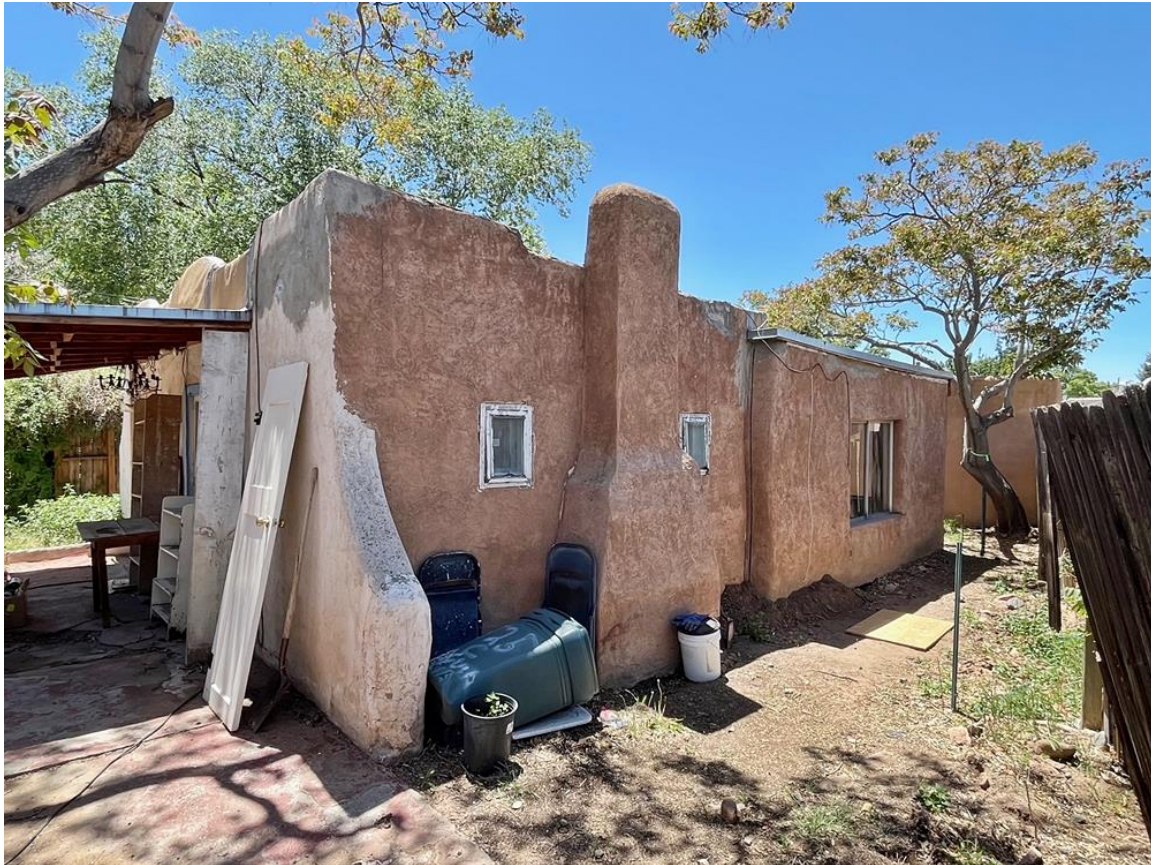
Photo 34: Building #3. North elevation. Camera facing southeast.
