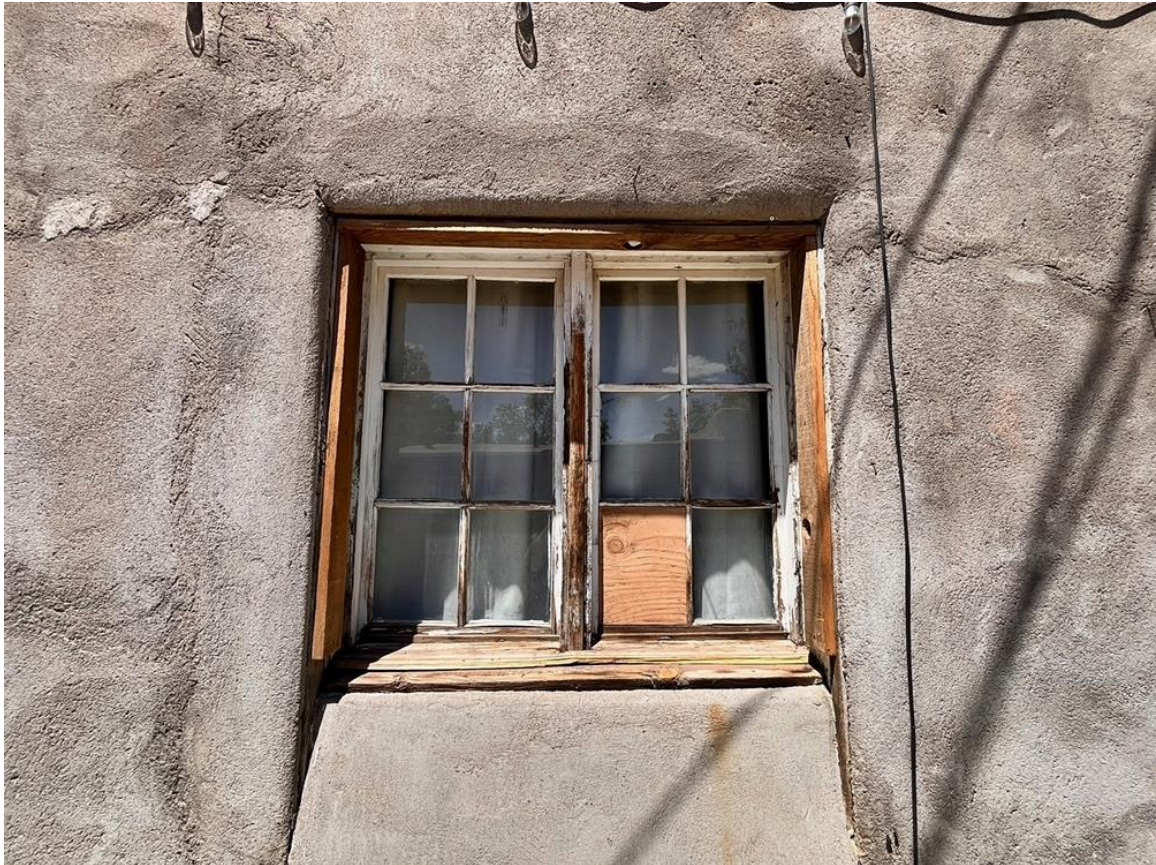
Photo 24: Building #2. South elevation. Window. Camera facing north.
