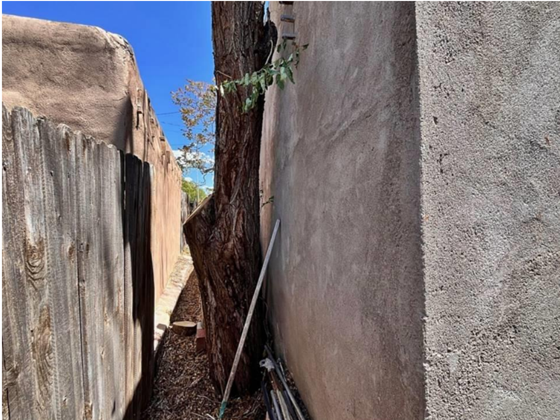
Photo 28: Building #2. North elevation. Camera facing east.
