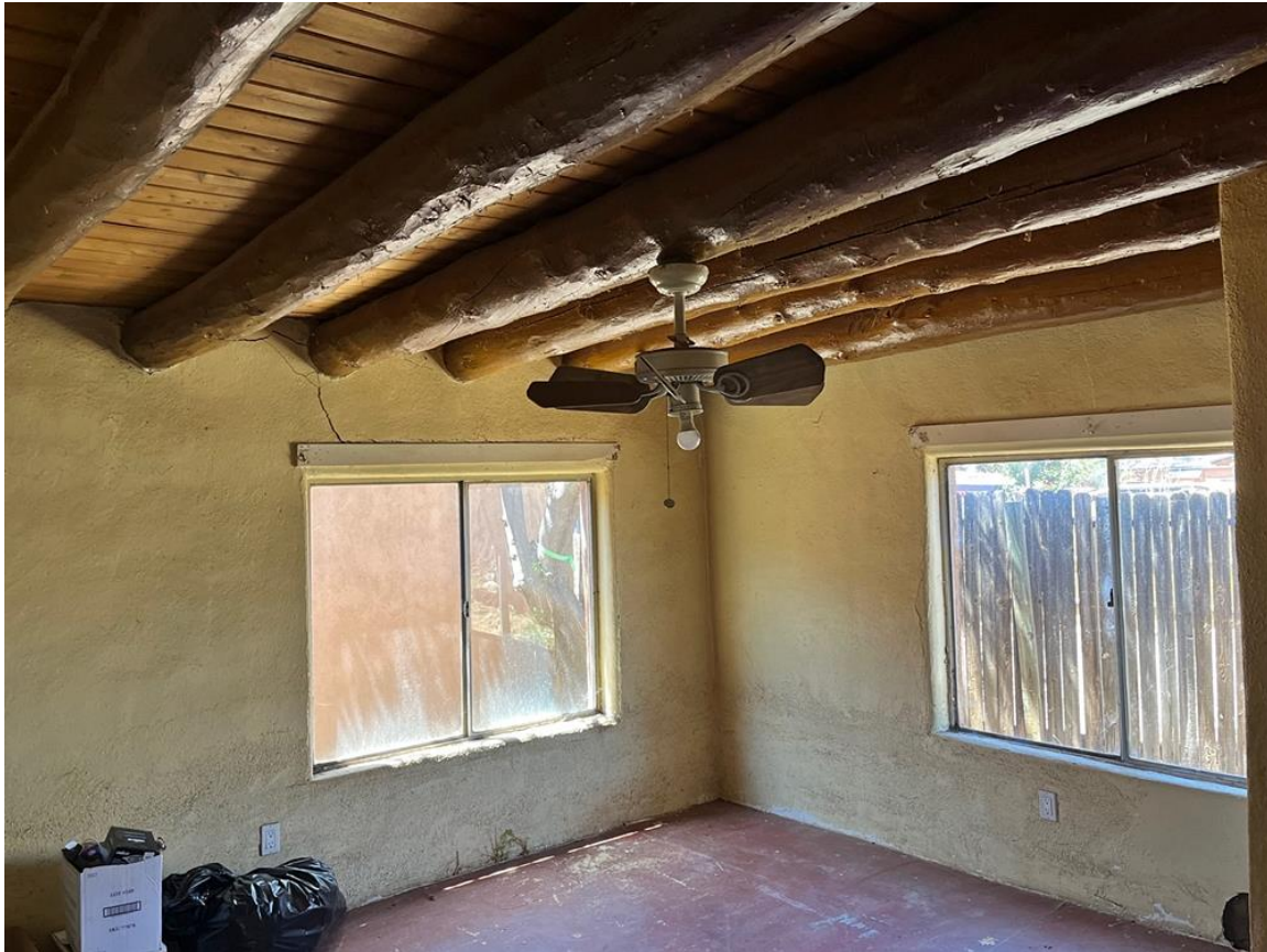
Photo 41: Building #3. Interior of bedroom. Camera facing northwest.
