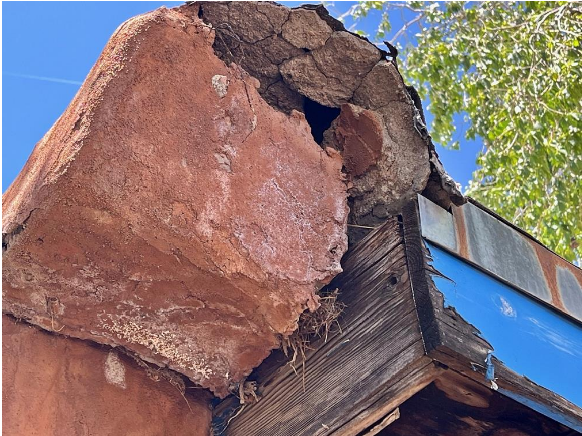
Photo 6: Building #1. False parapet. Camera facing up.
