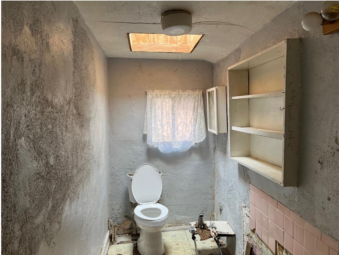
Photo 42: Building #3. Interior of bathroom. Camera facing west.
