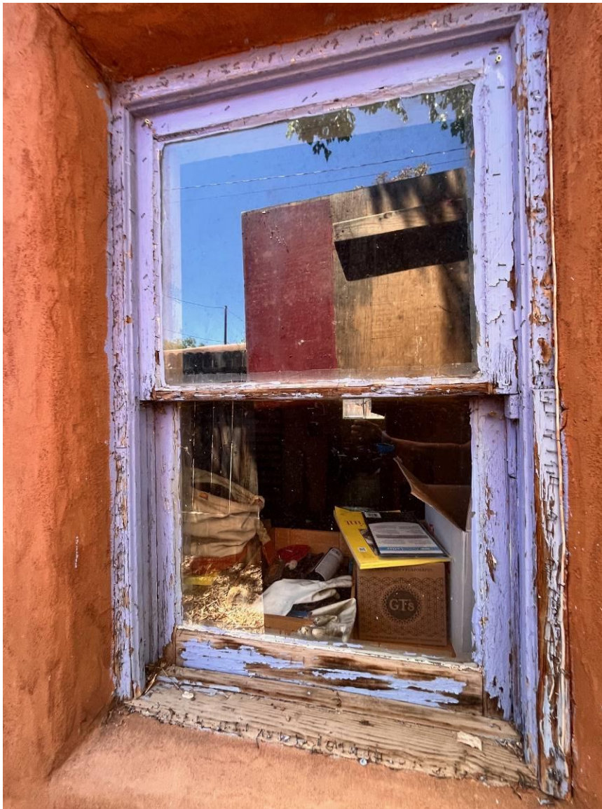
Photo 4: Building #1. East elevation. South window. Camera facing southeast.
