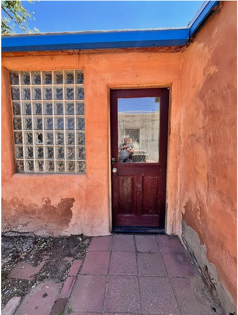
Photo 8: Building #1. North elevation. Enclosed porch. Camera facing south.
