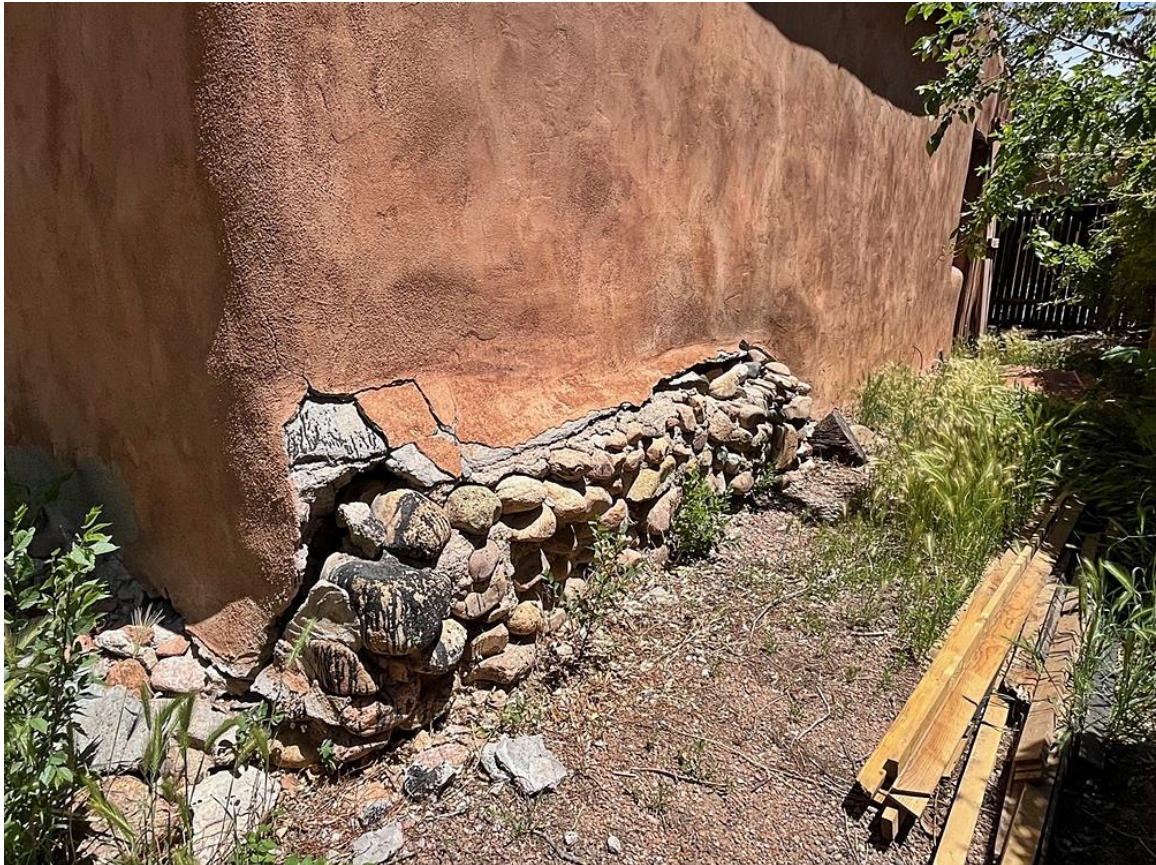
Photo 14: Building #1. South elevation. Camera facing northeast.
