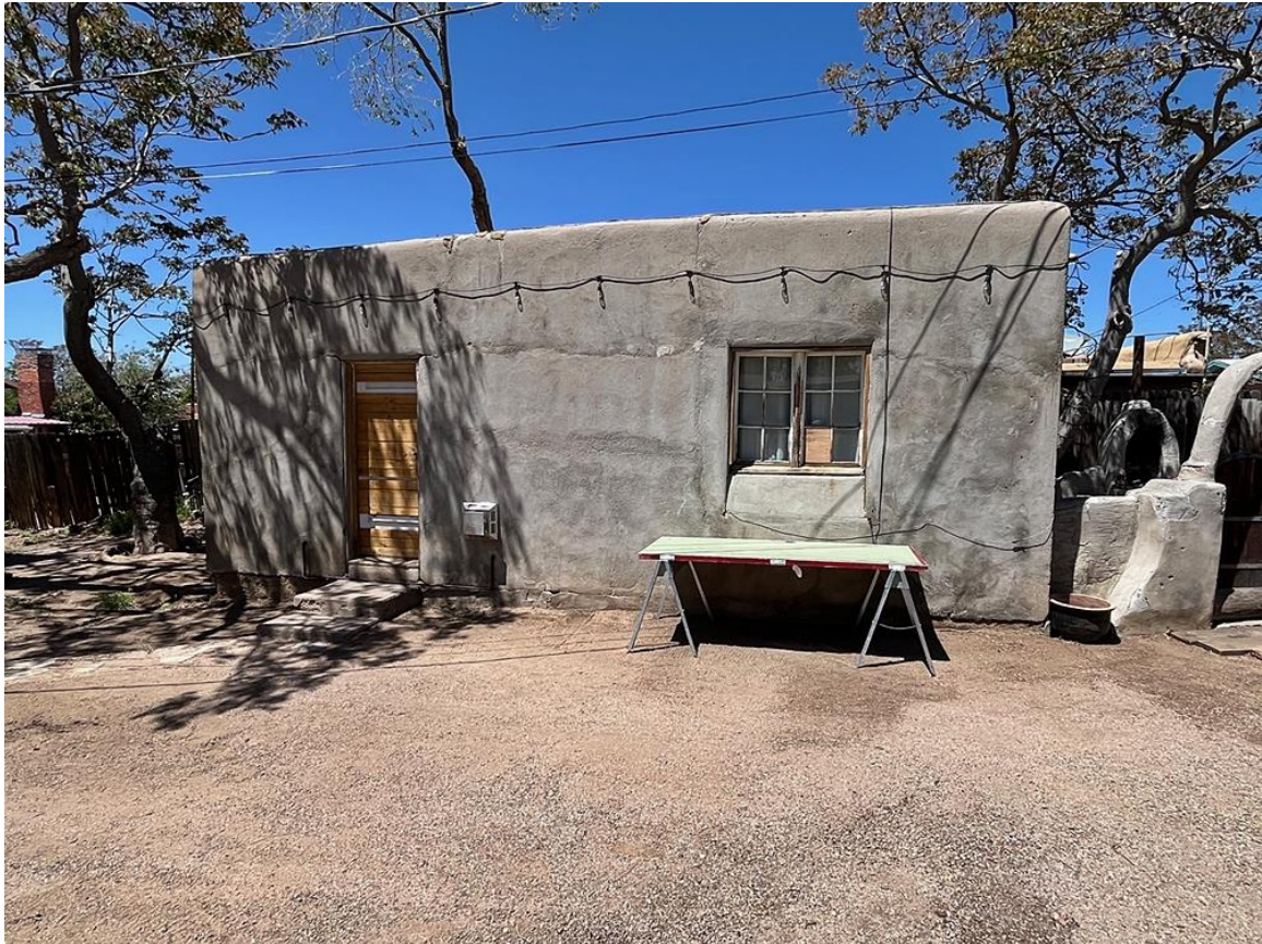
Photo 23: Building #2. South elevation. Camera facing north.
