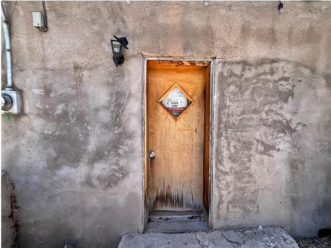
Photo 21: Building #2. East elevation. Camera facing west.
