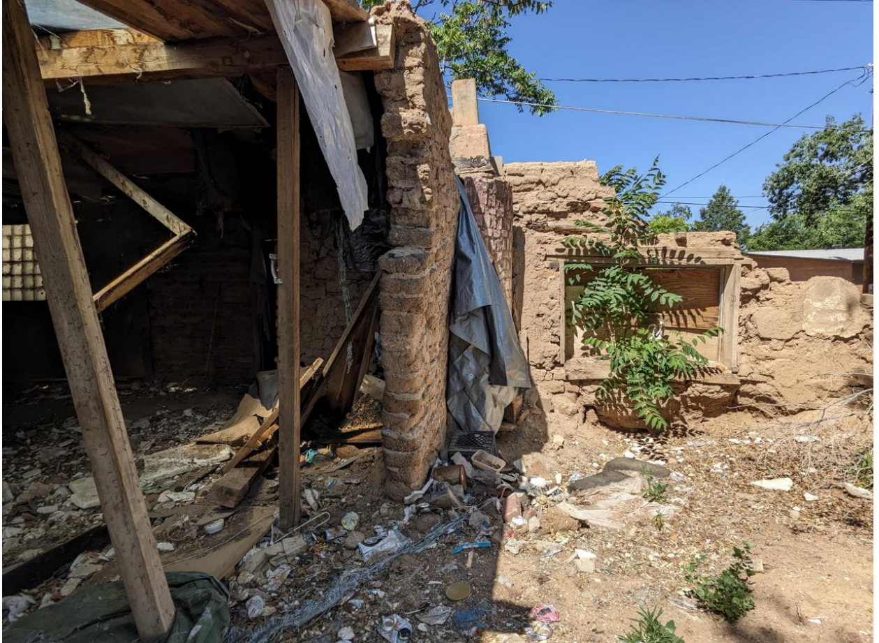
Figure 3: Interior of the Structure
