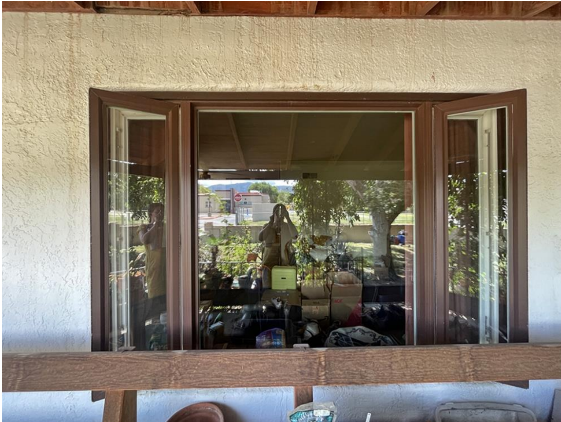
Photo 7: Porch. East elevation window. Camera facing west.
