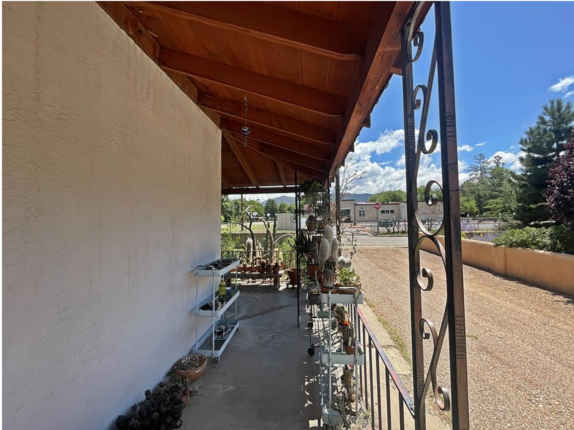
Photo 5: Porch on south elevation. Camera facing east.
