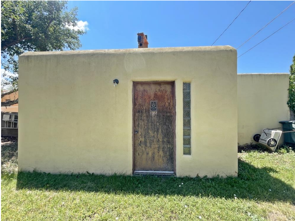
Photo 18: Workshop. North elevation. Camera facing south.
