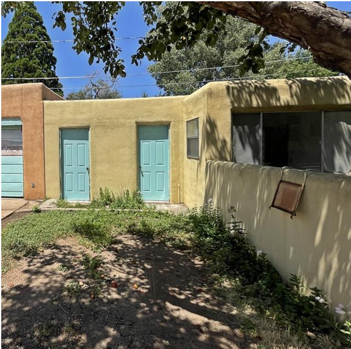
Photo 16: Former garage. Camera facing west.
