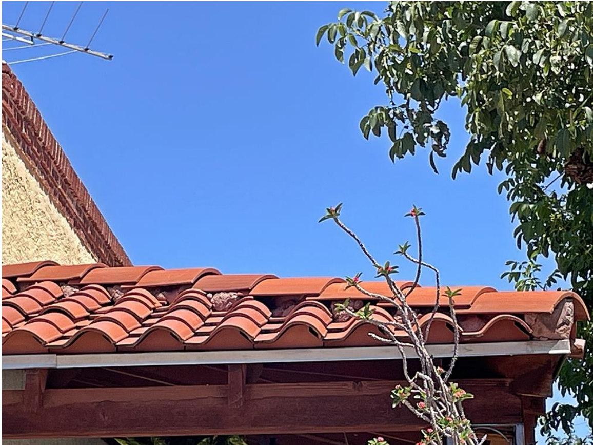
Photo 6: Porch roofing material. Camera facing up.
