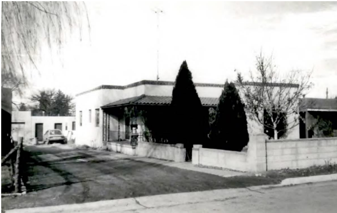
Figure 7: December 2, 1985, HBI survey photograph. Michael Belshaw. Note absence of the two greenhouse window boxes along the south elevation.
