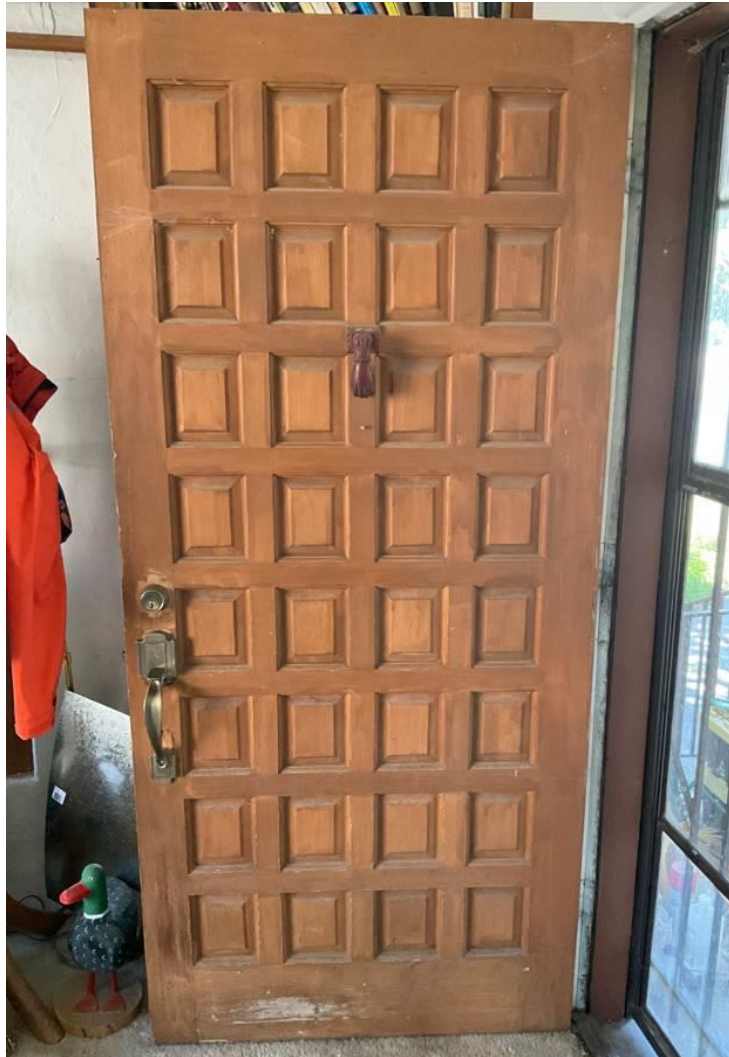
Photo 8: Porch. East elevation entry door to apartment. David Kozlowski, August 5, 2025.
