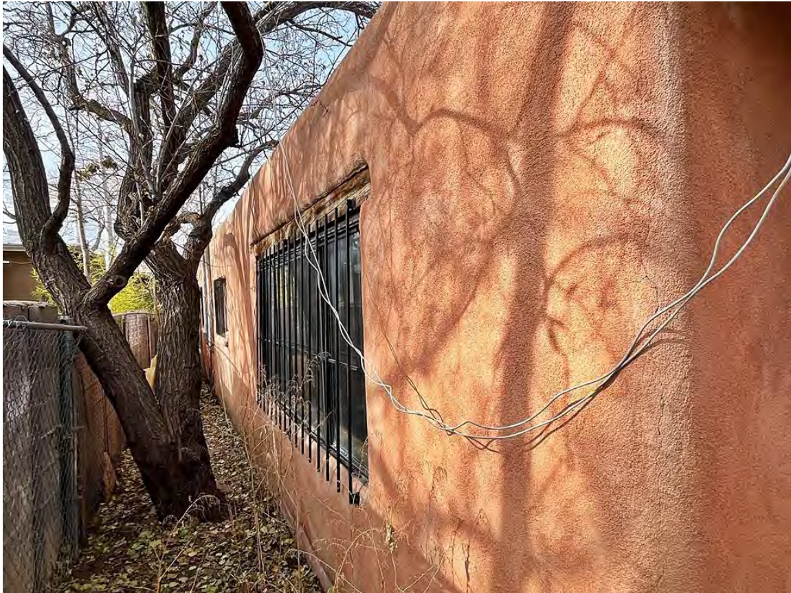
Photo 11: South elevation. Camera facing northwest.
