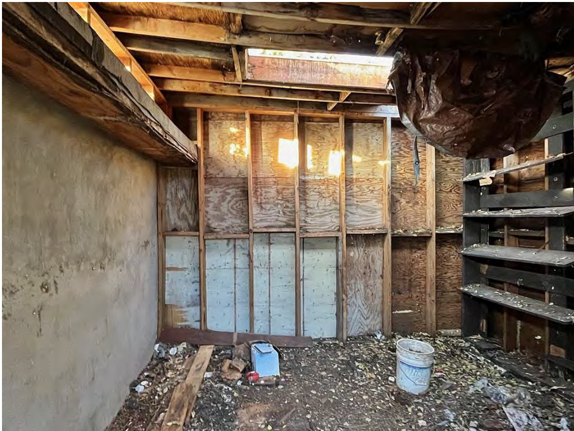
Photo 26: Photo 25: Shop. Addition, interior. Camera facing north.
