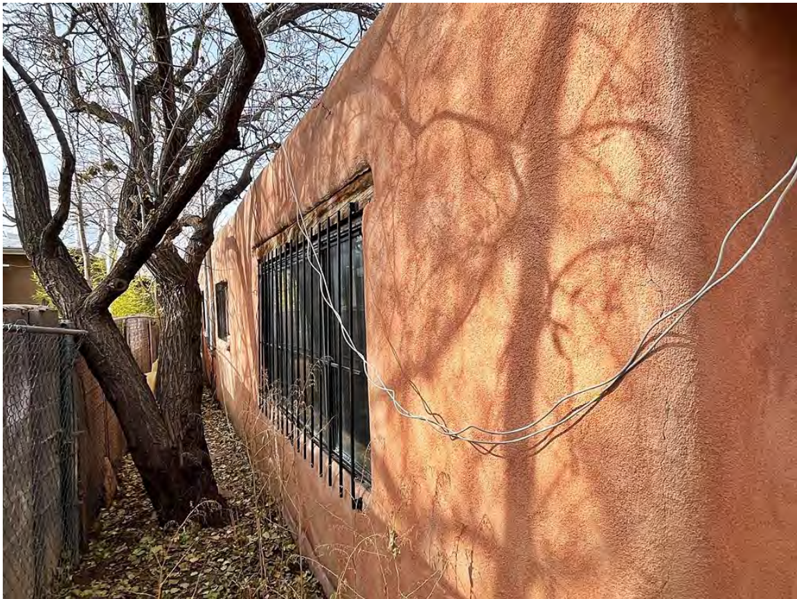
Photo 11: South elevation. Camera facing northwest.
