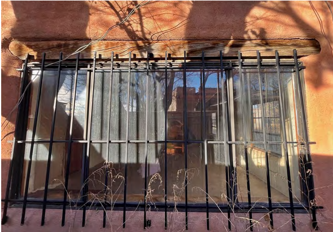
Photo 12: South elevation at 1980s addition. Window at living room. Camera facing north.
