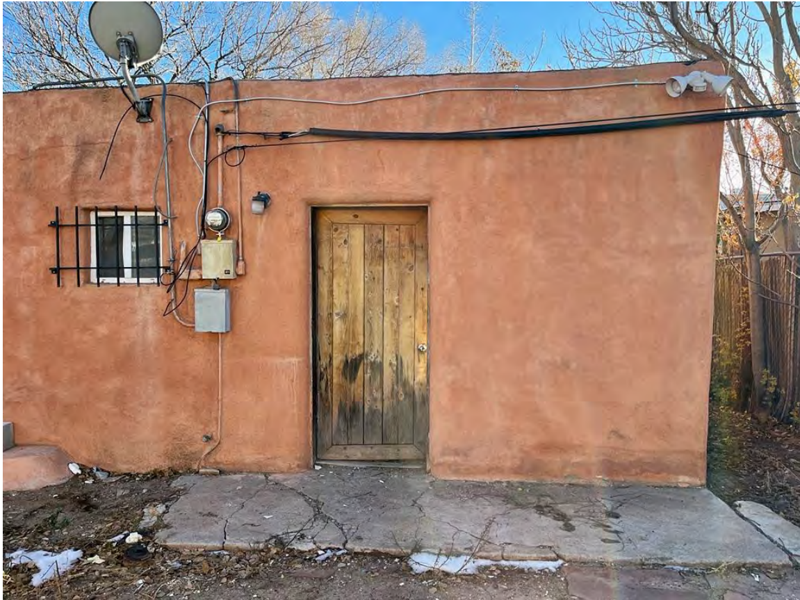
Photo 6: North elevation representing the northwest room of the original core. Camera facing south.
