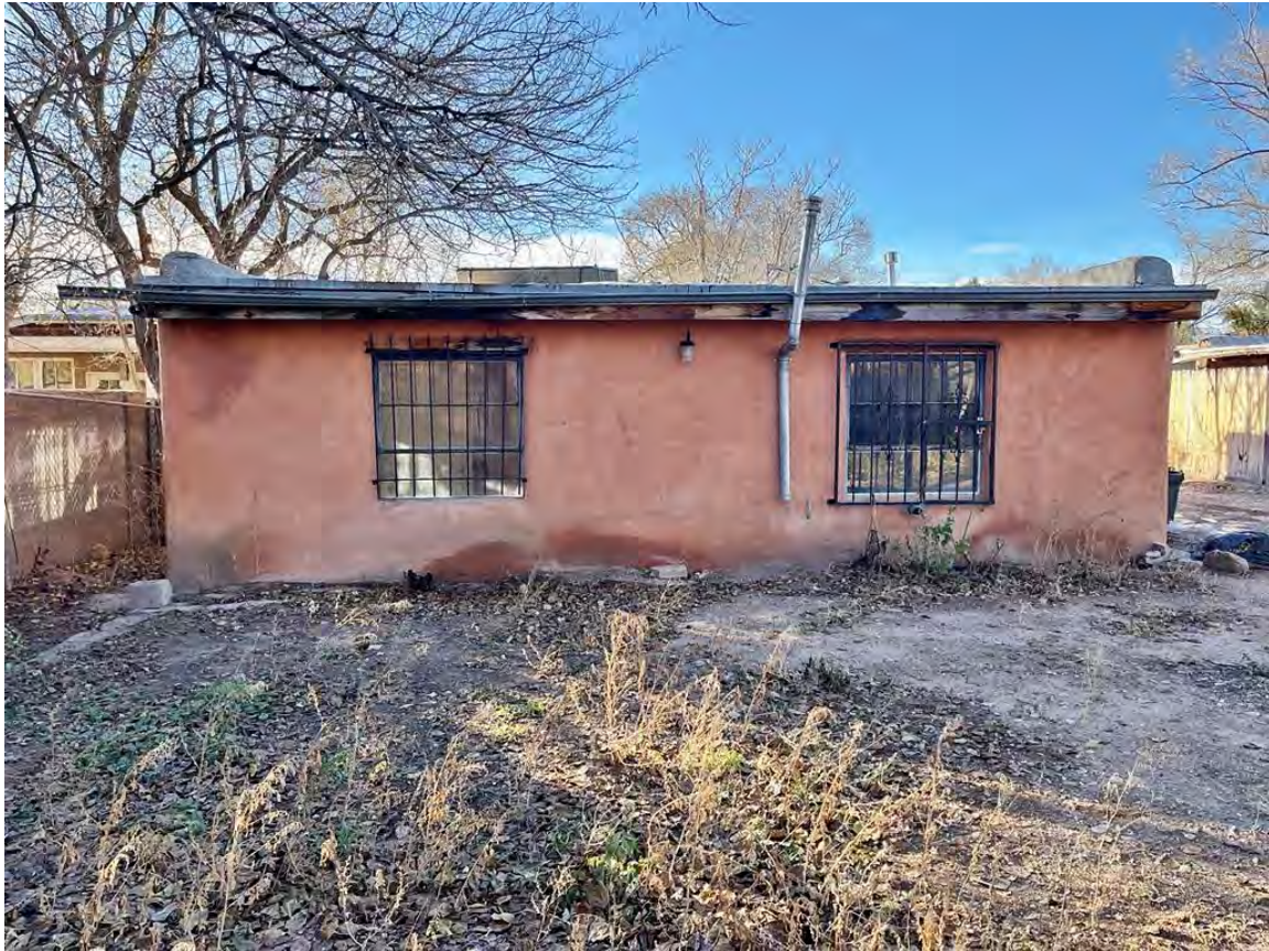
Photo 9: East elevation representing 1980s addition. Camera facing west.
