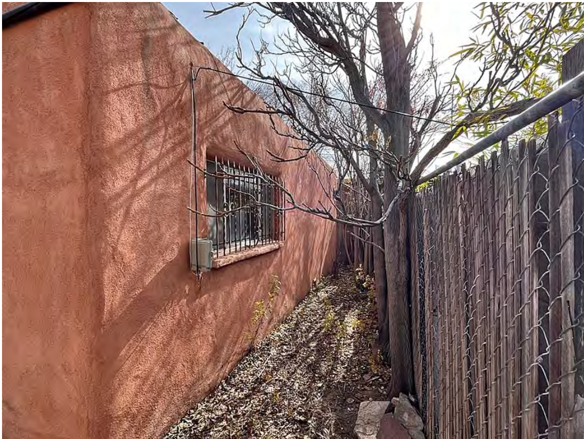
Photo 16: West elevation. Camera facing southeast.
