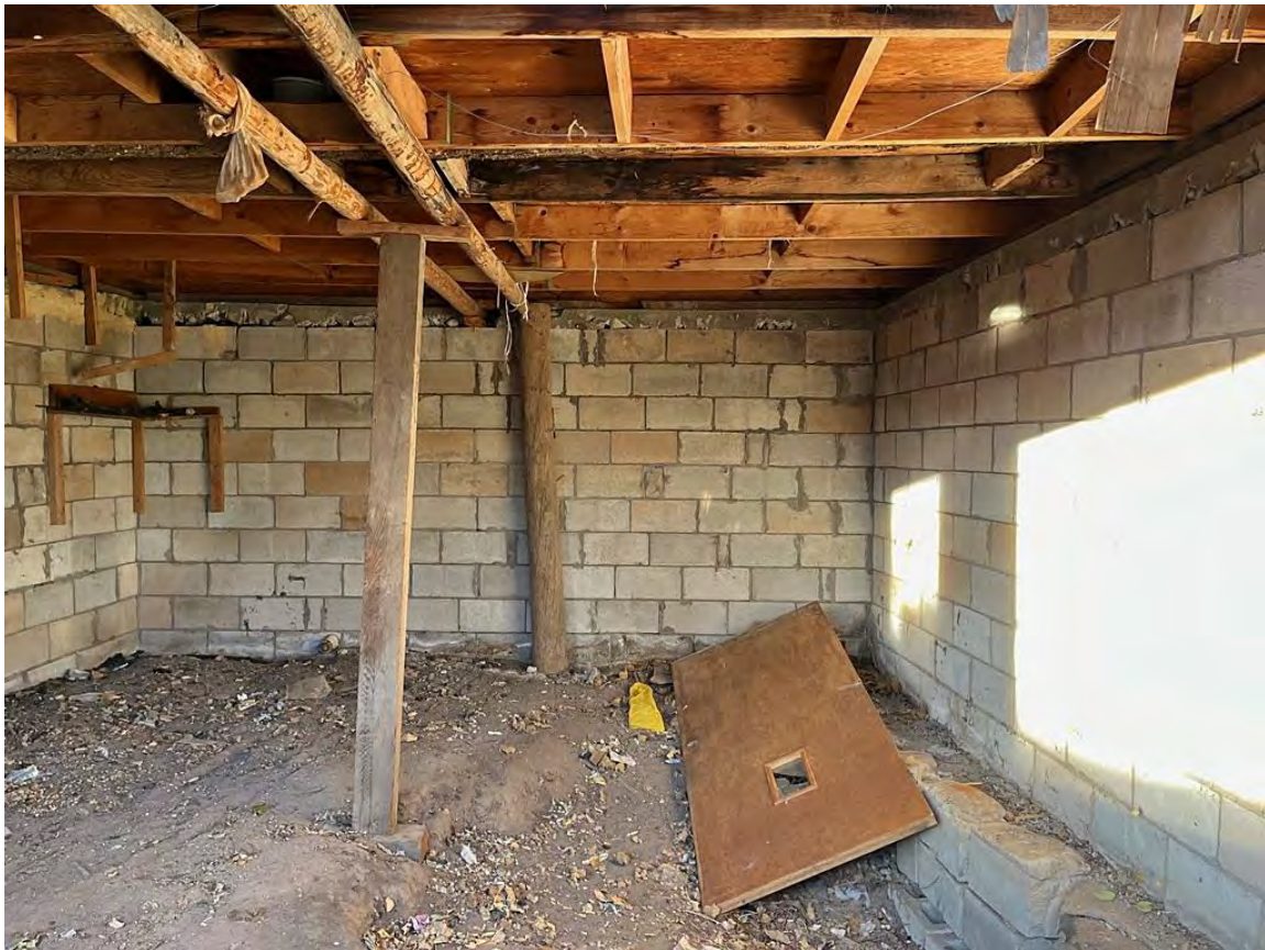
Photo 24: Shop. Interior. Camera facing north.
