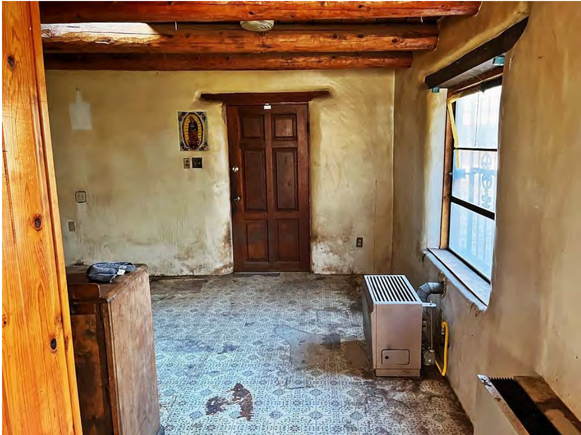
Photo 22: 1980s addition. Camera facing north.
