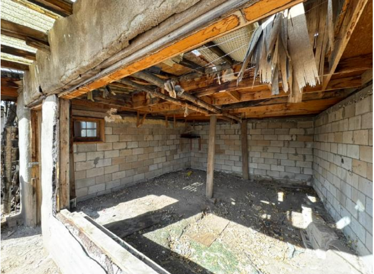
Figure 3: Interior of the Accessory Structure
