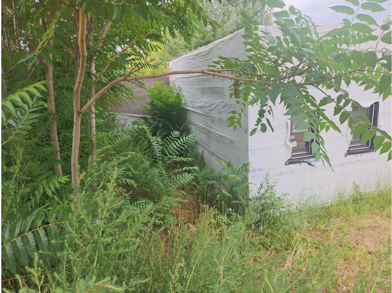
The subject studio behind the trees, not visible from the street due to elevation changes, 1301 adobe-esque wall, and foliage.
