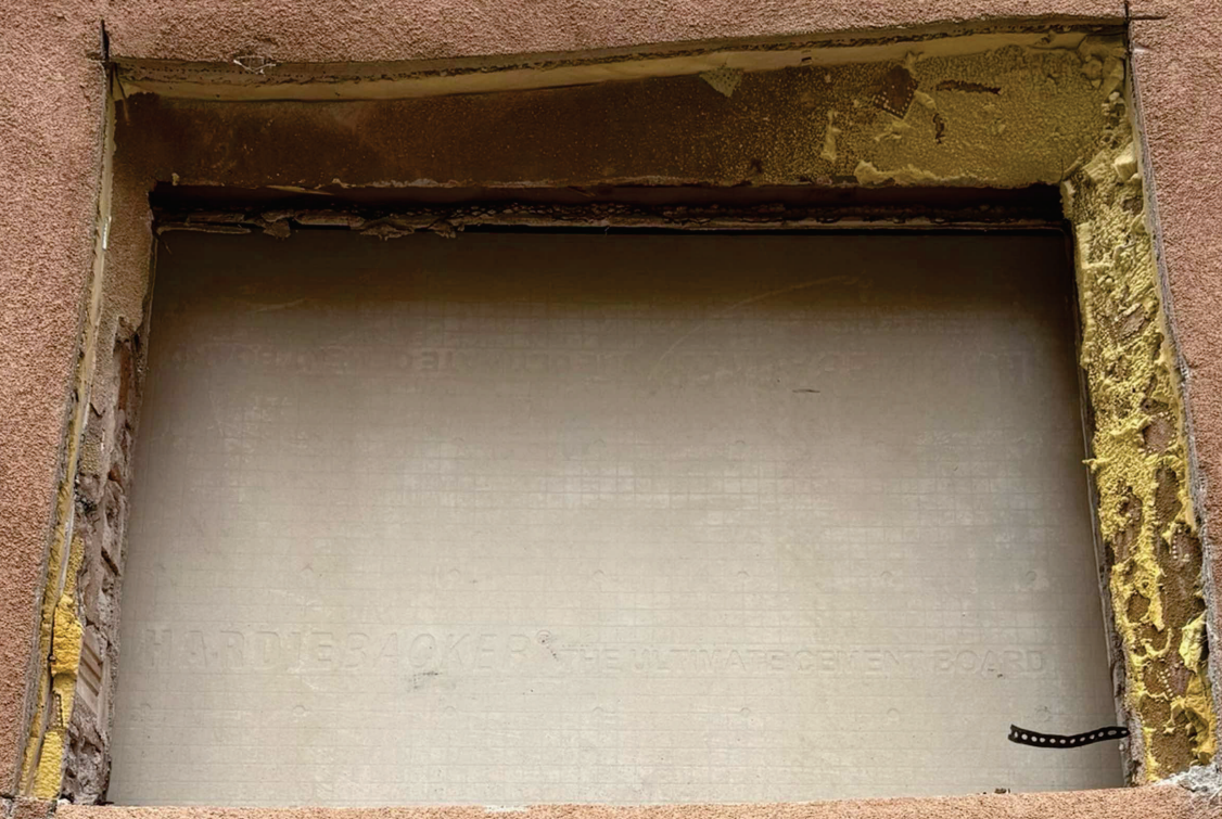
South Elevation Window #3
