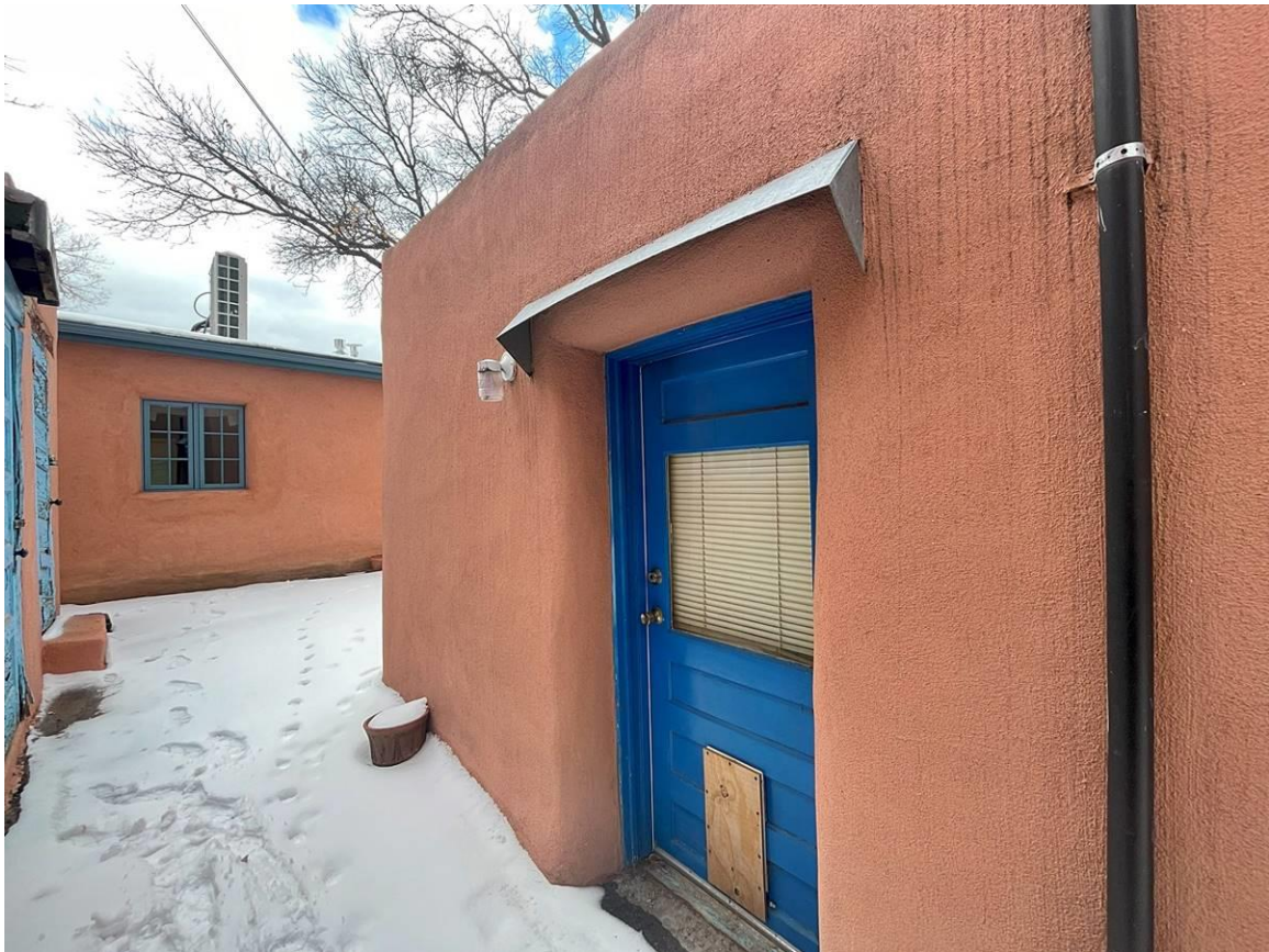
Photo 8: North elevation, entry. Camera facing southeast.
