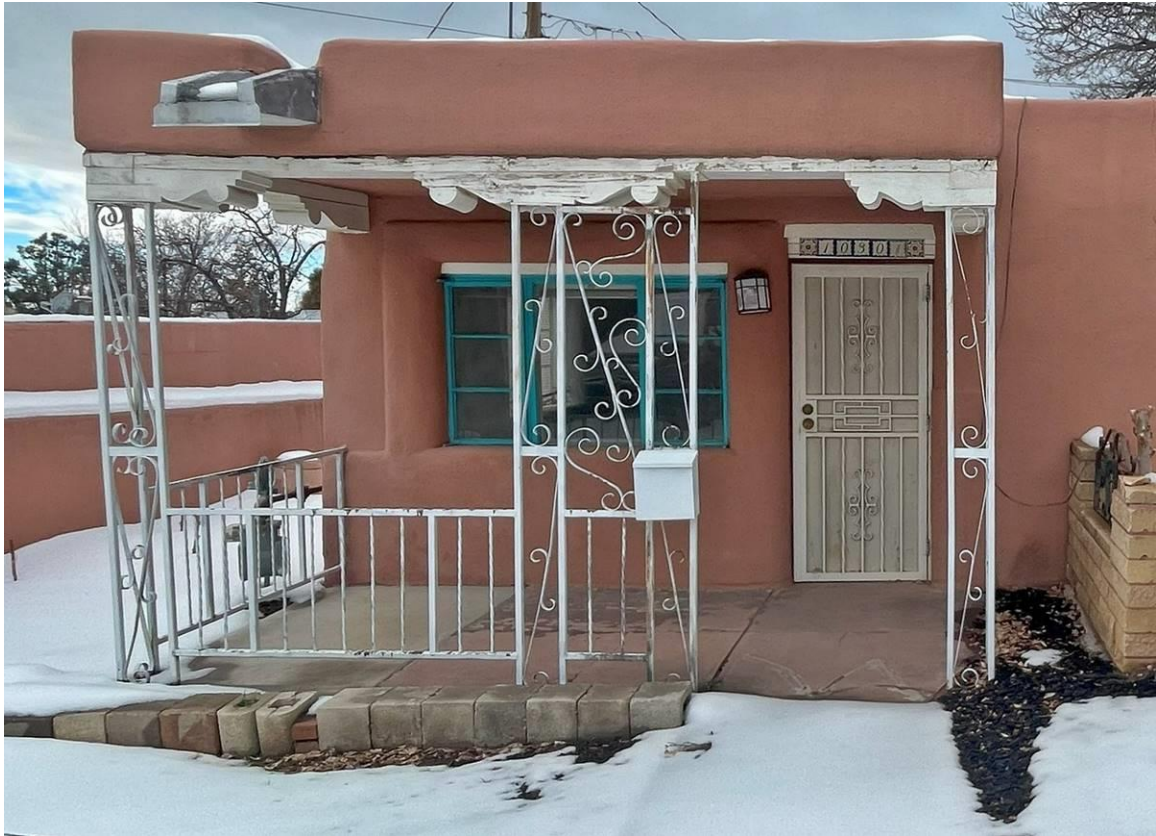
Photo 4: East elevation, porch. Camera facing west.
