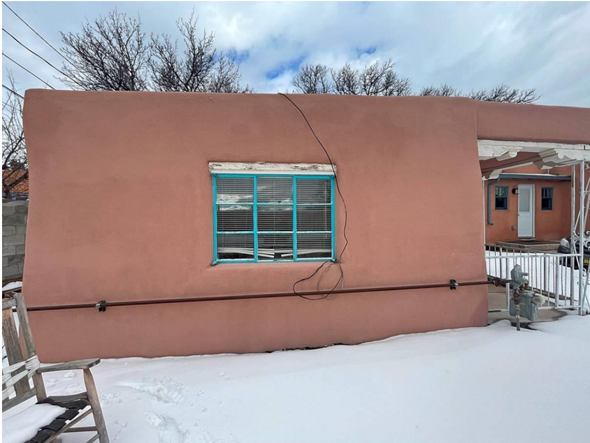
Photo 10: South elevation. Camera facing north.
