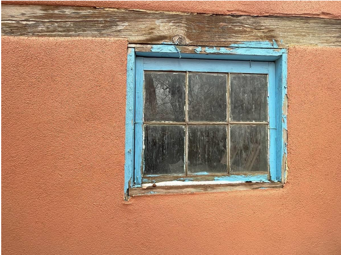
Photo 14: East elevation. Camera facing northwest.
