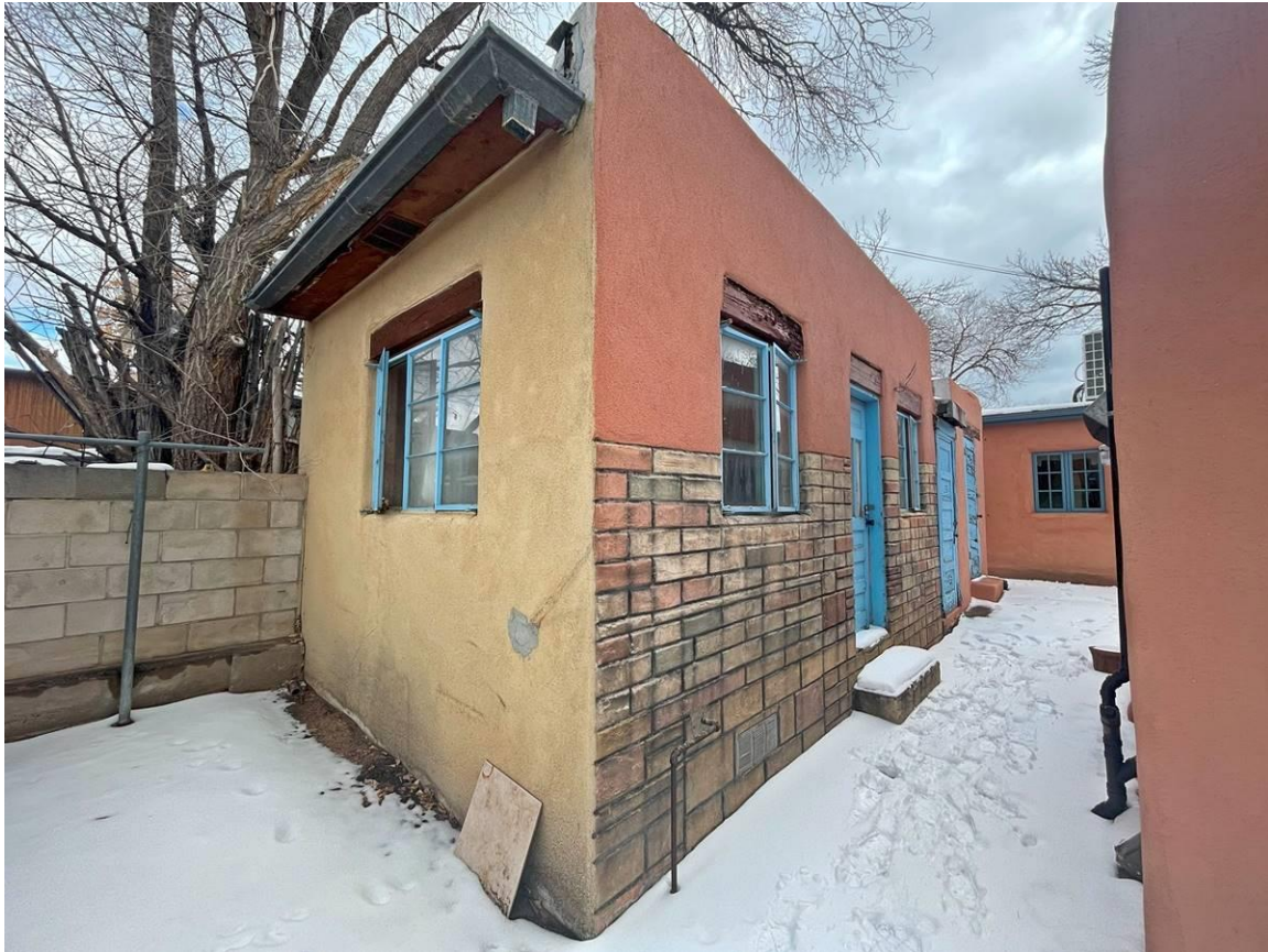
Photo 13: West and south elevations. Camera facing northeast.
