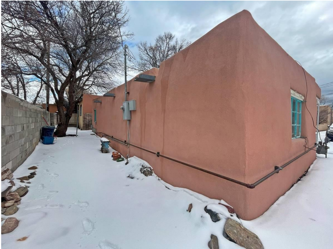
Photo 11: West and south elevations. Camera facing northeast.
