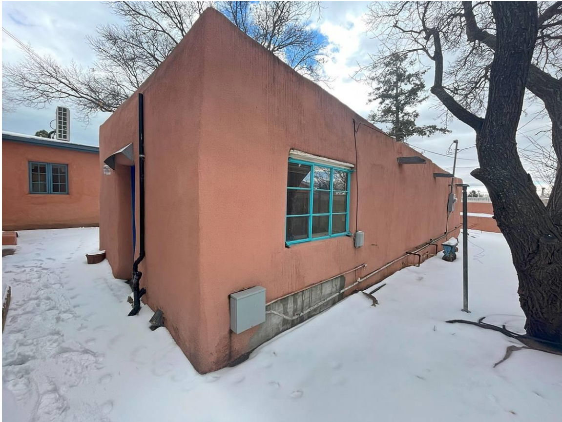
Photo 9: North and west elevations. Camera facing southeast.
