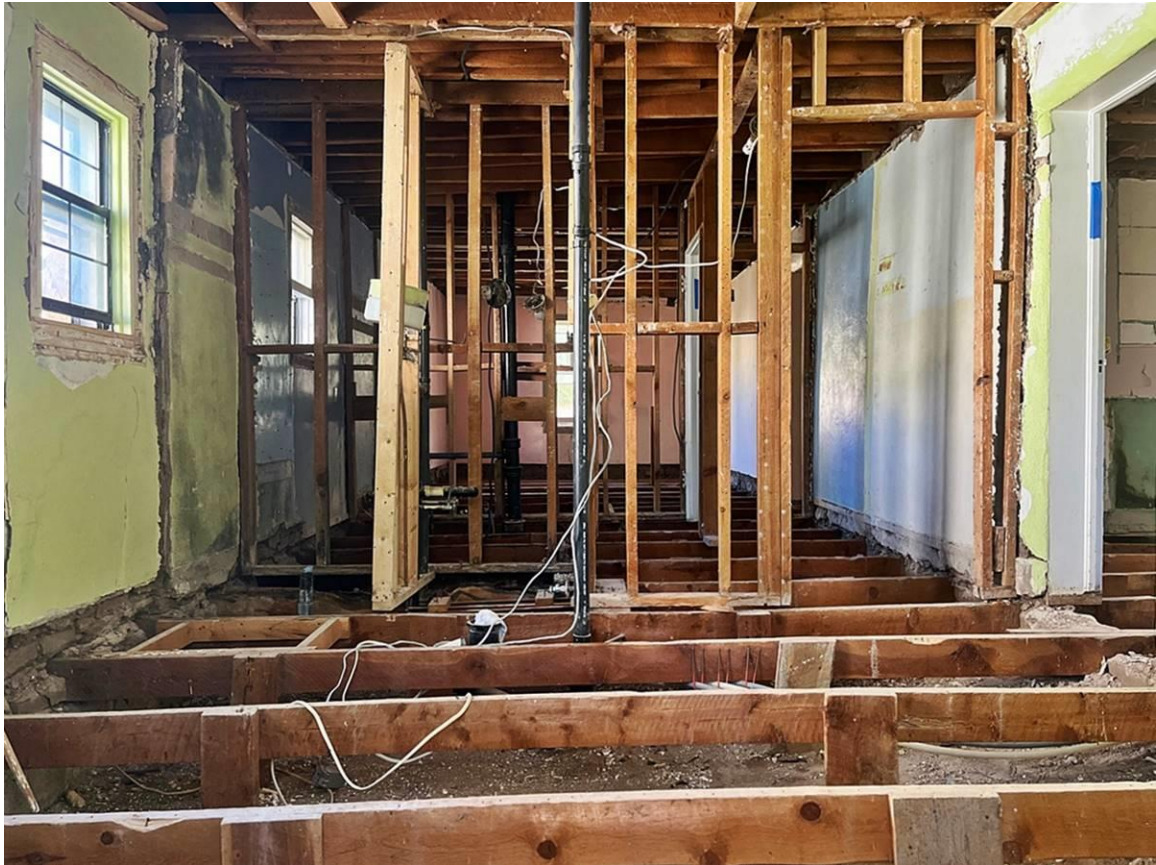
Photo 15: Bedroom Wing interior. Camera facing east.
