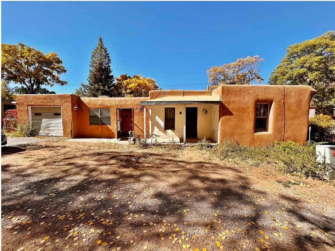
Photo 2: Full east façade. Camera facing southwest.
