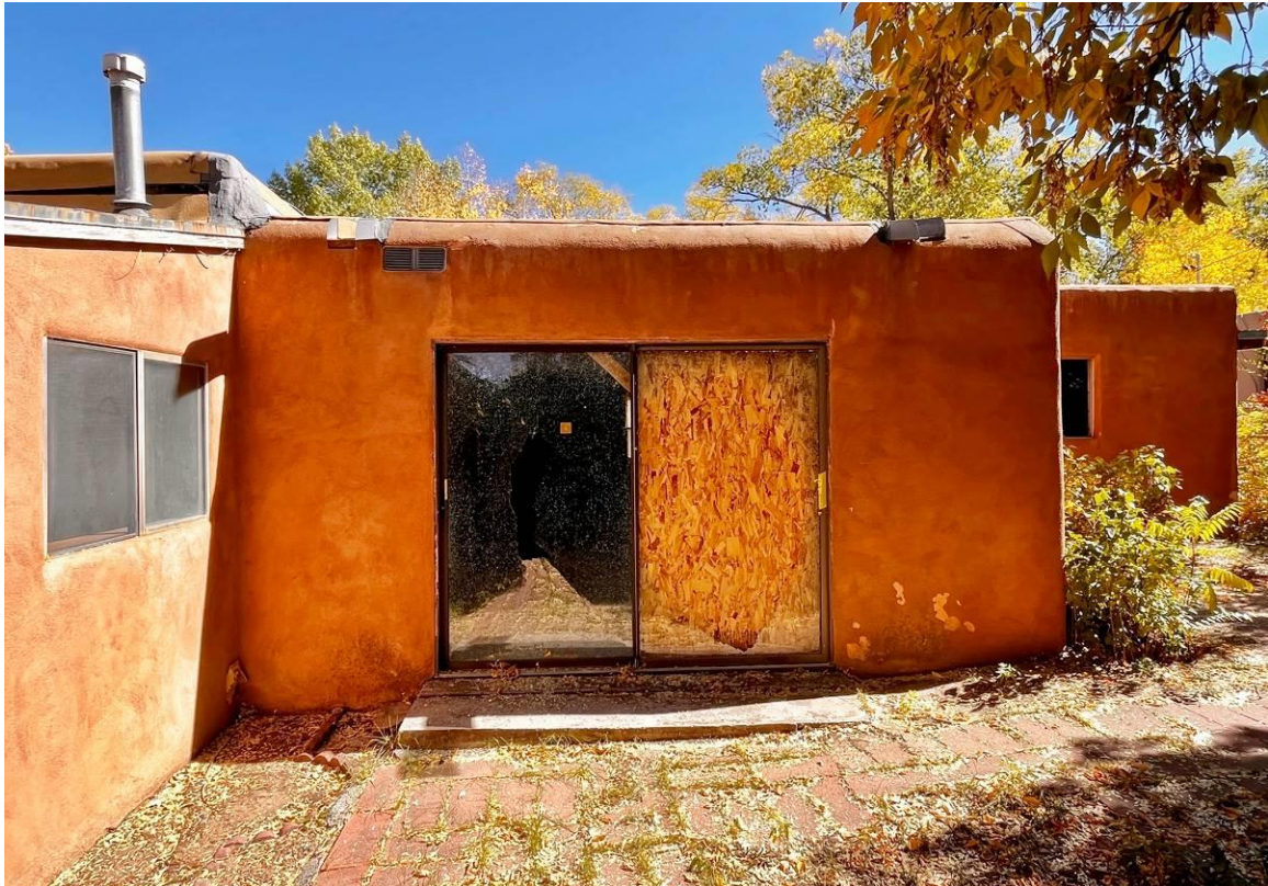
Photo 19: West elevation, Family Room (c.1976). Camera facing east.
