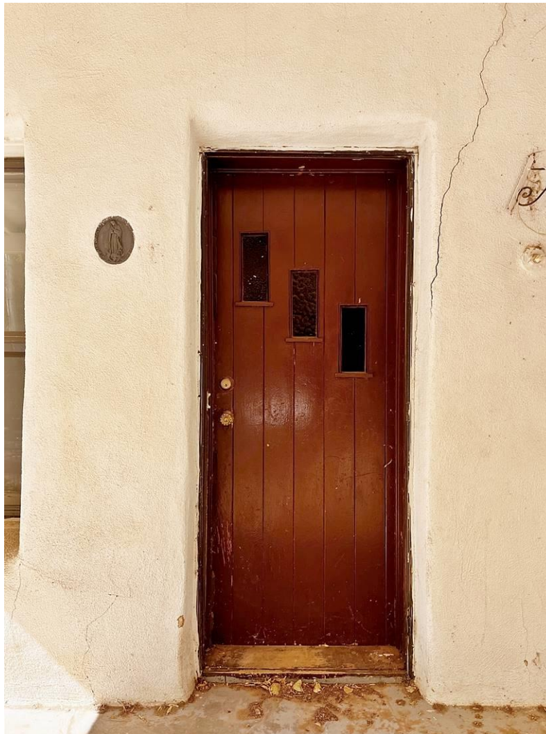
Photo 8: East façade, entry. Camera facing west.
