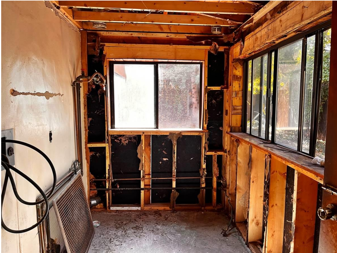
Photo 18: Laundry Room interior. Camera facing south.
