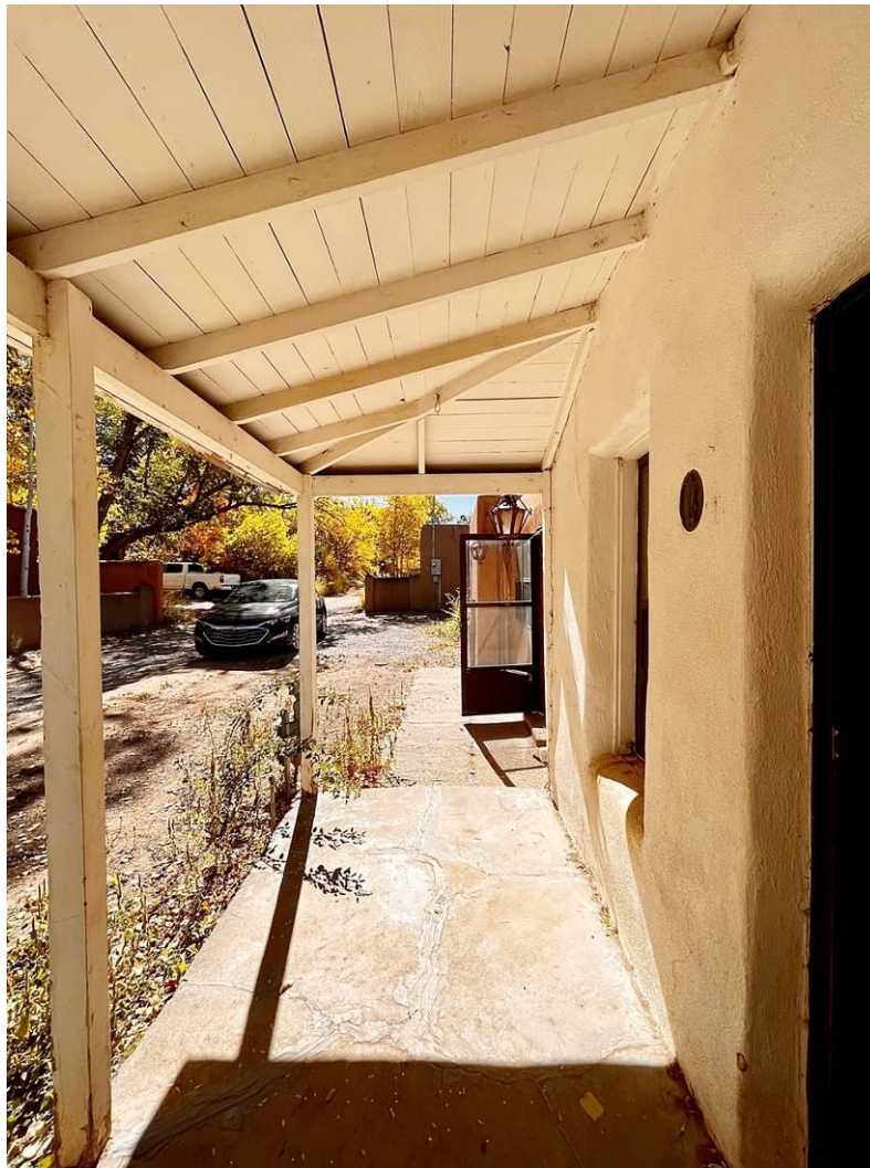
Photo 7: Porch, decking. Camera facing south.
