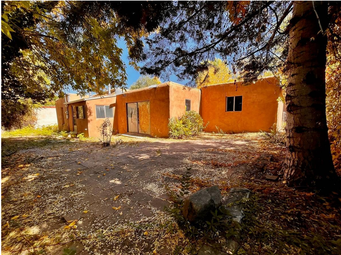
Photo 16: Full west elevation. Camera facing northeast.
