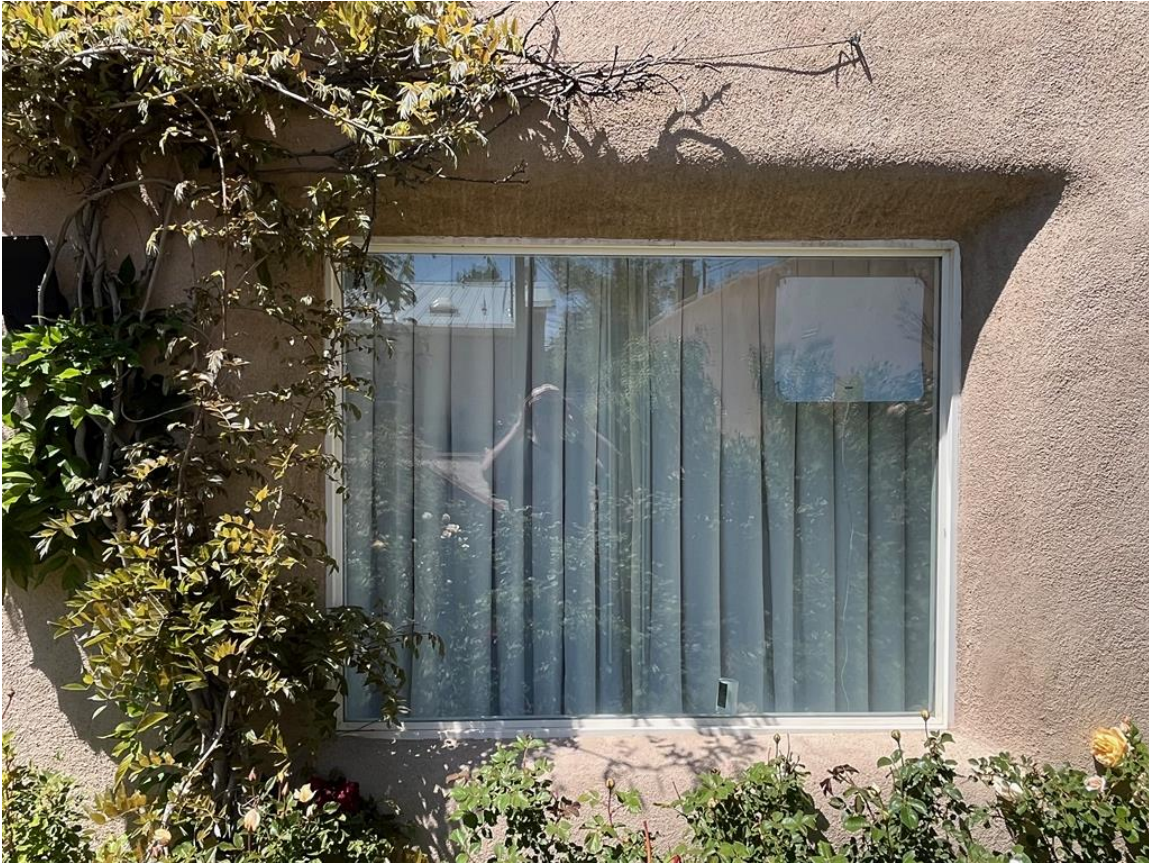
Photo 5: South elevation. Window set in original garage door opening. Camera facing north.
