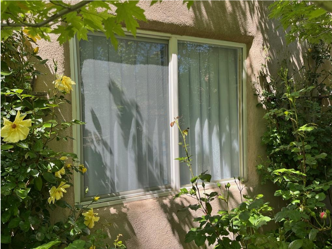
Photo 6: South elevation. Window in 1960s addition. Camera facing northeast.
