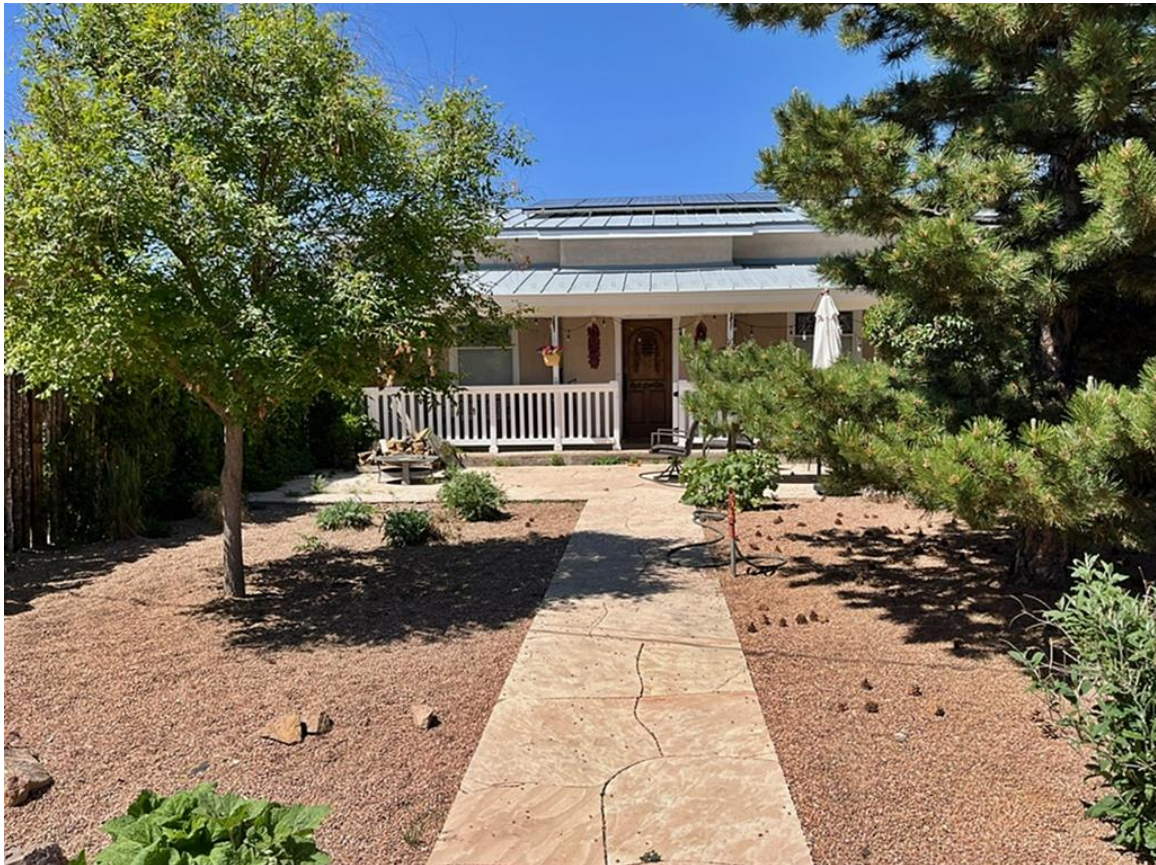
Photo 3: Hilario Ortiz House. Camera facing north.
