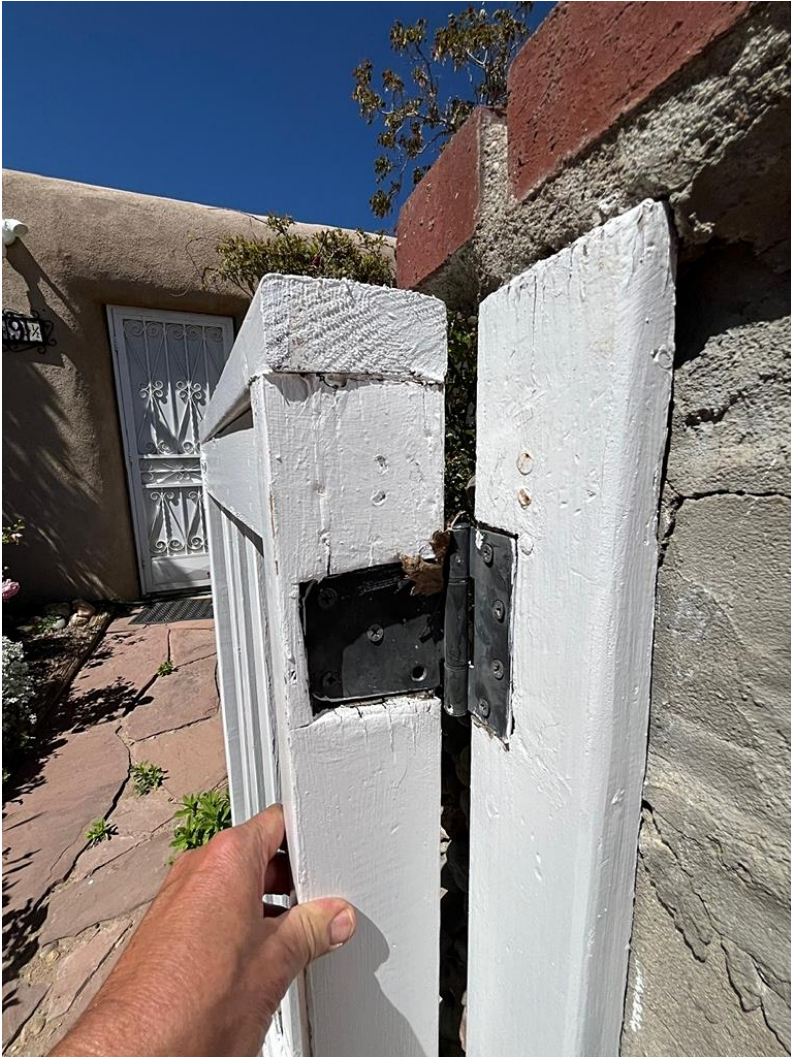
Photo 15: Gate. Detail of construction. Camera facing north.
