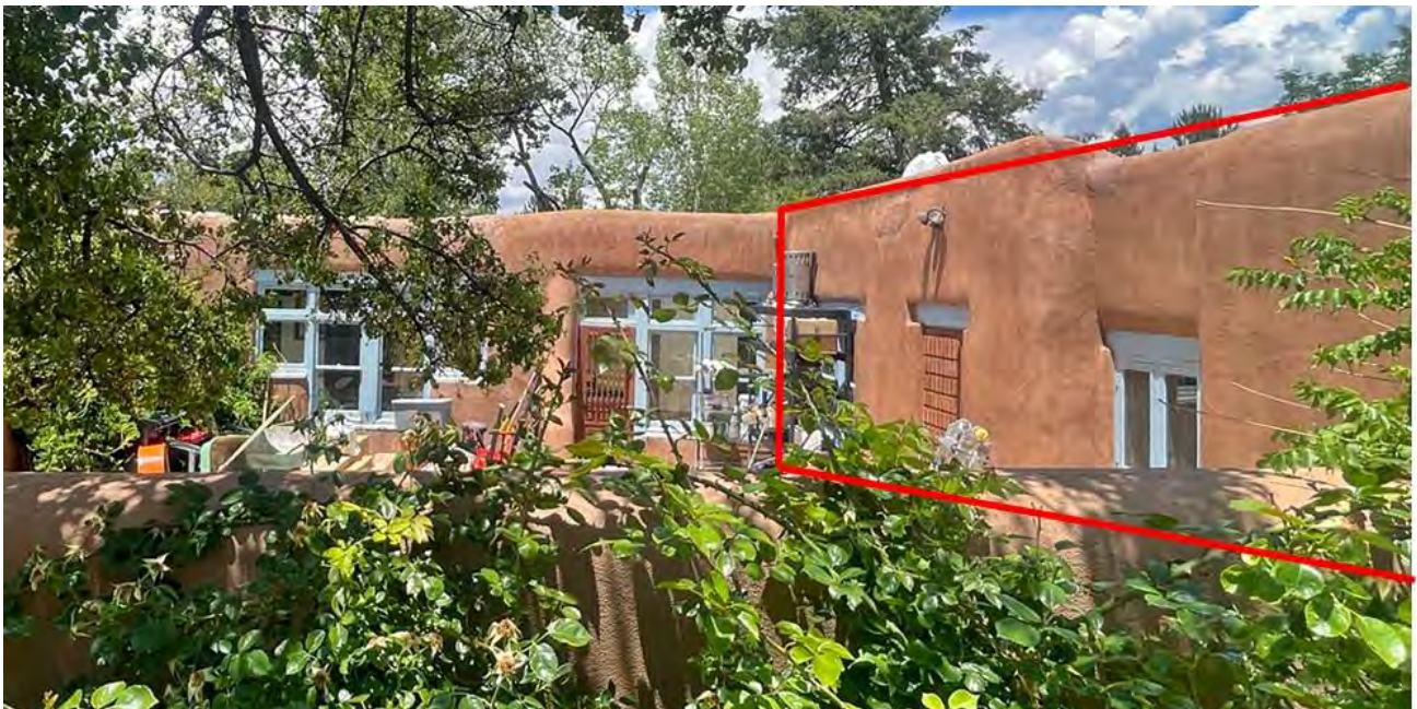
Figure 21: Courtyard. Red indicates post-Austin/Meem additions.
