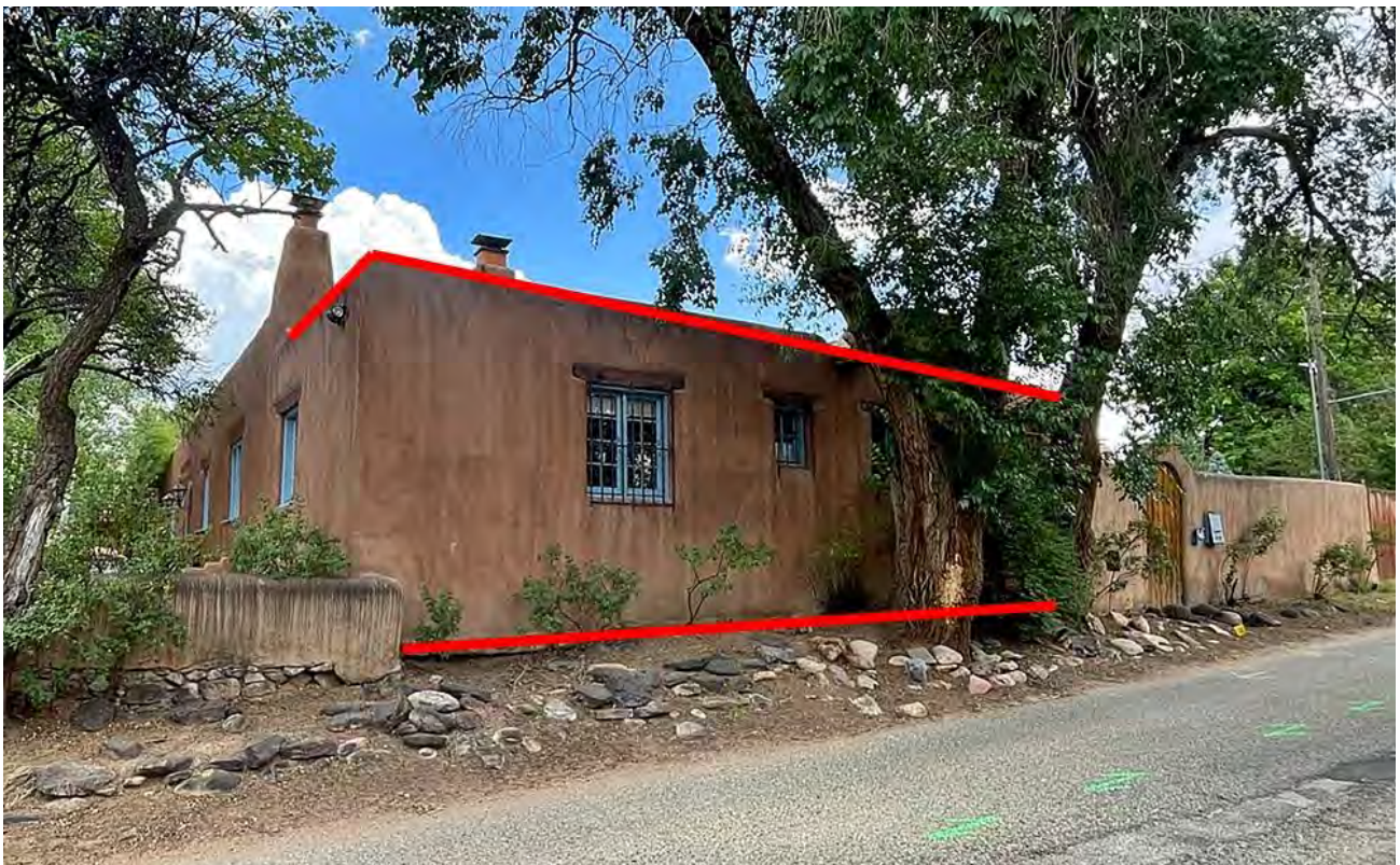
Figure 19: West elevation. Red indicates post-Austin/Meem additions.
