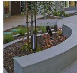
CURVILINEAR CONCRETE WALLS
