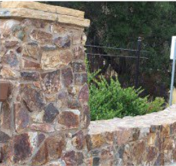
MORTARED ROCK WALL
