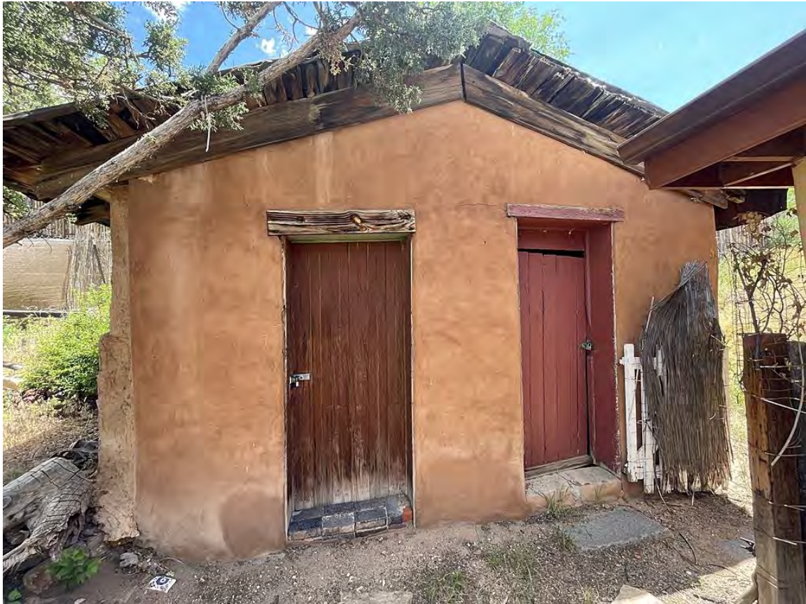
Photo 16: Shed. South elevation. Camera facing northeast.
