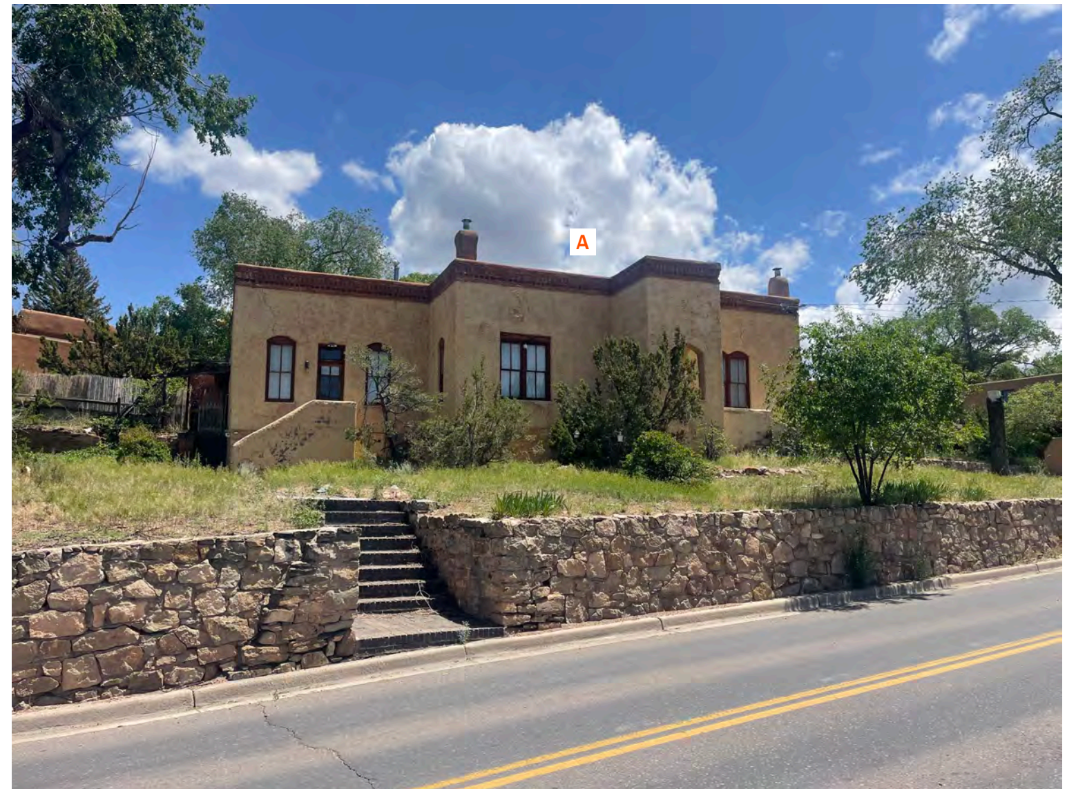
SITE FROM SOUTHWEST
