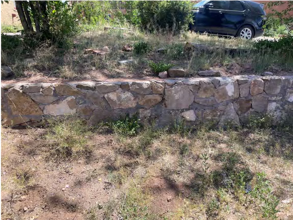
Photo 21: Minor retaining wall. Camera facing southeast.
