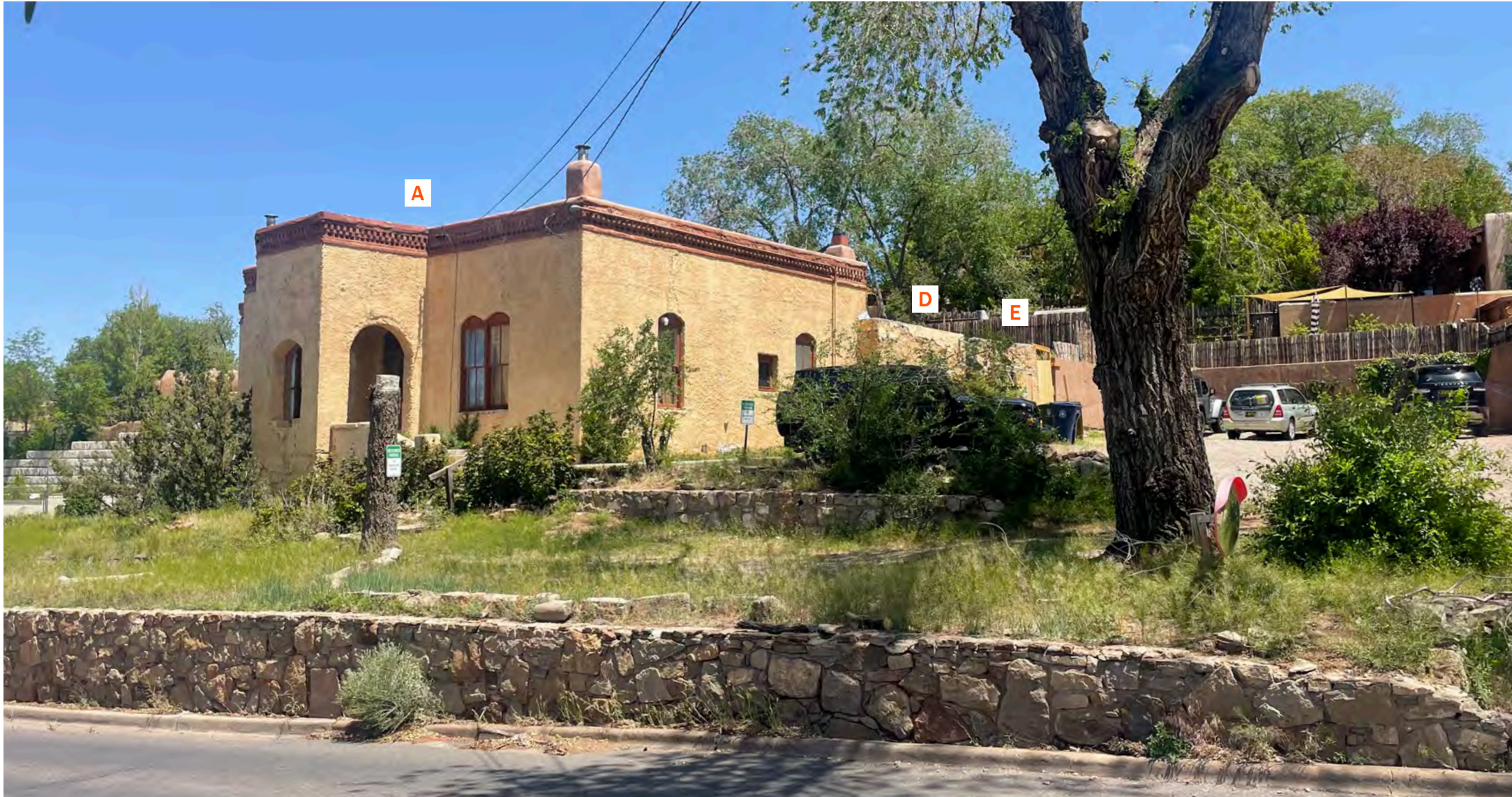
SITE FROM SOUTHEAST
