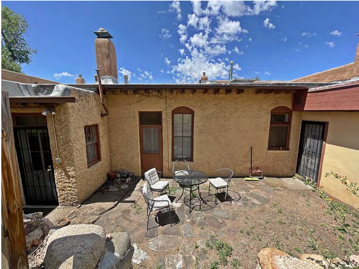
Photo 11: North elevation. Original garage (left); bedroom addition (right). Camera facing southeast.
