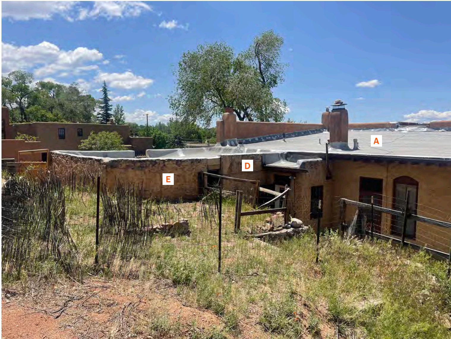
SITE FROM NORTH — TOWARD RUBBLE GARAGE
