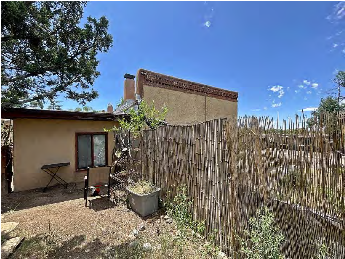
Photo 14: West elevation of bedroom addition. Camera facing southeast.
