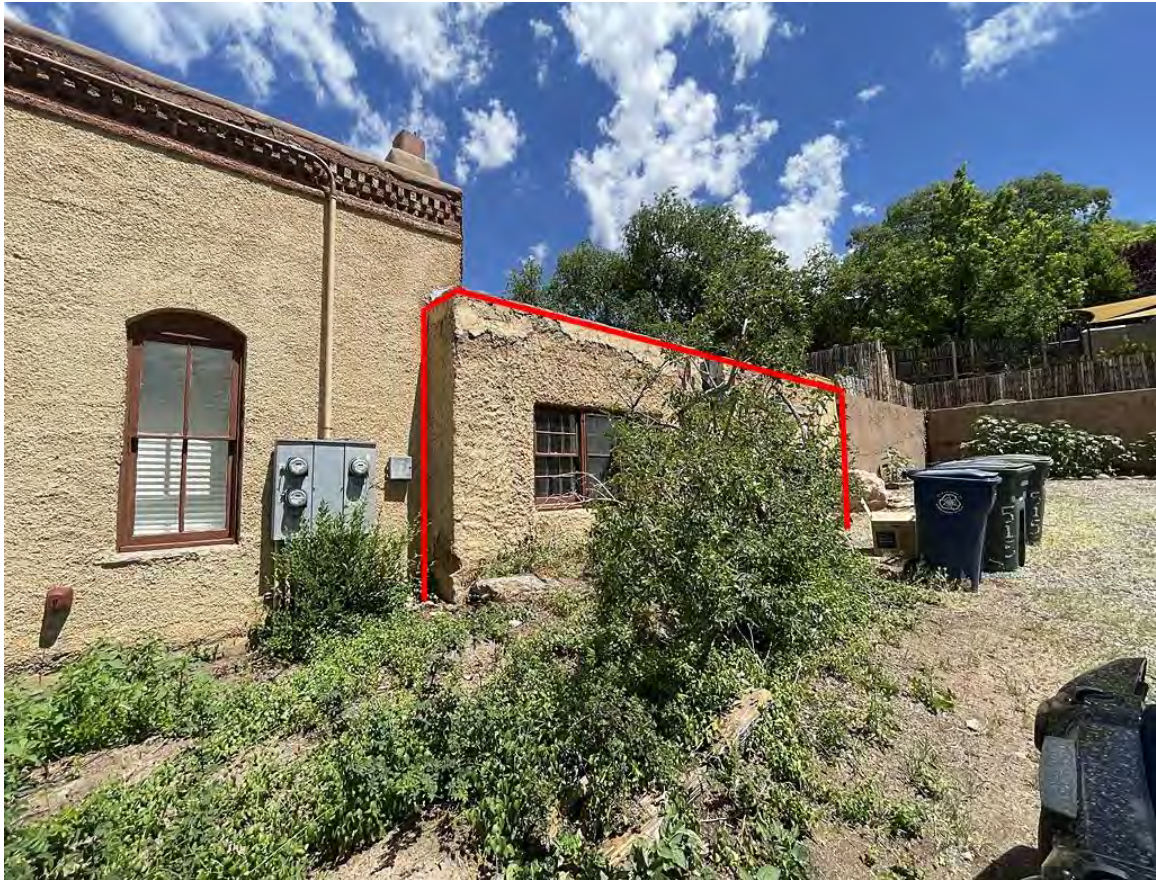
Photo 7: East elevation oblique. Two garage additions highlighted. Camera facing north.
