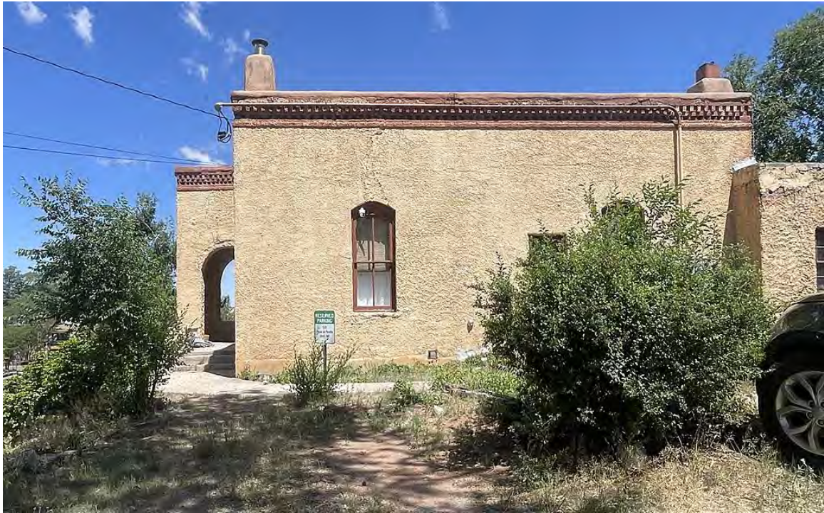
Photo 6: East elevation of the original building. Camera facing northwest.
