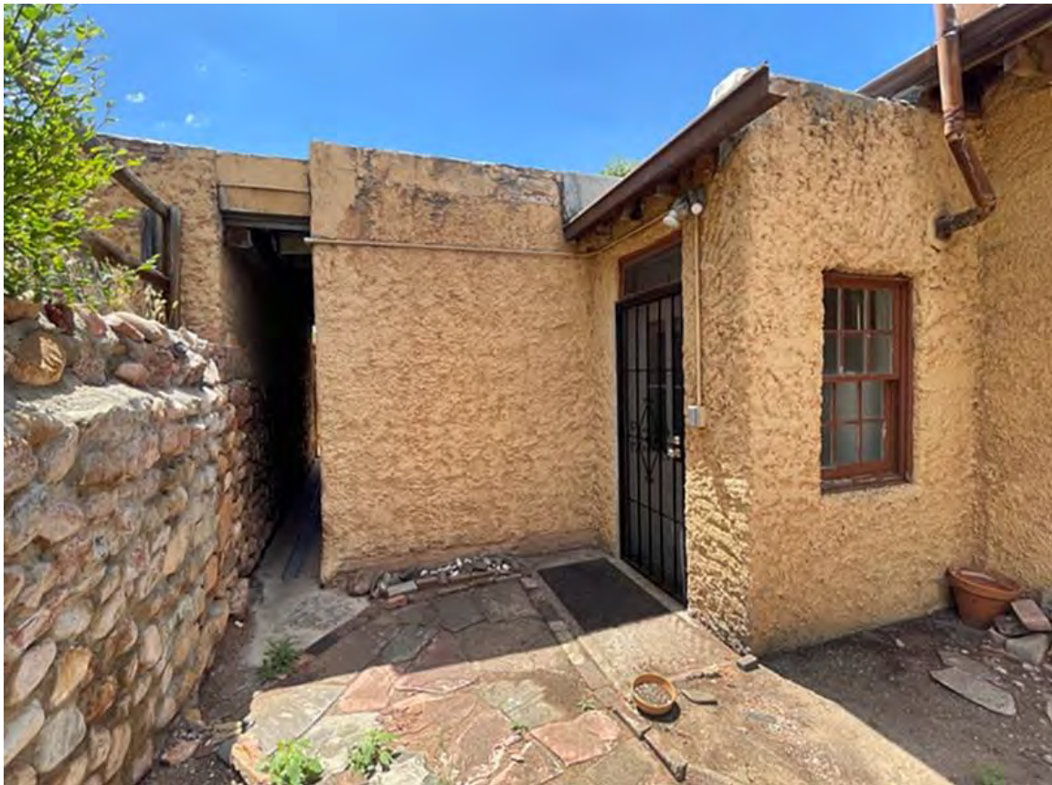
Photo 20: North retaining wall. Camera facing southeast.
