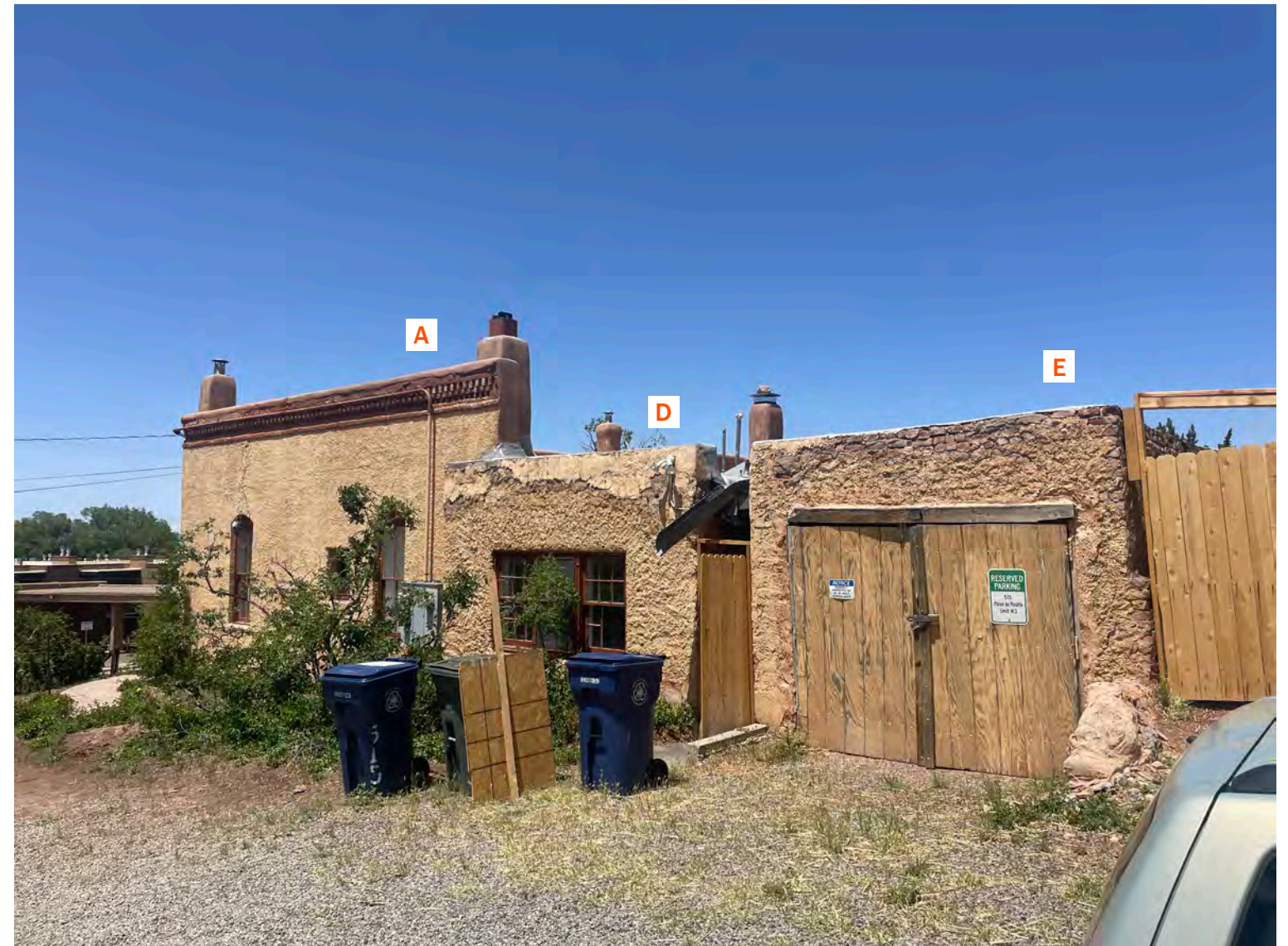
SITE FROM EAST
