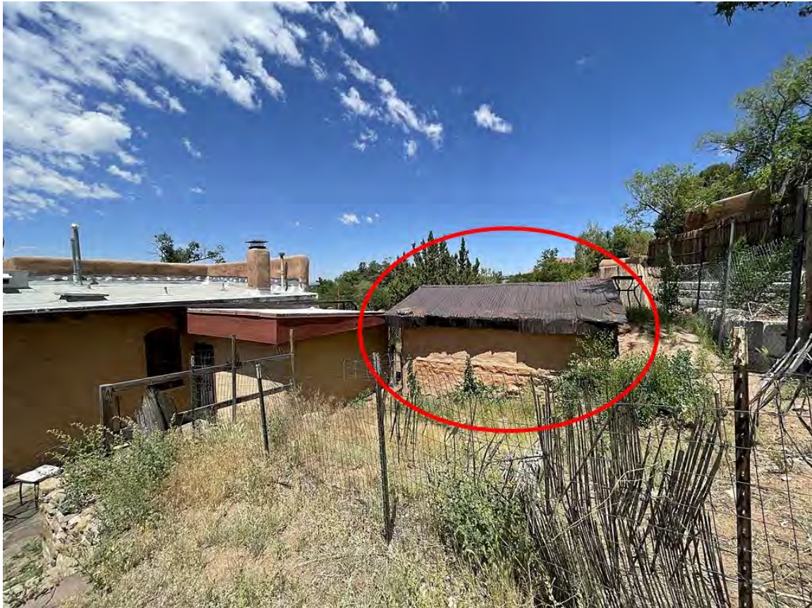
Photo 15: Shed. East elevation. Camera facing northwest.
