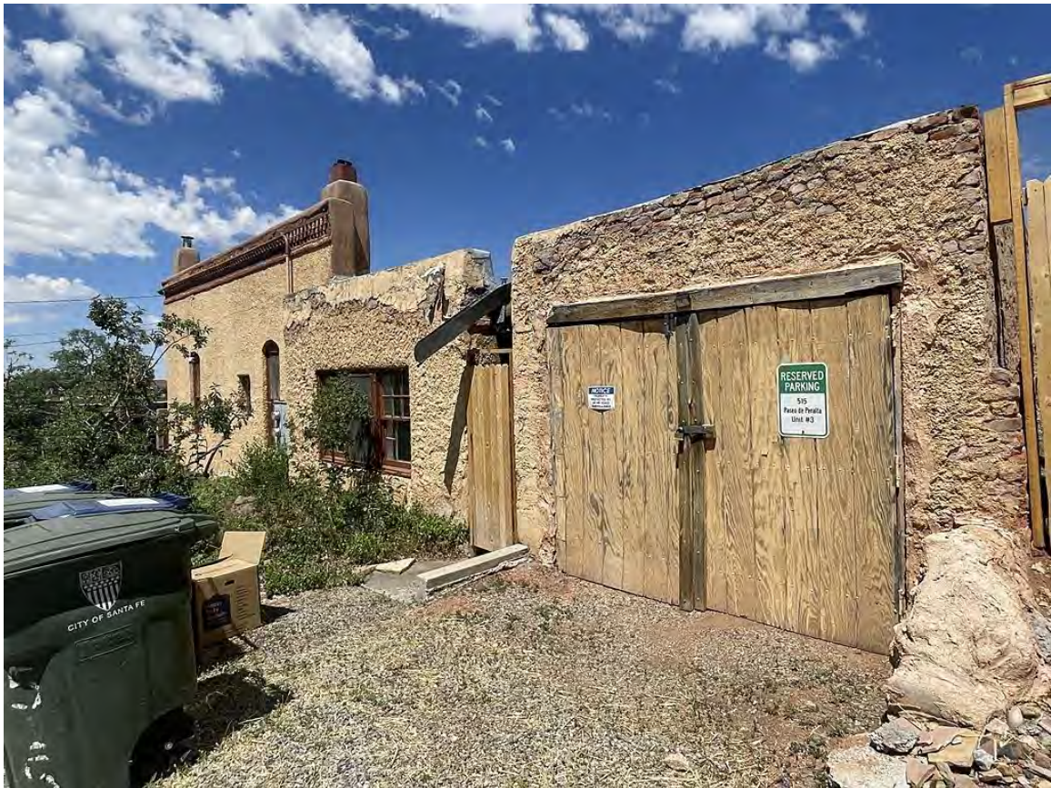
Photo 9: East elevation oblique. Later garage at right. Camera facing southwest.
