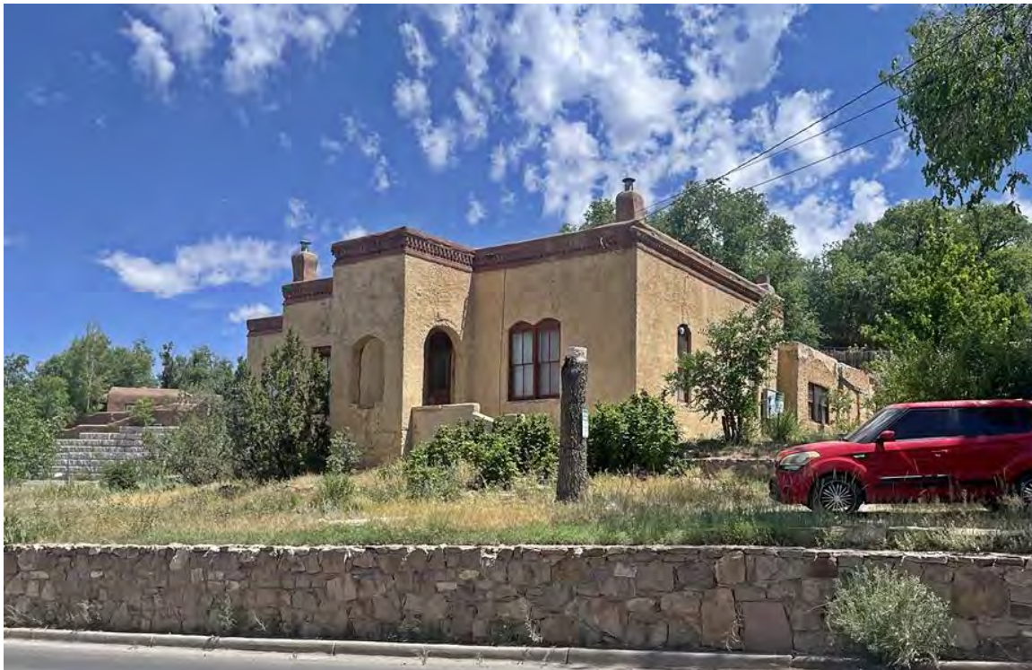
Photo 2: Setting. Camera facing northwest.
