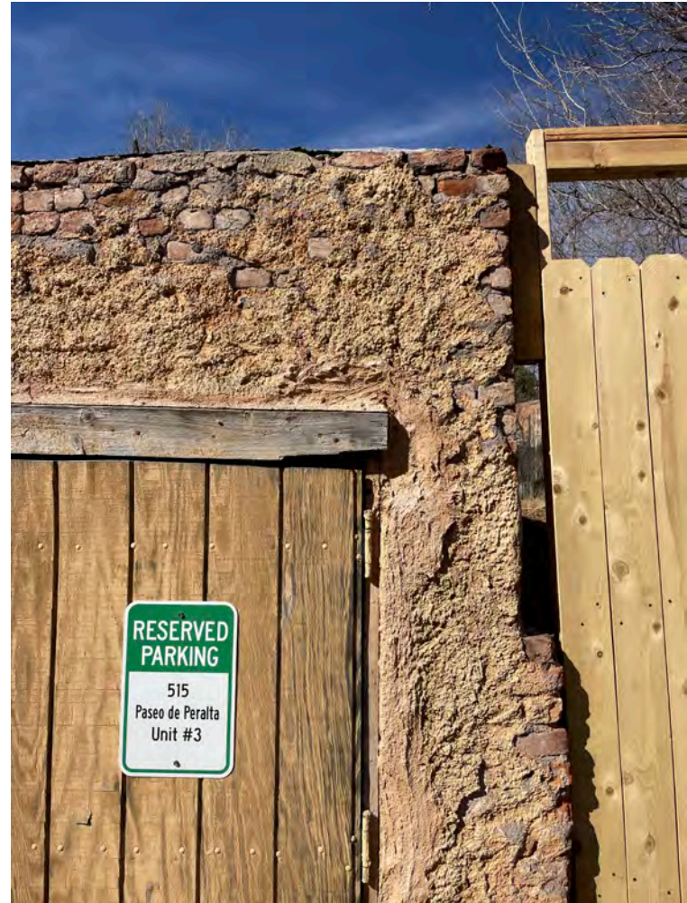
DETERIORATING BRICK
