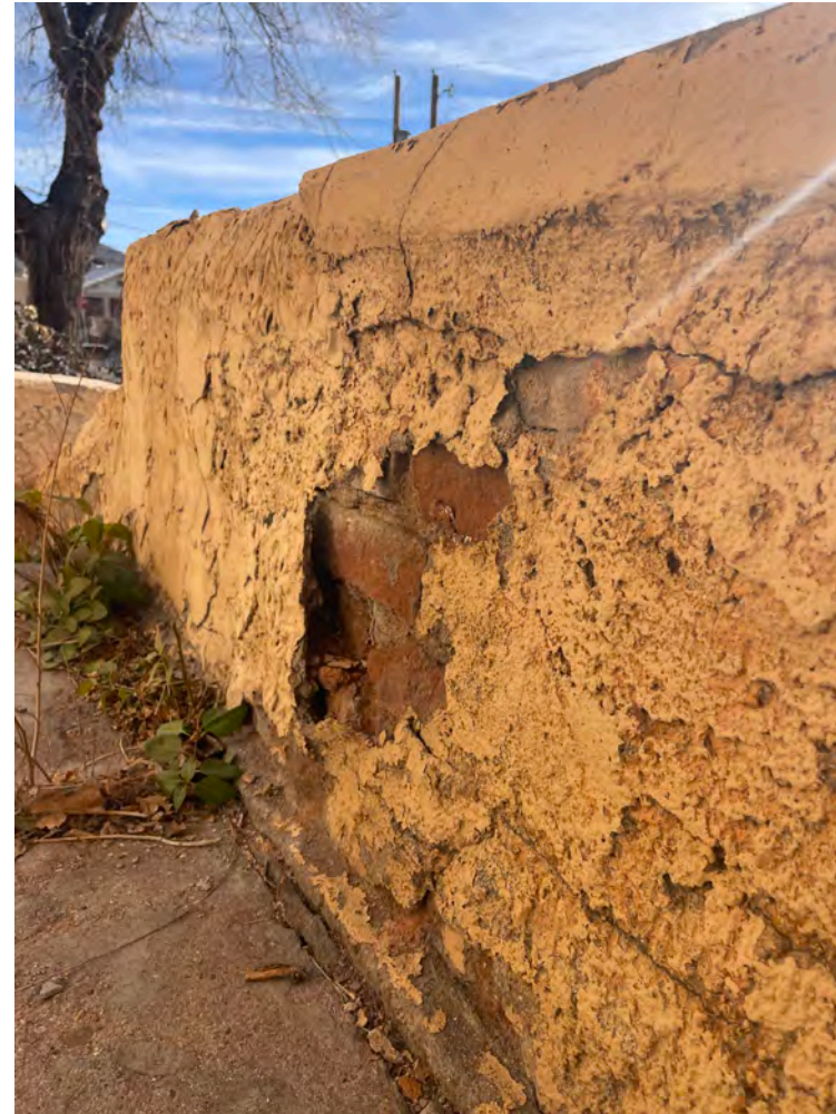
STUCCO & BRICK BENEATH
