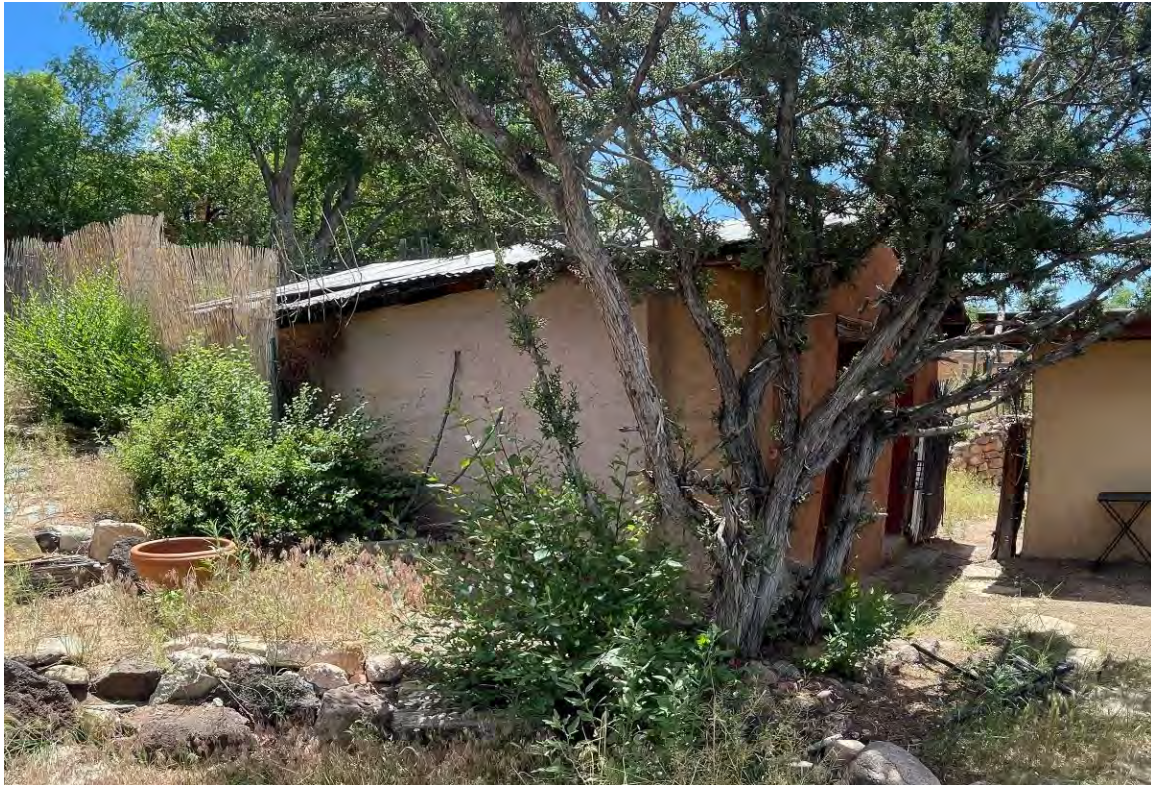
Photo 17: Shed. West elevation. Camera facing northeast.
