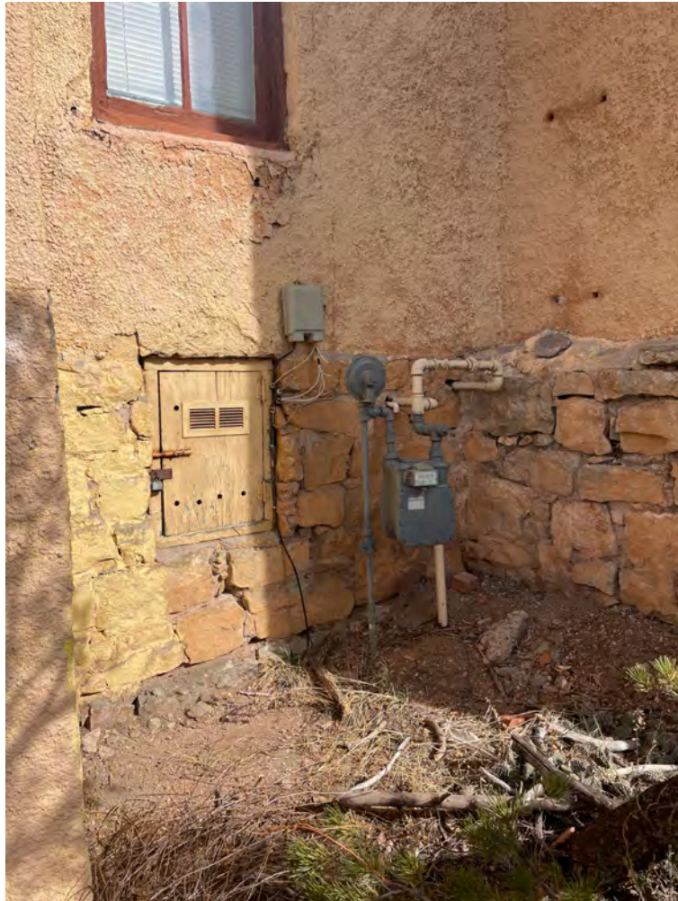
EXPOSED RUBBLE FOUNDATIONS
