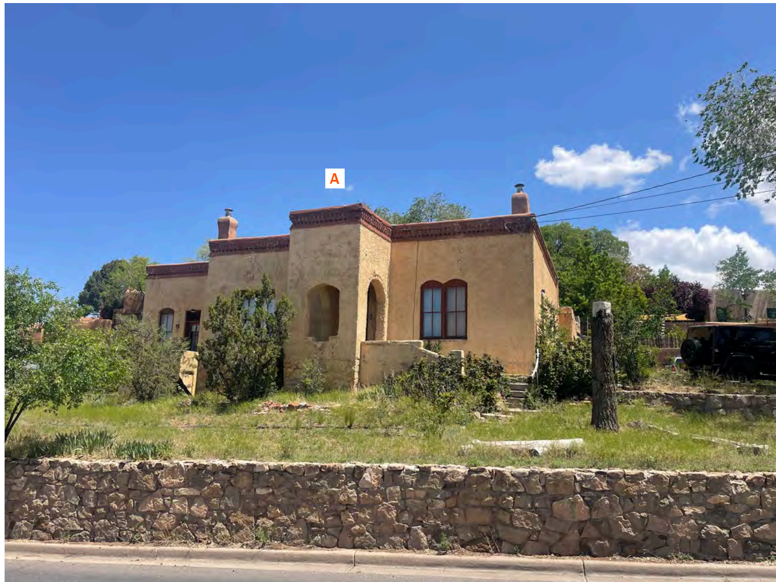
SITE FROM SOUTH
