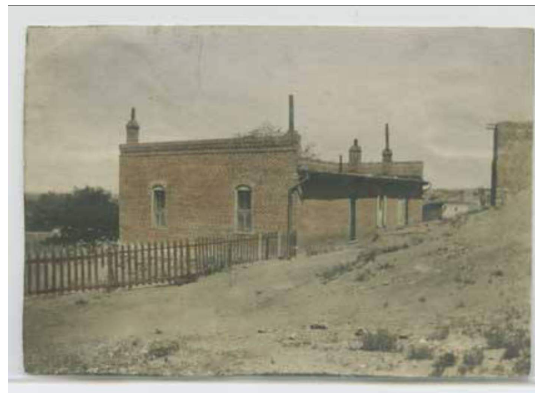
East facade, approx. 1910
