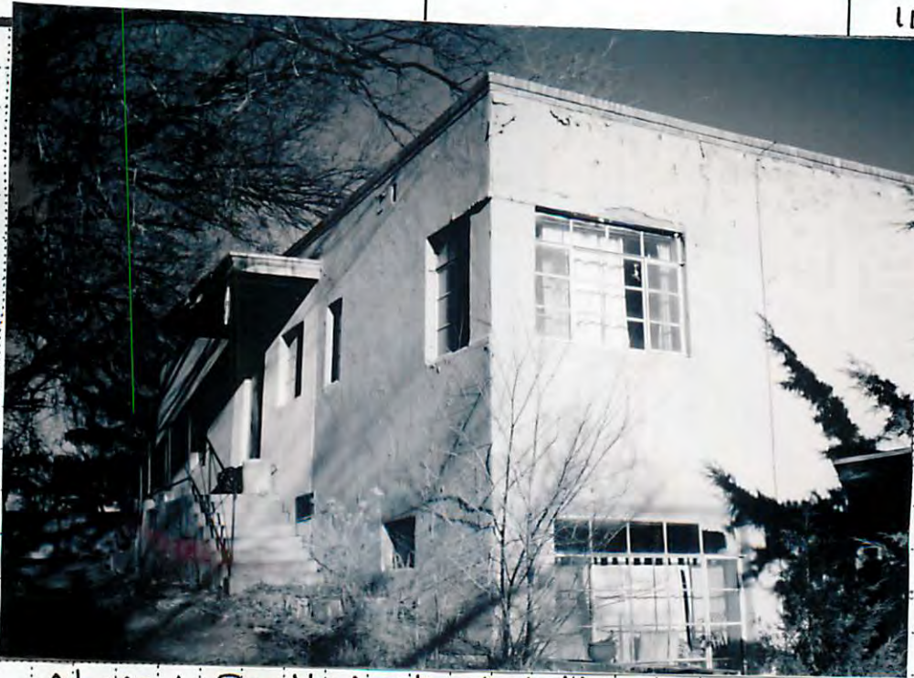
Above: Southwest elevation
