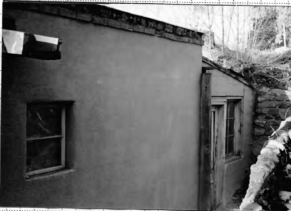
Above: Detail of rear east elevation
