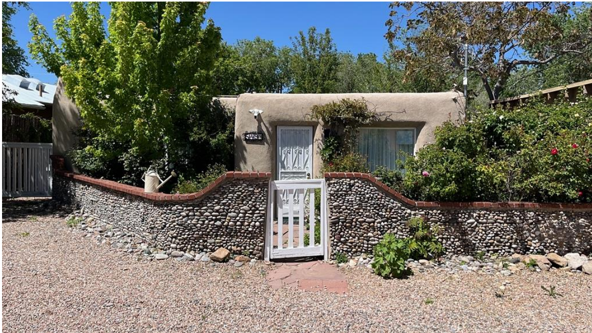
Photo 4: Subject dwelling and context. Camera facing north.
