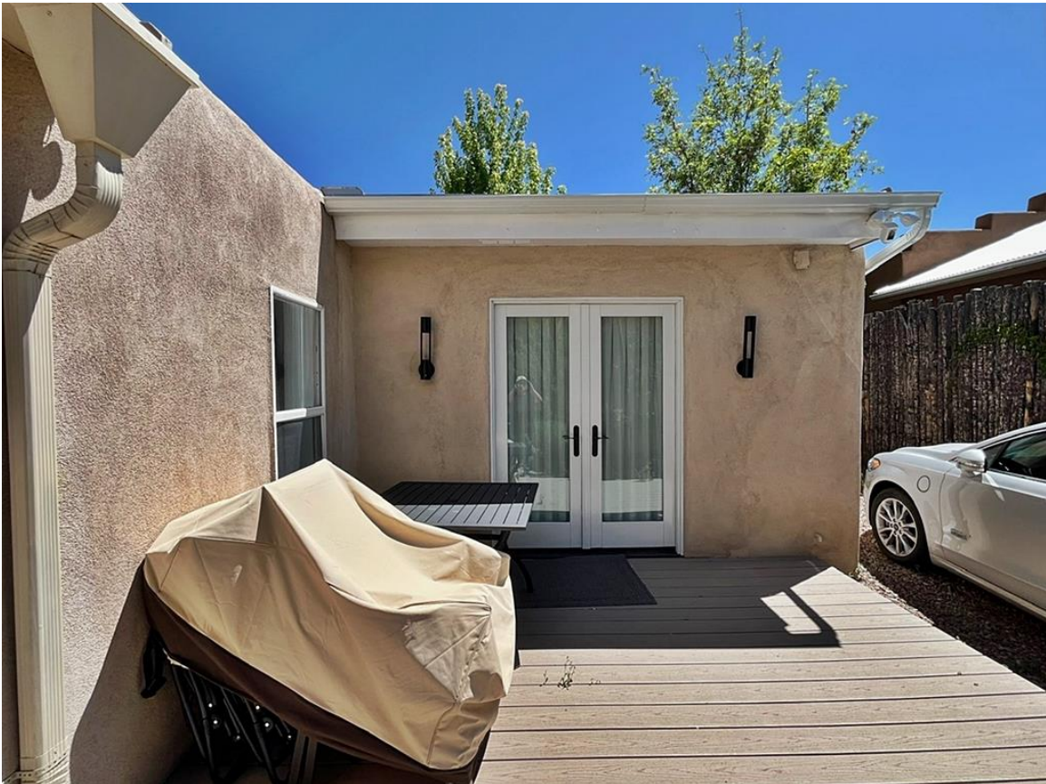
Photo 10: North elevation. Recent doors in 1960s addition. Camera facing south.
