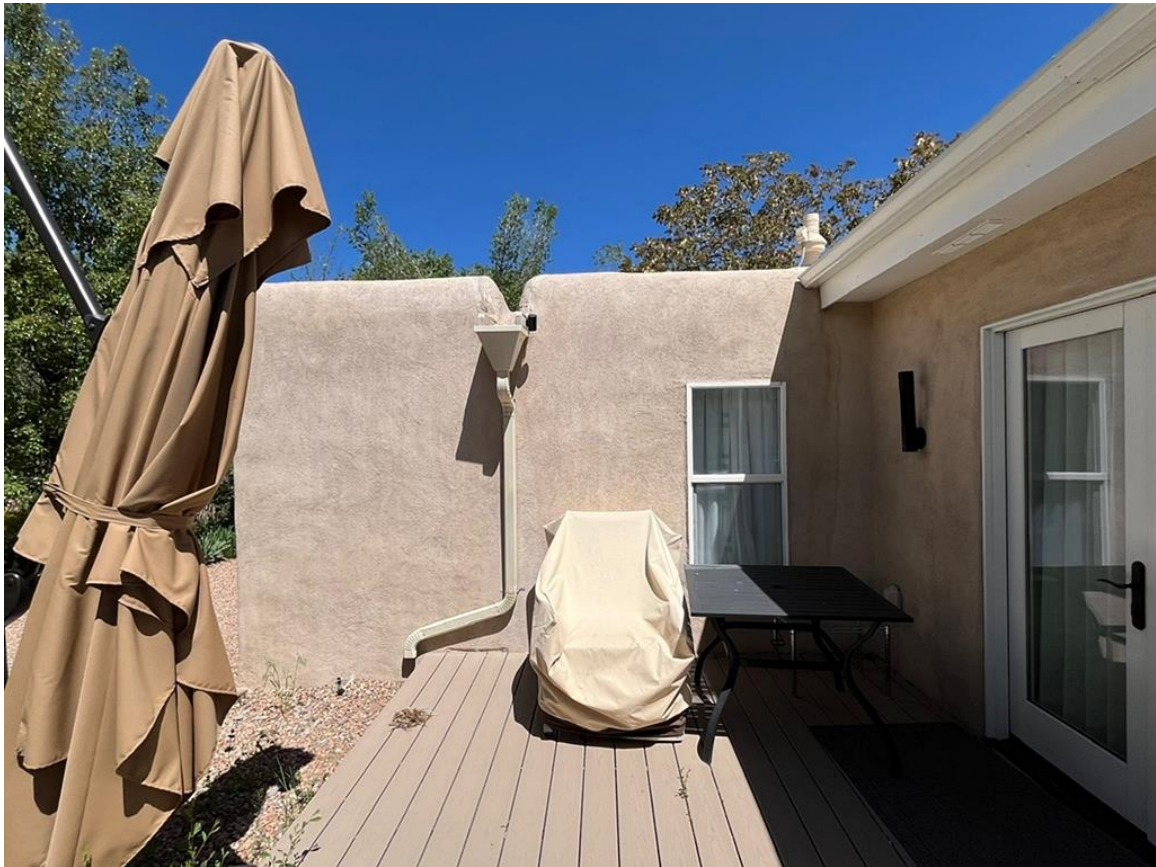
Photo 8: West elevation. Window in 1940s addition. Camera facing east.
