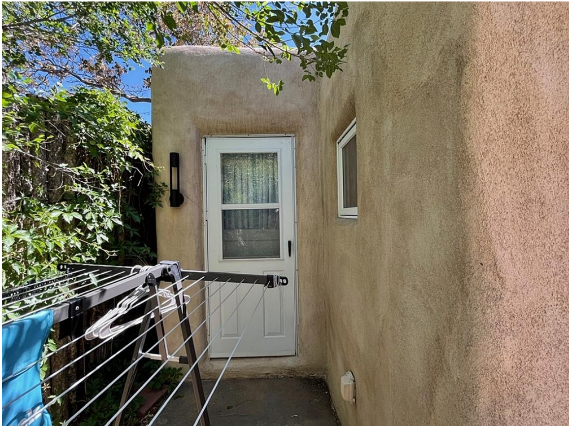
Photo 12: East elevation, north end. Window and door in 1940s addition. Camera facing south.
