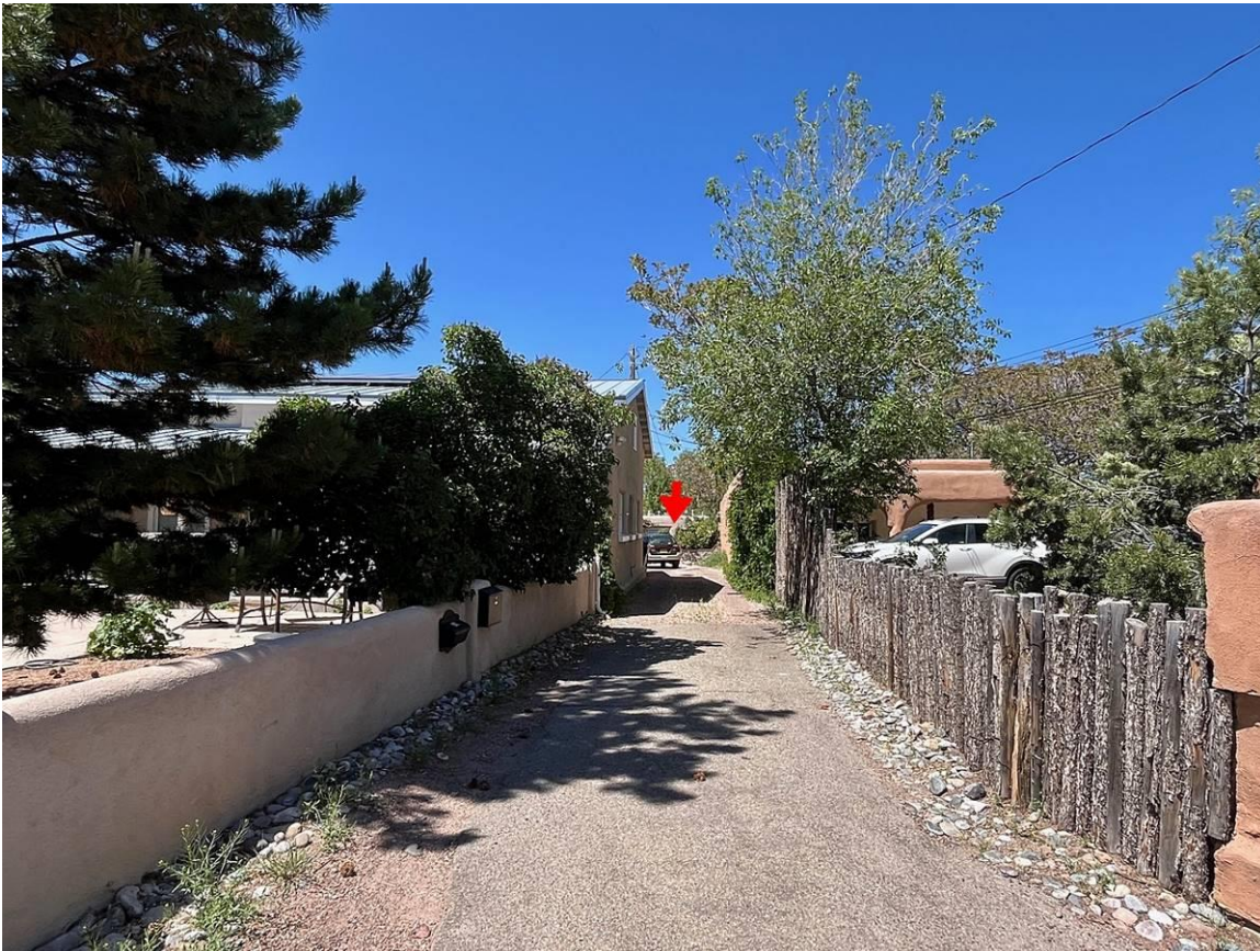
Photo 2: View of Hesch-Gonzales Cottage (arrow) from north side on Agua Fria Street. Camera facing north.
