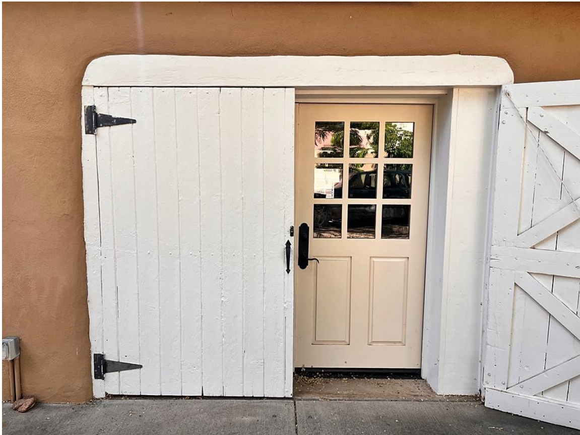
Photo 15: Garage/Carport. East elevation door. Camera facing west.
