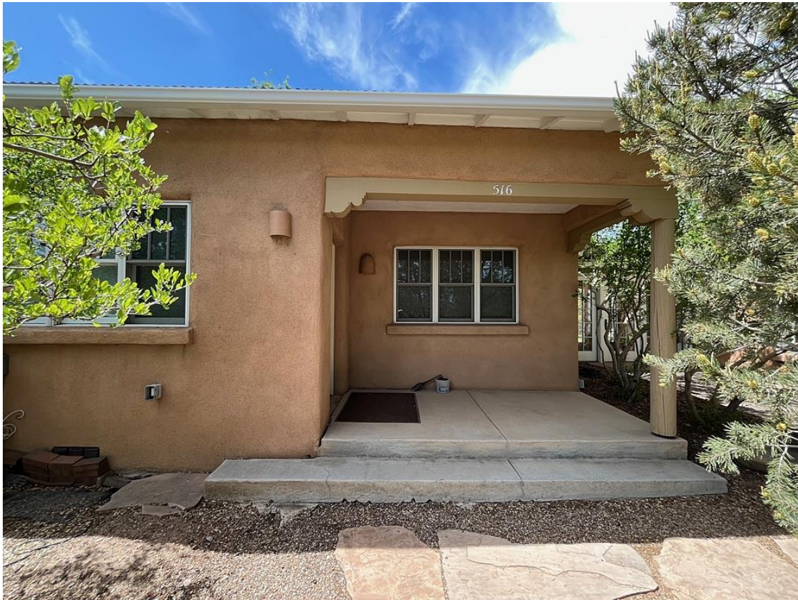
Photo 5: North façade of 516. Camera facing south.
