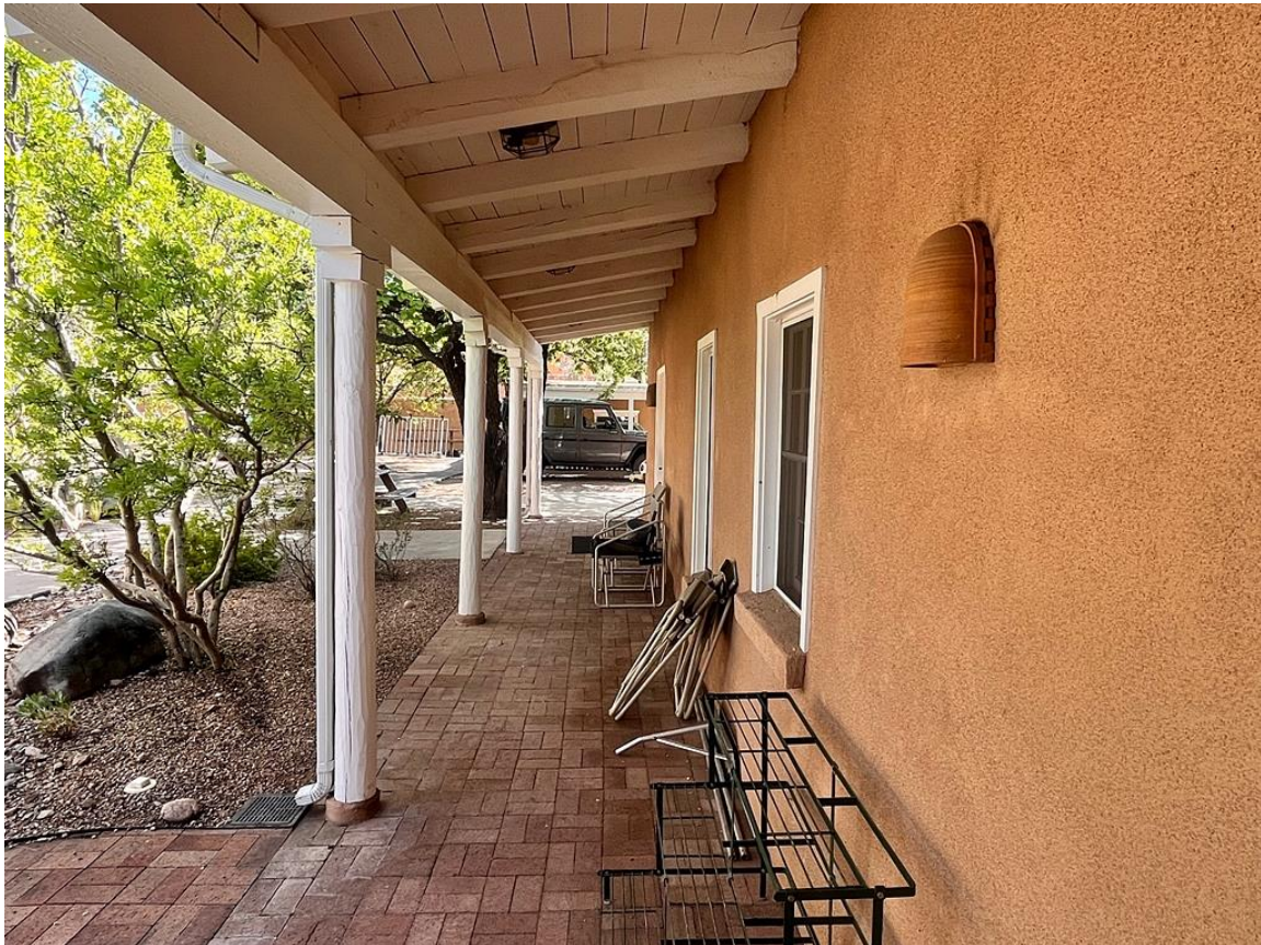
Photo 12: East (courtyard) elevation of 516 ½ with reconstructed porch. Camera facing south.
