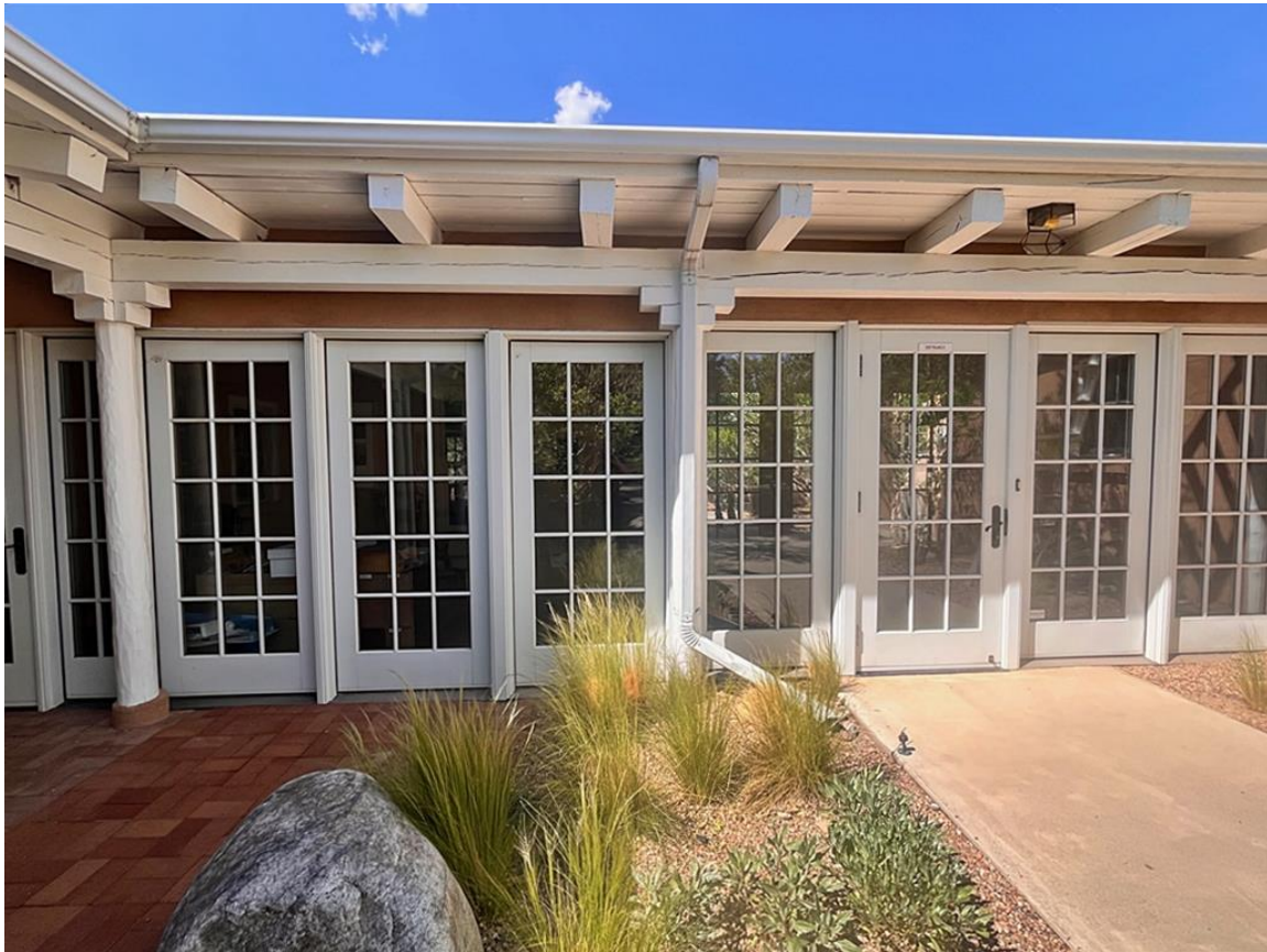
Photo 9. Glazed corridor between 516 and 516 ½. Camera facing north.
