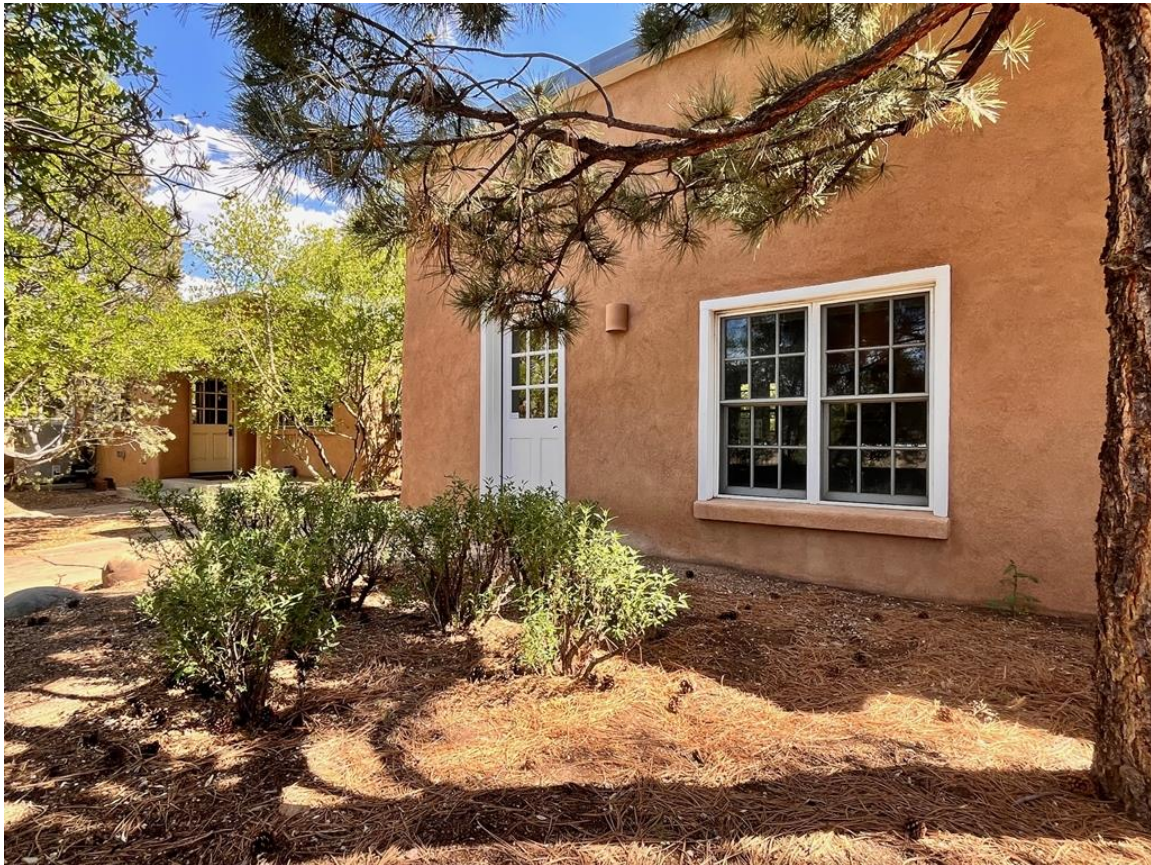
Photo 3: North façades of 516 (left) and 516 ½ (right). Camera facing southeast.
