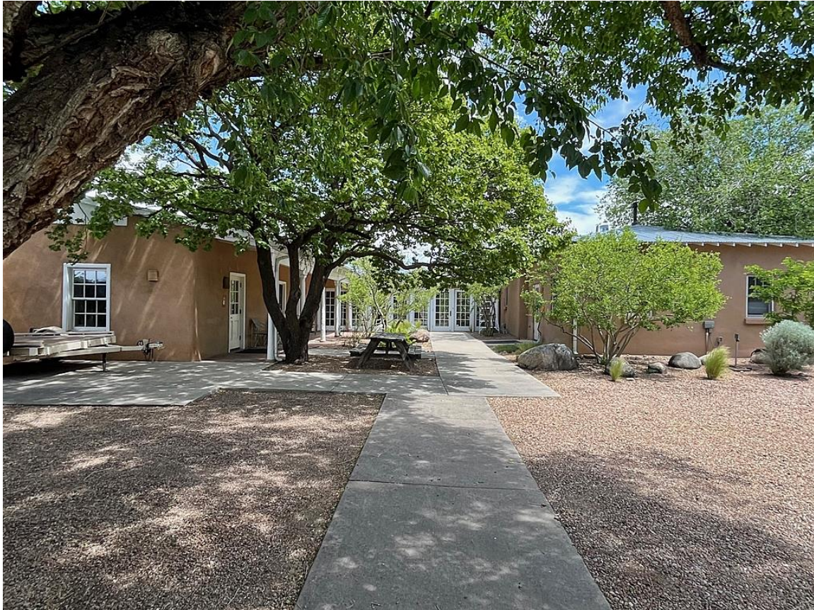
Photo 8: Courtyard elevation. Camera facing north.
