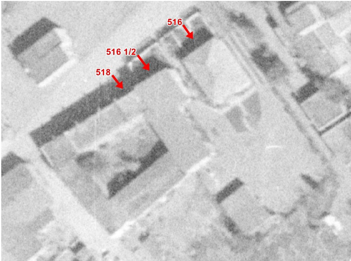
Figure 4: November 10, 1958, aerial photograph.
