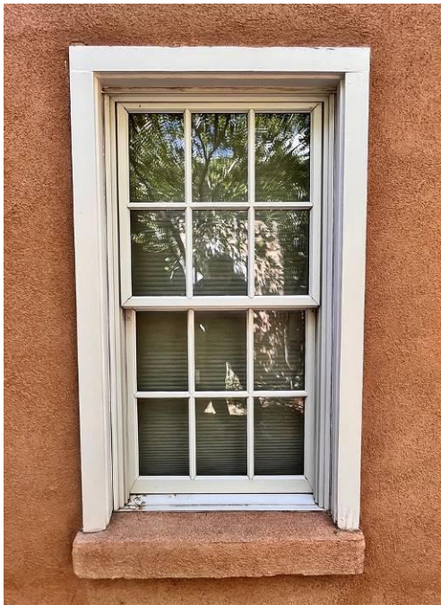
Photo 2: Reconstructed window openings with 1990s Pella vinyl clad units.
