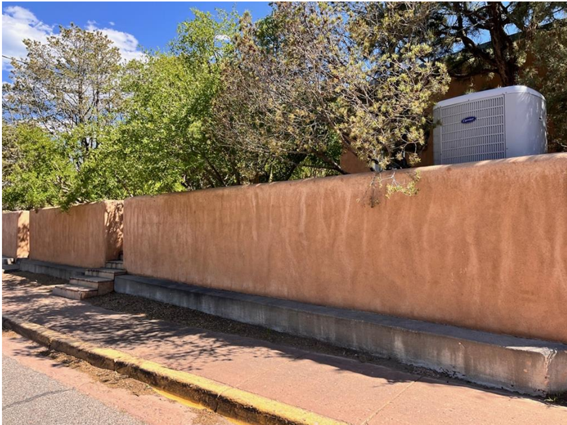
Photo 16: Alto Street retaining wall. Camera facing southeast.
