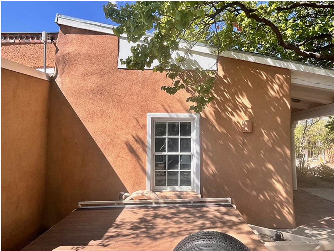
Photo 10: South elevation of 516 ½. Camera facing north.
