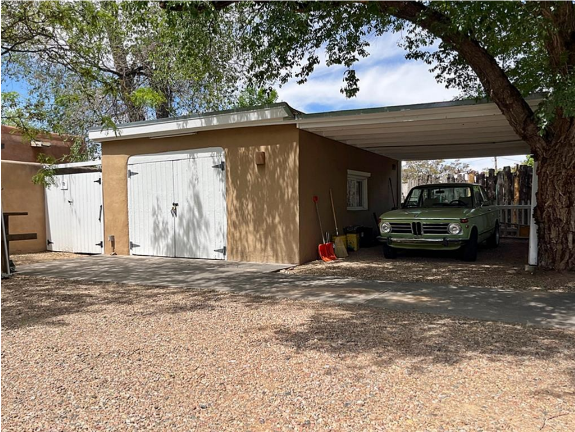
Photo 14: Garage/Carport. East elevation. Camera facing southwest.
