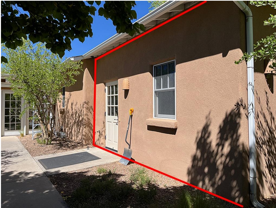
Photo 11: West (courtyard) elevation of c.1996 addition to 516. Camera facing northeast.
