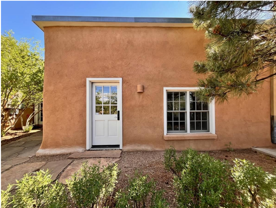
Photo 6: North façade of 516 ½. Camera facing south.
