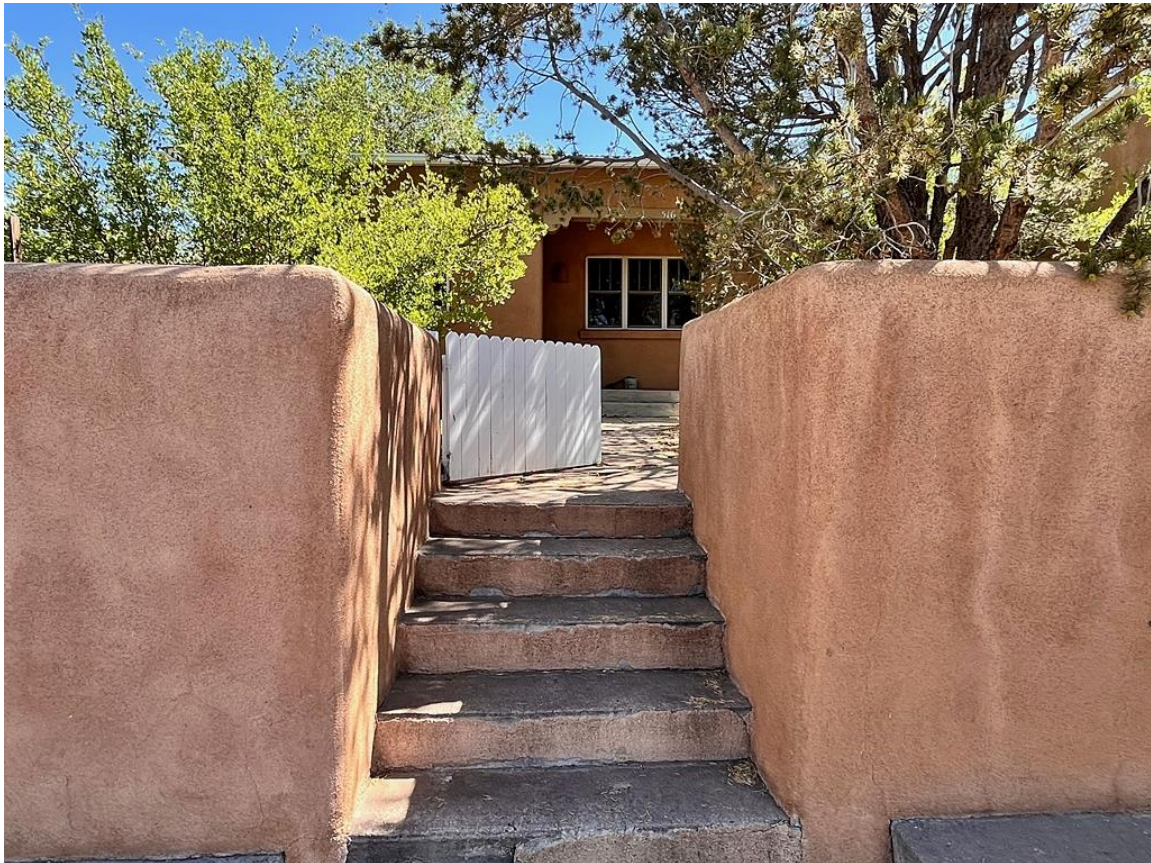
Photo 17: Alto Street retaining wall. Gate opening for 516. Camera facing south.
