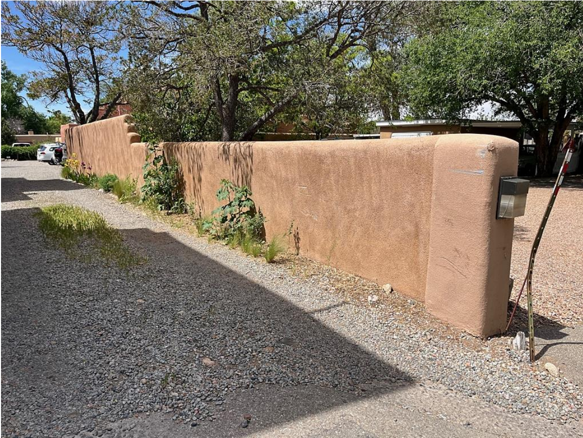
Photo 18: East and south perimeter walls. Camera facing southwest.
