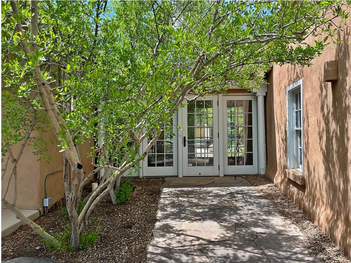
Photo 4: Glazed corridor between 516 and 516 ½. Camera facing south.
