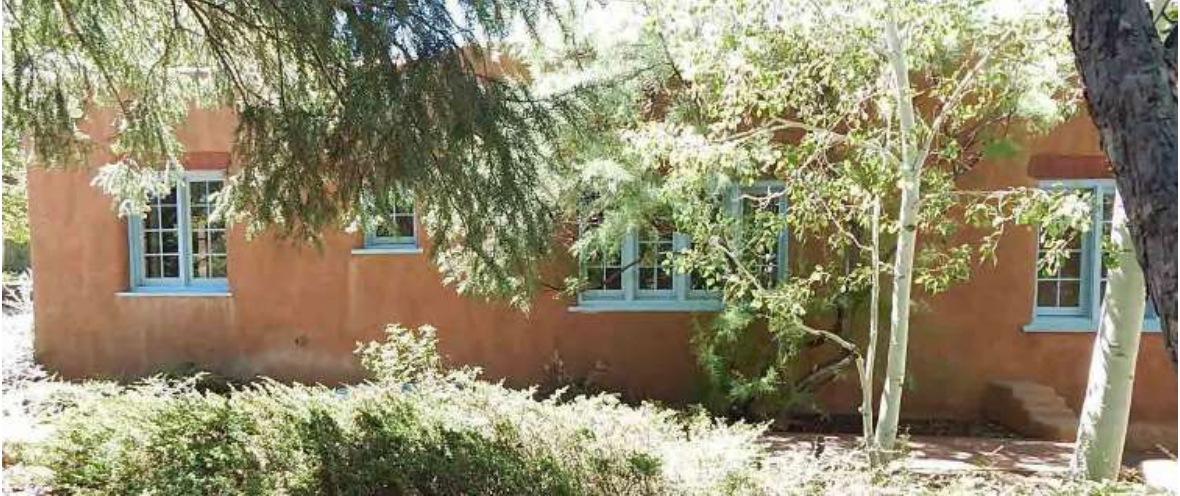
Figure 2. North Facade II.
