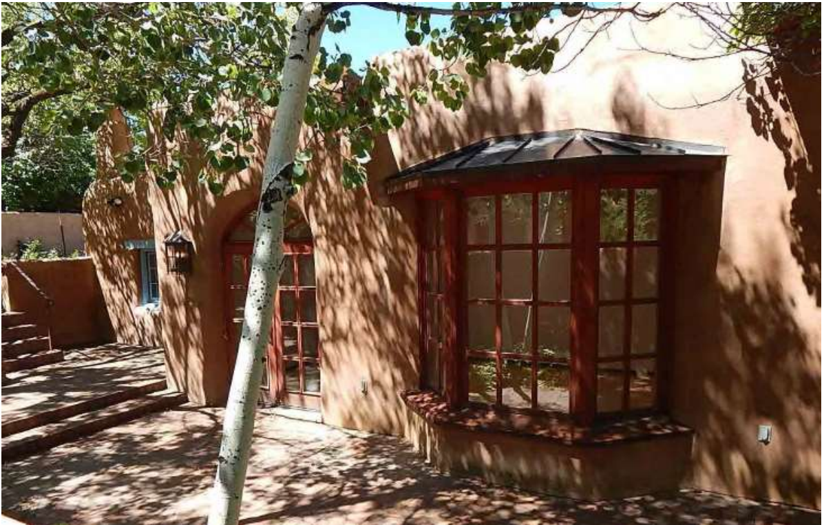
Figure 5. East Facade III.
