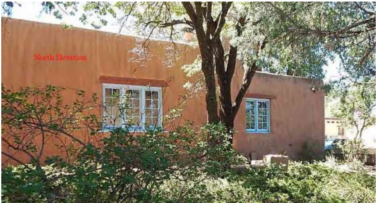
Figure 1. North Facade I.
