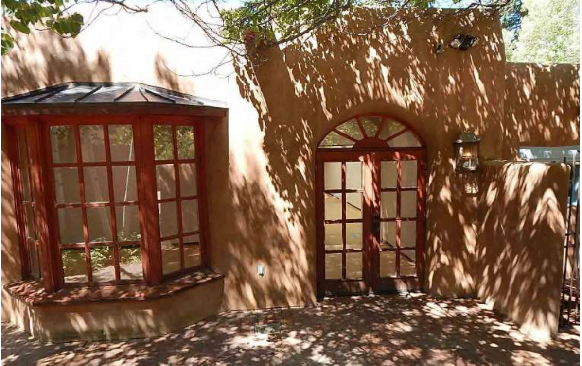
Figure 4. East Facade II.
