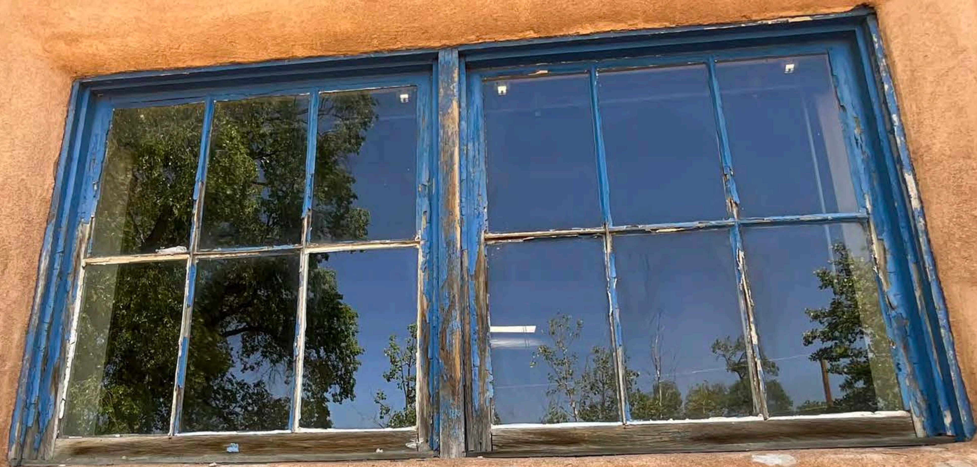
Main House Window MH-A
