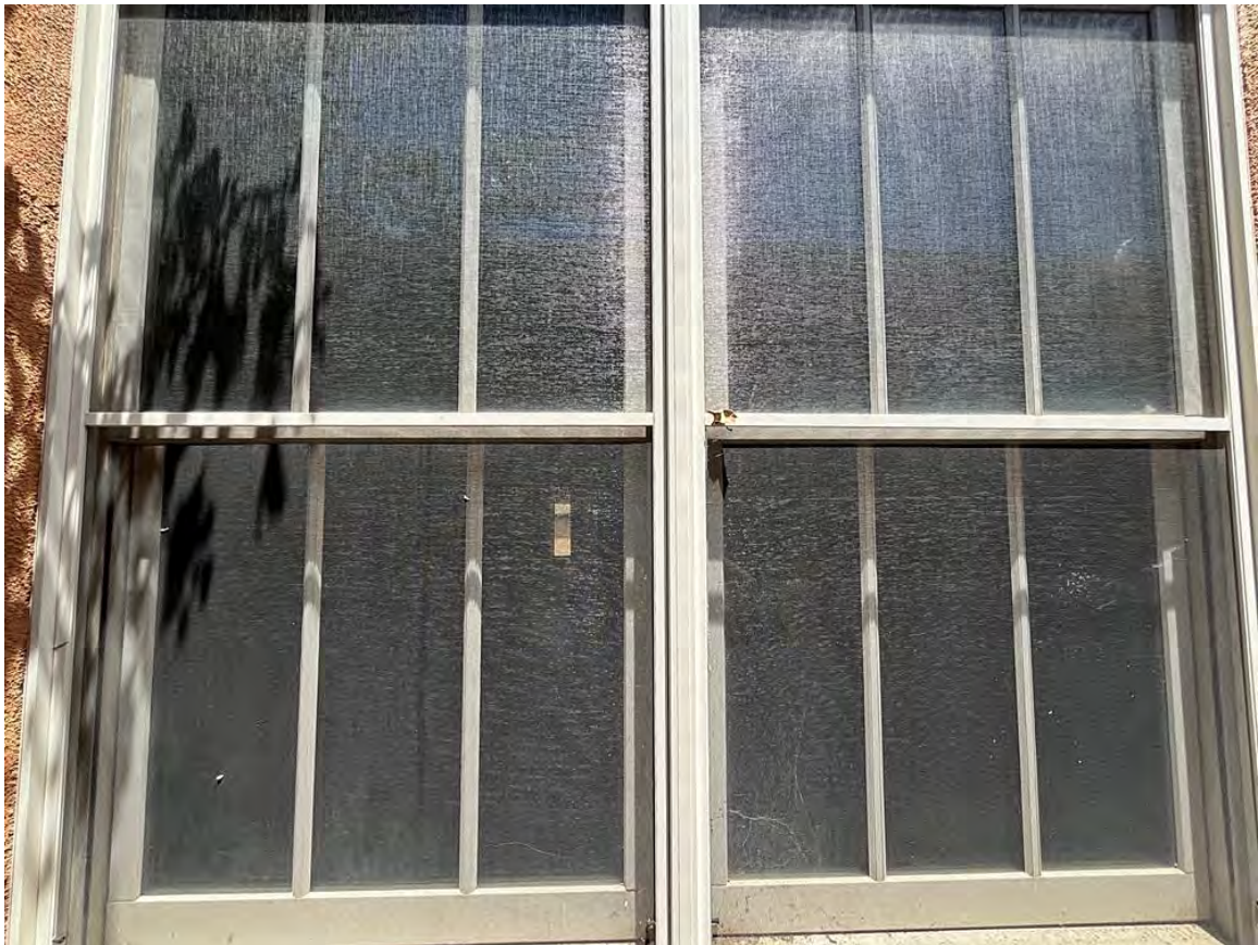
Photo 15: Primary House, south elevation. Middle window. Camera facing north.
