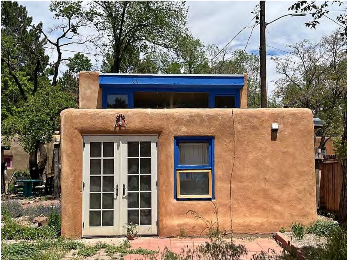
Photo 26: Guesthouse, south elevation. Camera facing north.
