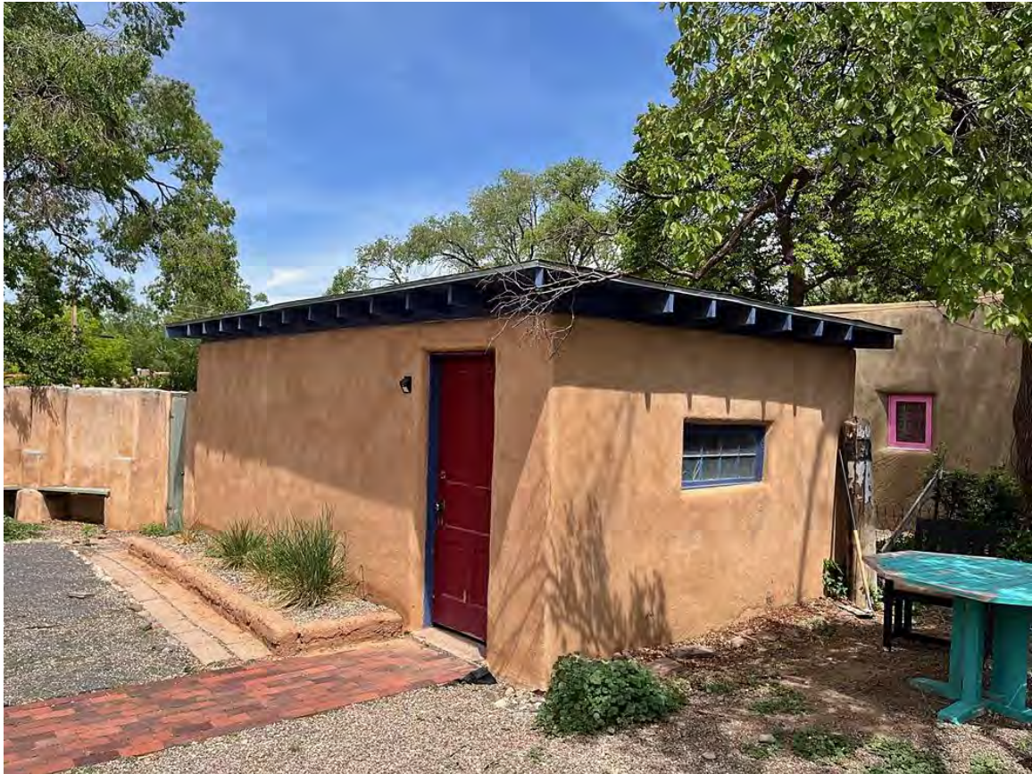
Photo 31: Garage, south and east elevations. Camera facing northwest.
