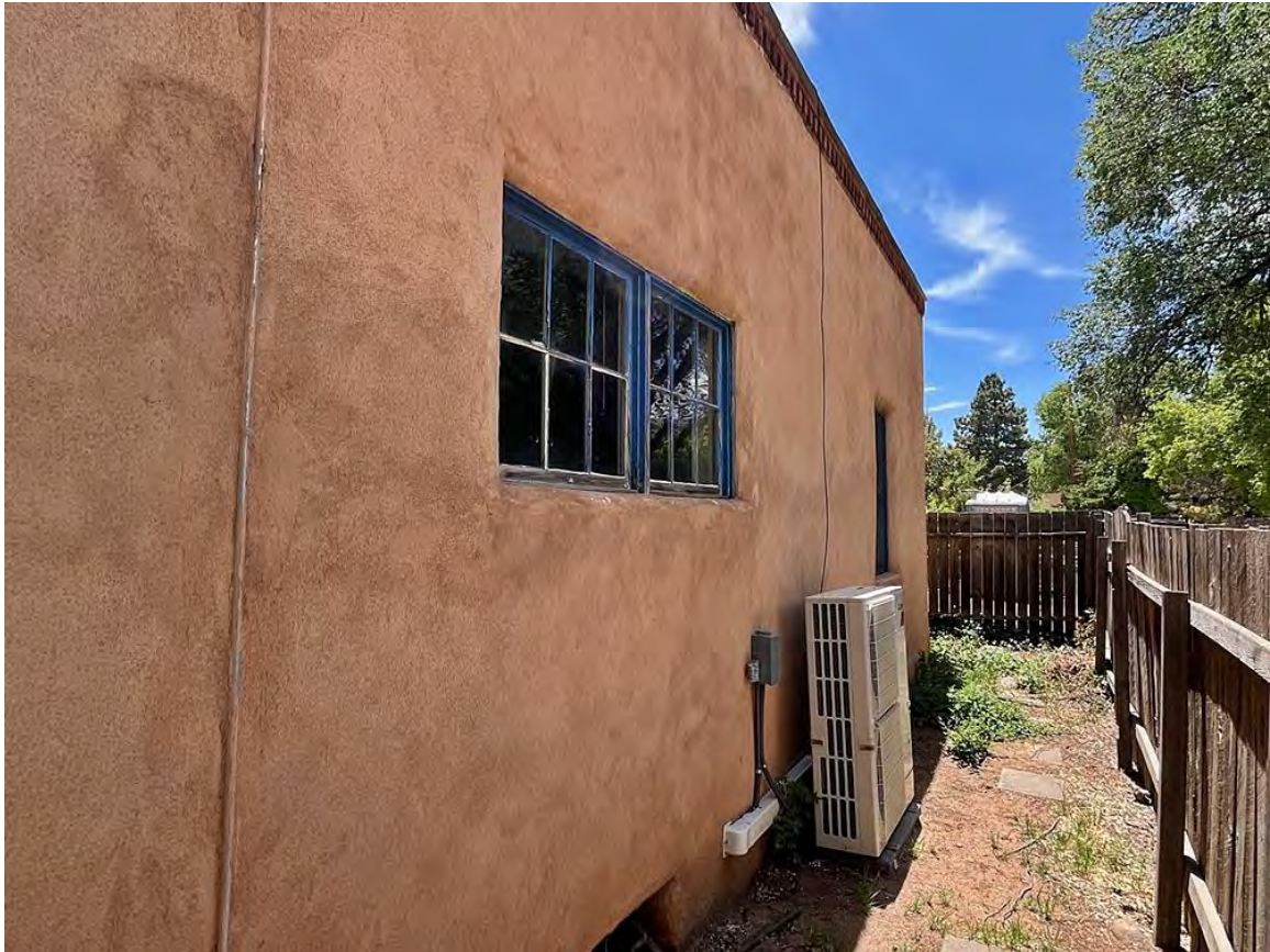
Photo 10: Primary House, west elevation. Camera facing south.
