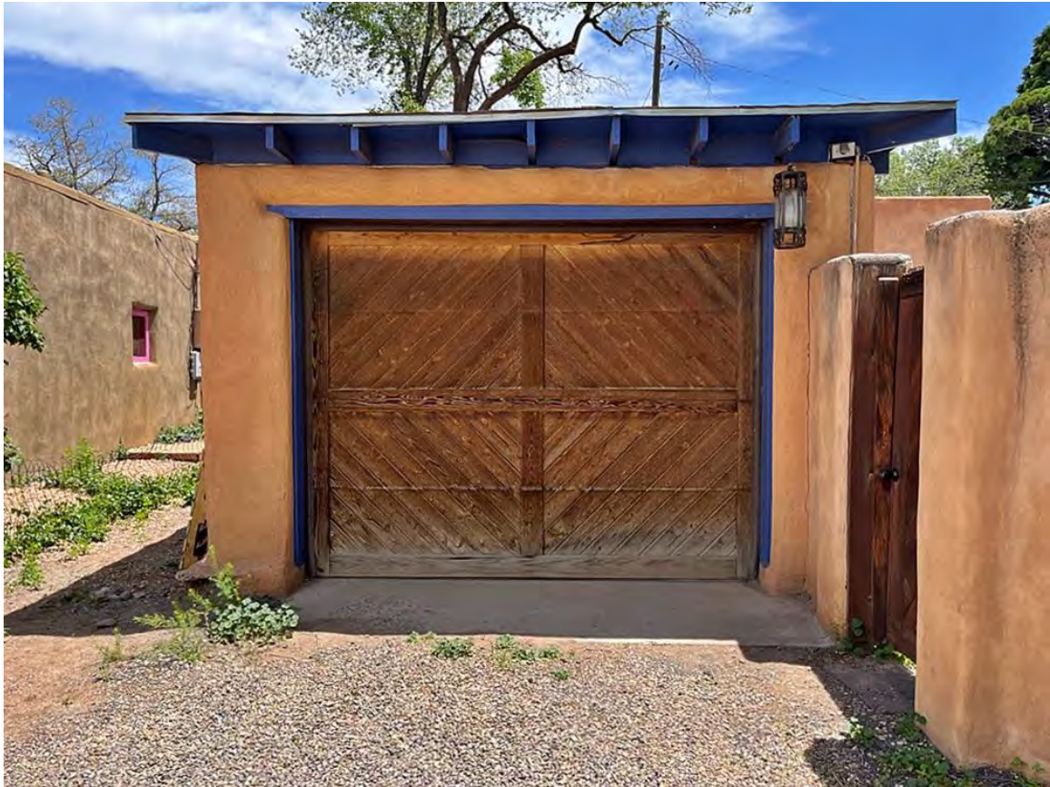
Photo 30: Garage, west elevation. Camera facing east.
