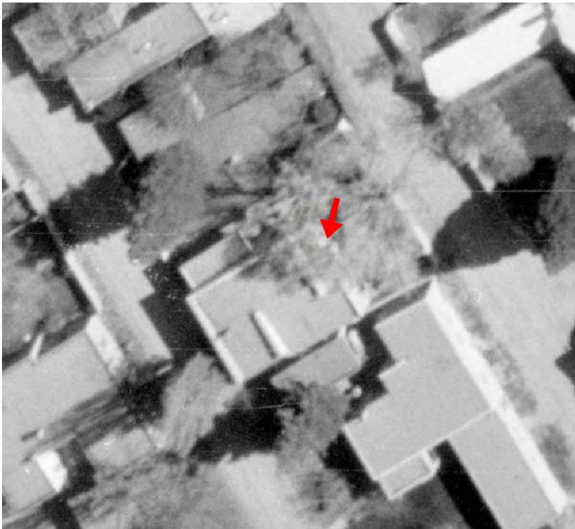
May 11, 1973, aerial photograph. Arrow: The closet-bathroom addition has been constructed.
