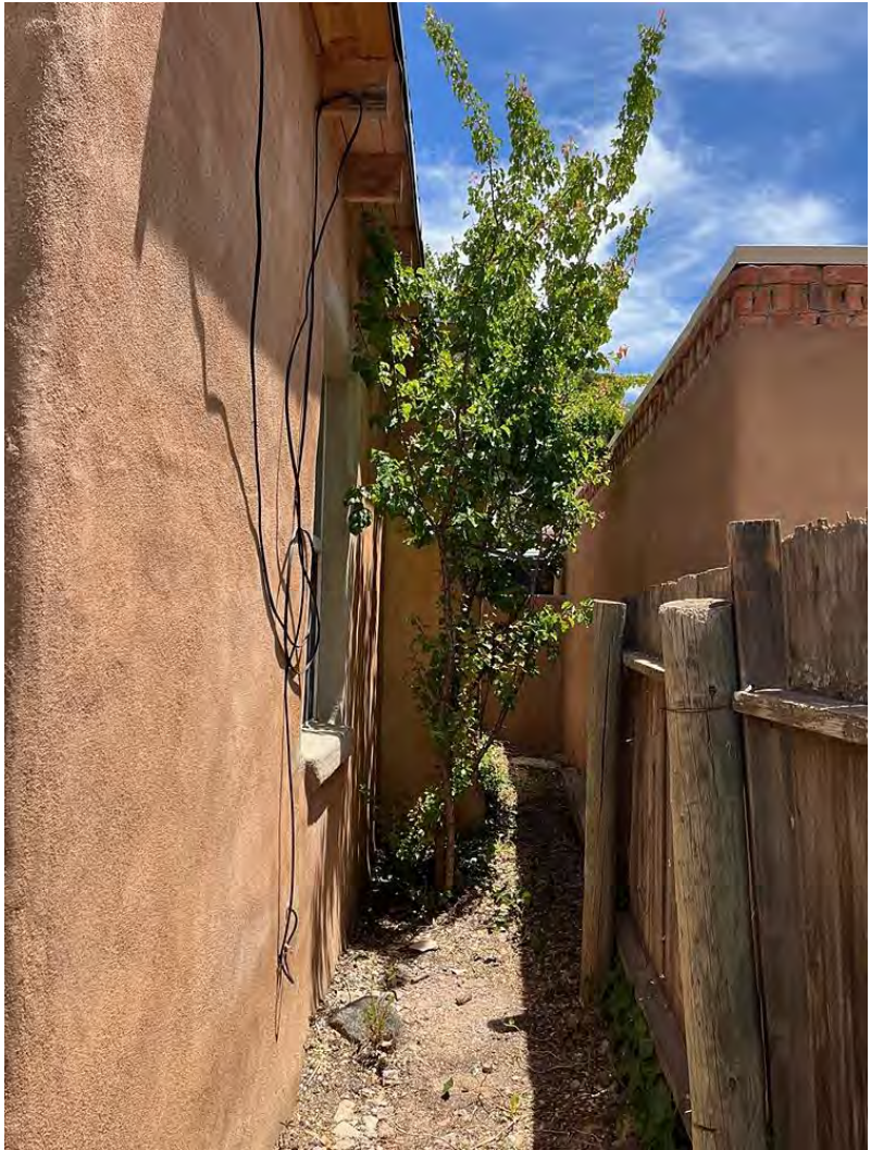
Photo 13: Primary House, south elevation. Camera facing east.
