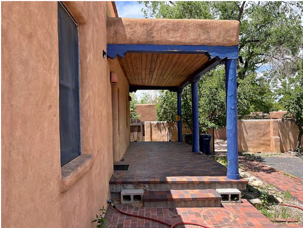
Photo 4: Primary House, north elevation. Portal. Camera facing west.
