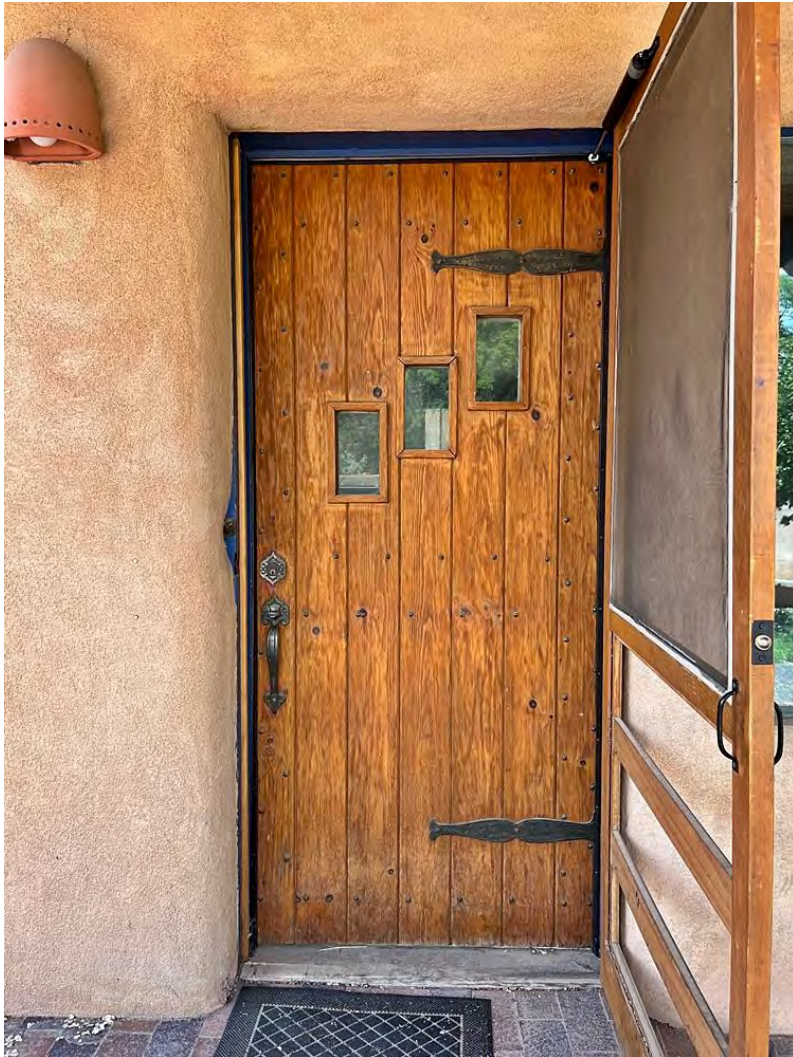
Photo 5: Primary House, north elevation. Entry door. Camera facing south.
