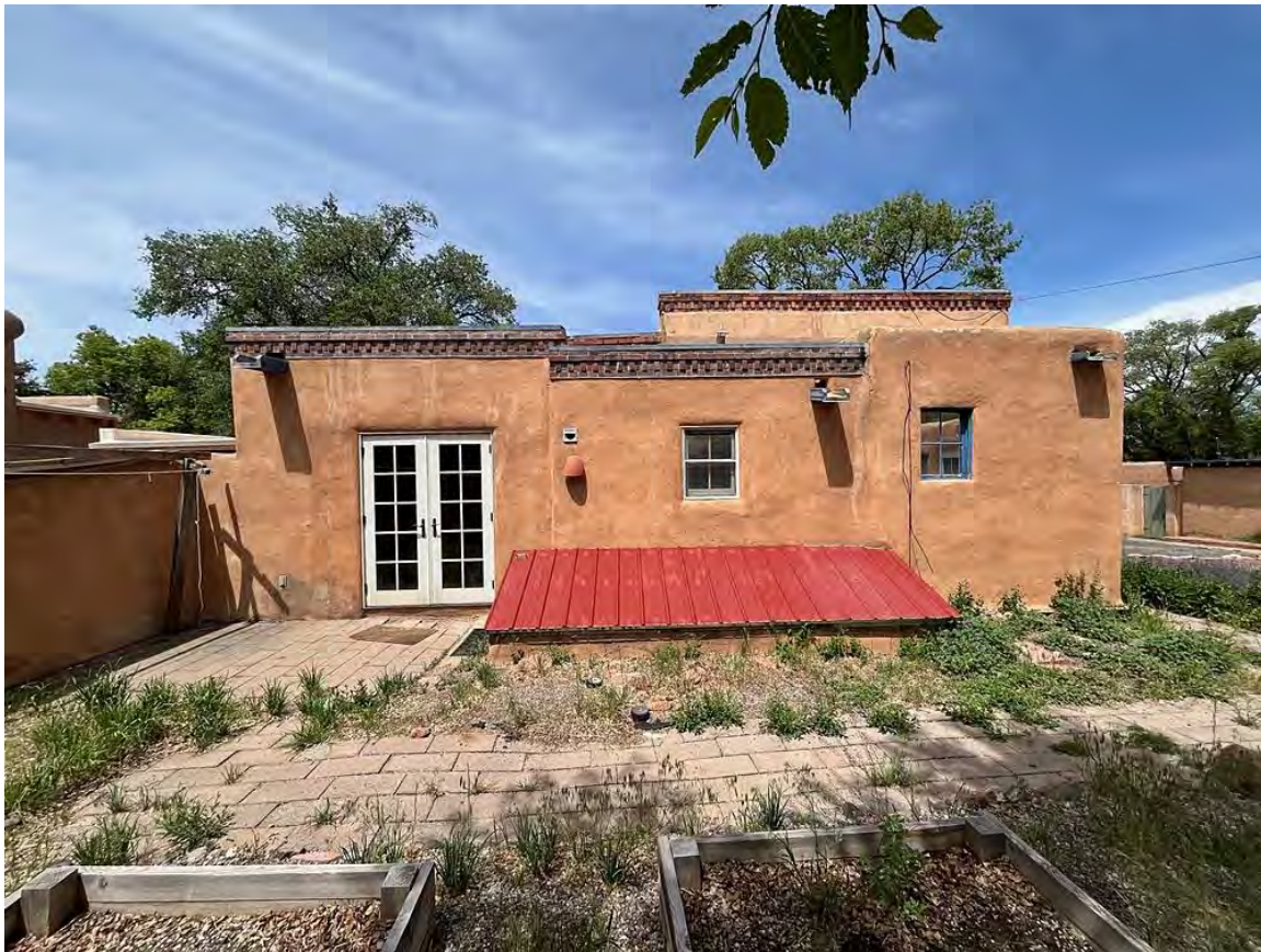
Photo 16: Primary House, east elevation. Camera facing west.
