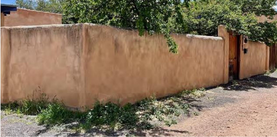
Figure 6: West Yard Wall
