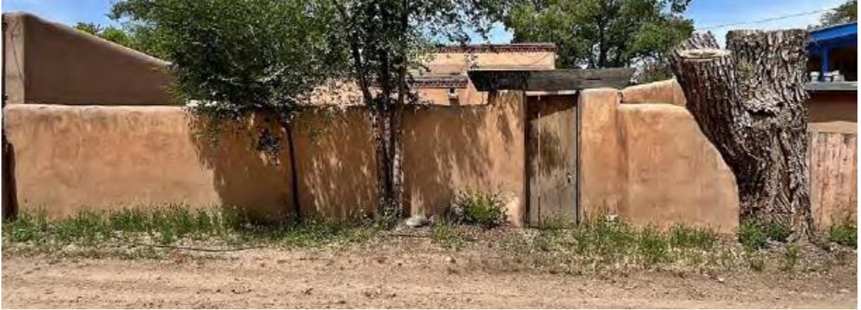
Figure 5: East Yard Wall
