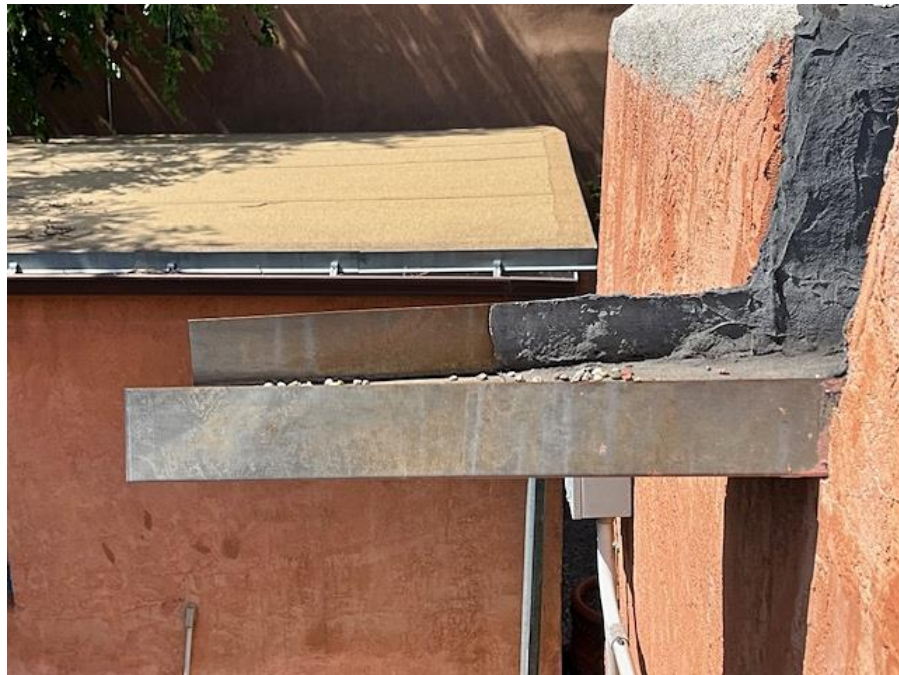
Figure 4: East elevation canale, side view.
