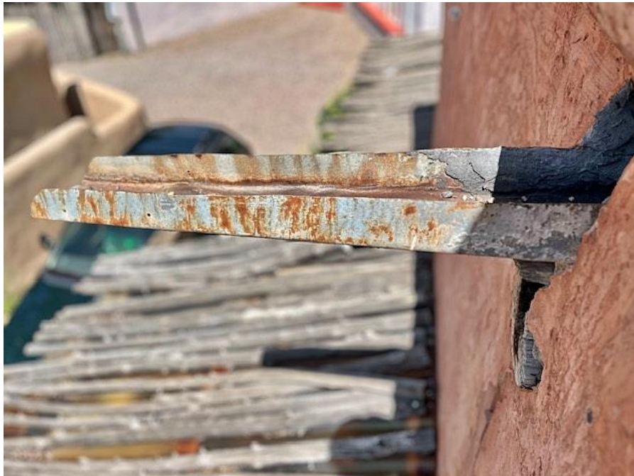
Figure 2: South façade canale, side view.
