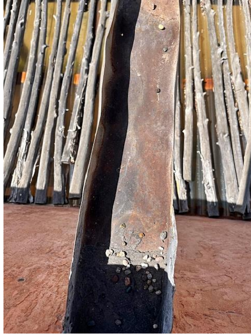
Figure 3: Souh façade canale, down view.
