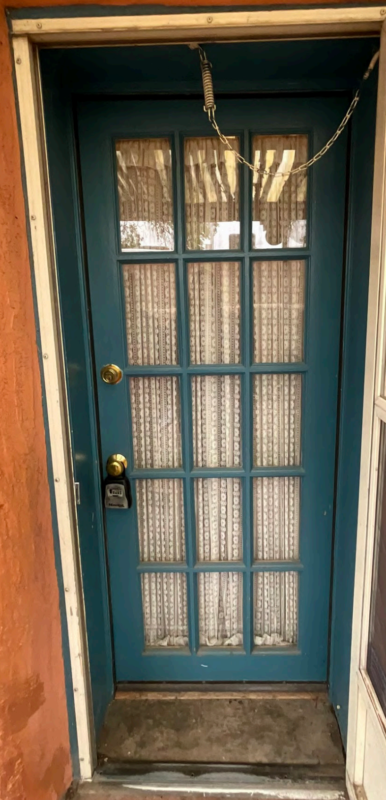
South Elevation Door #2
