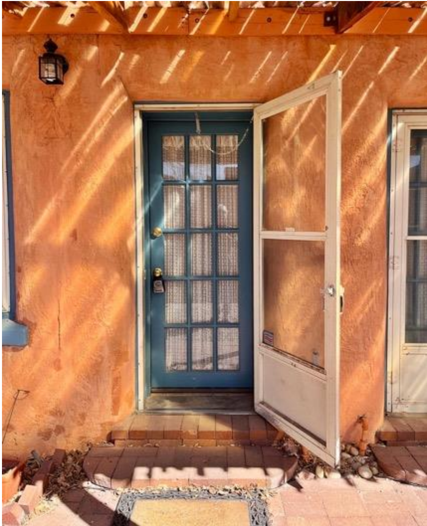
Photo 18: Room 3. West door. Camera facing north.
