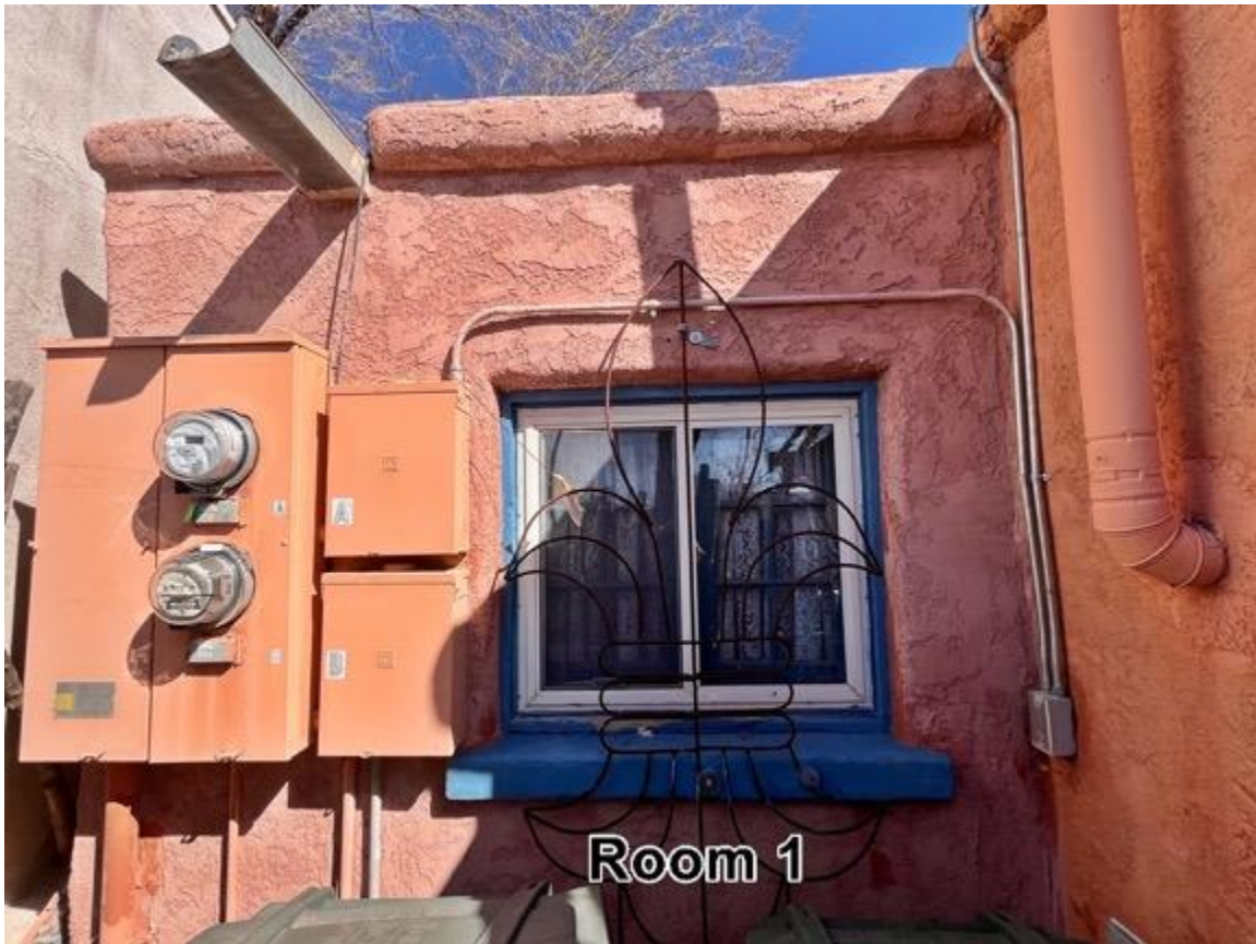
Photo 7: Room 1. Camera facing north.
