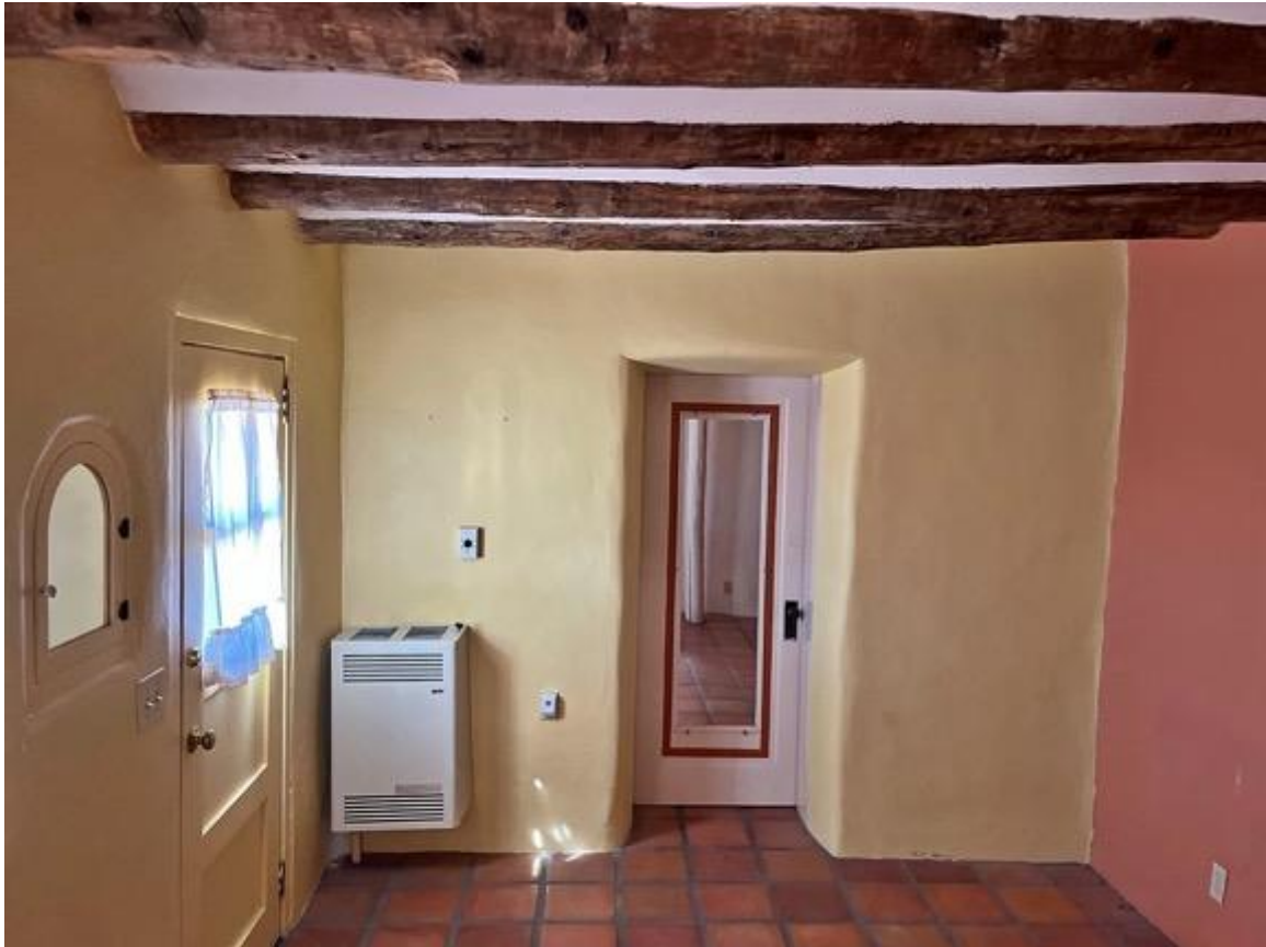
Photo 13: Room 2. Interior. Camera facing west.
