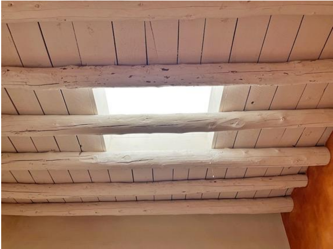
Photo 22: Room 3. Interior ceiling.
