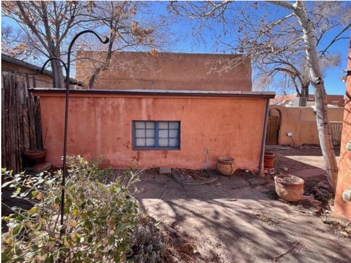
Photo 32: Garage. North elevation. Camera facing south.
