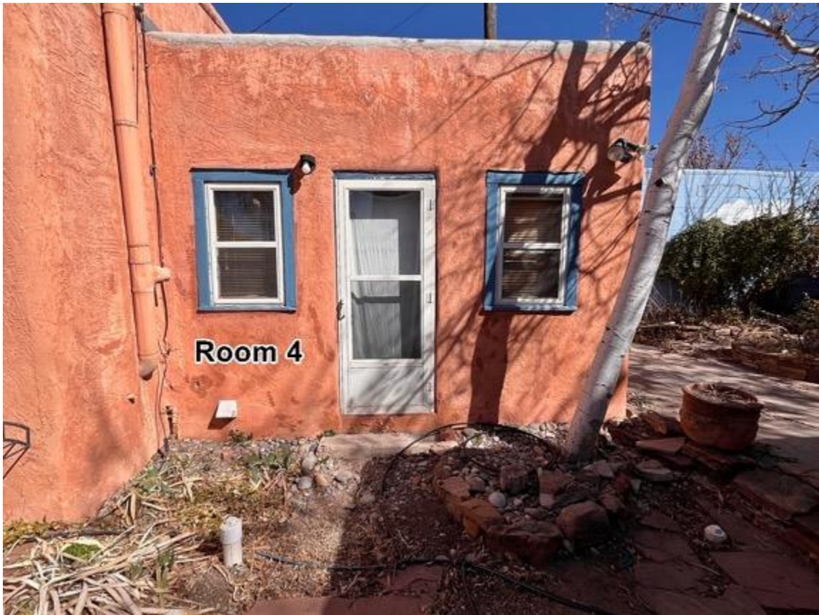
Photo 24: Room 4. Camera facing north.
