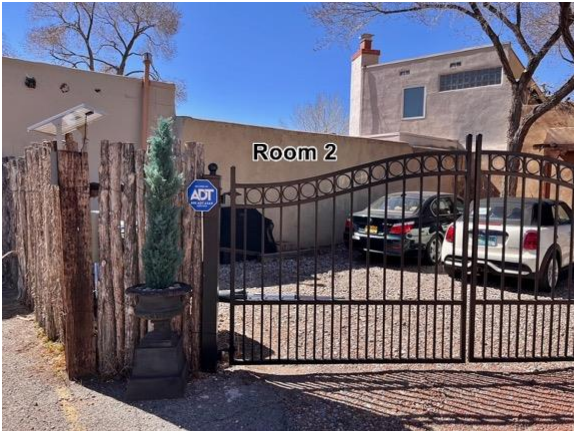
Photo 30: Room 2. North elevation. Camera facing southwest.
