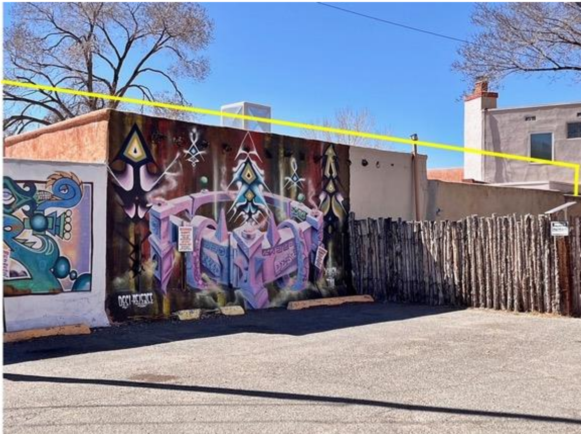
Photo 28: Subject building. North elevation at North Guadalupe Street parking lot. Camera facing southwest.
