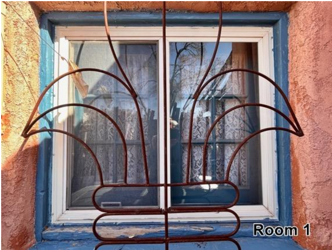
Photo 8: Room 1. Window. Camera facing north.
