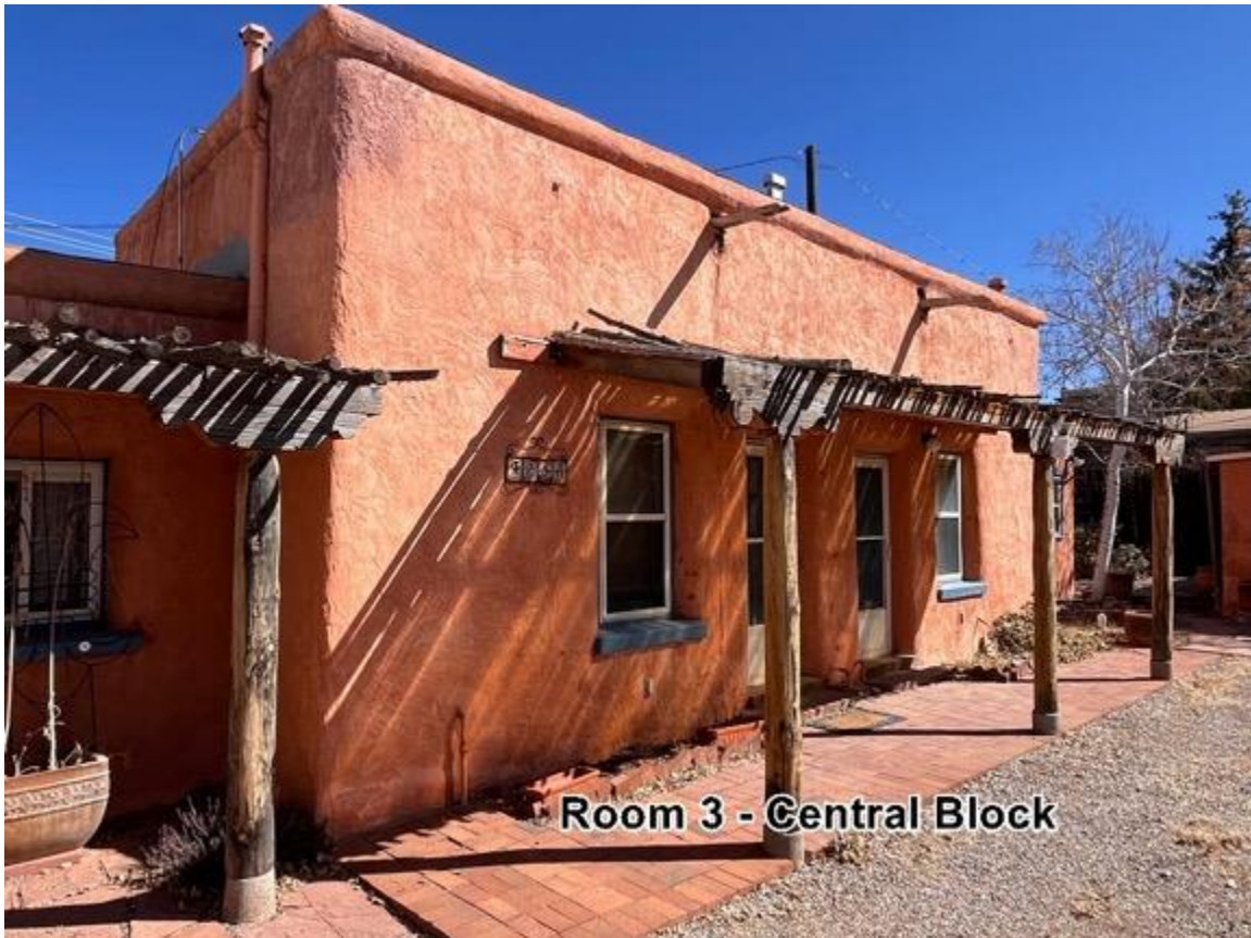
Photo 15: Room 3 (Central Block). Camera facing northeast.
