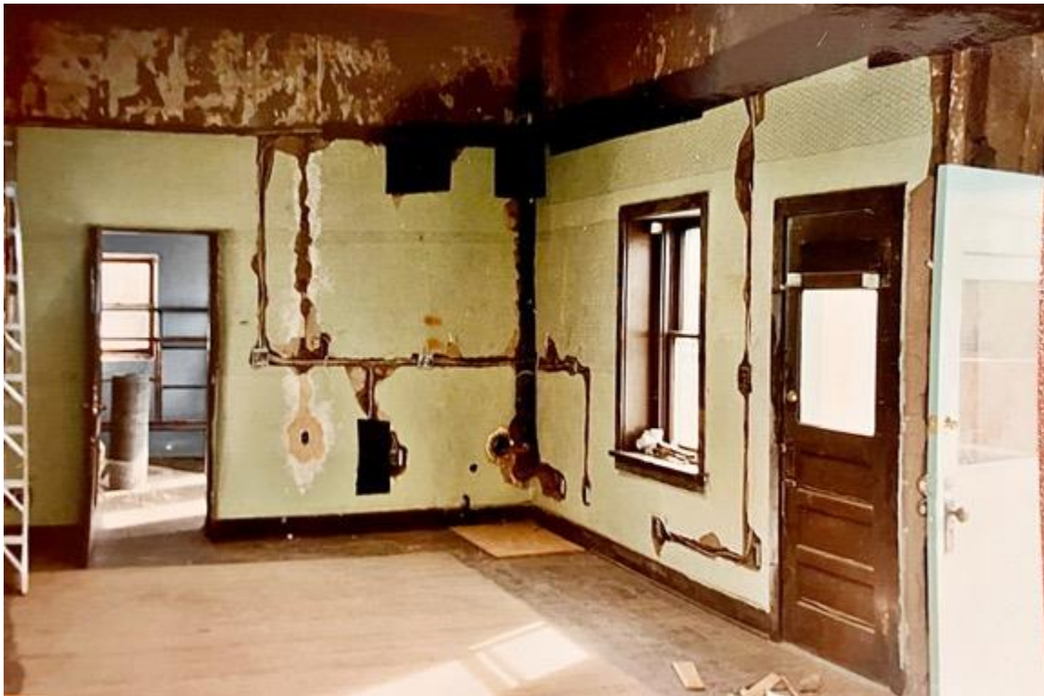
Photo 21: Room 3. 1990s renovation photograph. Camera facing southeast. Note conduit cuts in the adobe walls, removal of ceiling, and older window and door. Courtesy of Heidi Cost.
