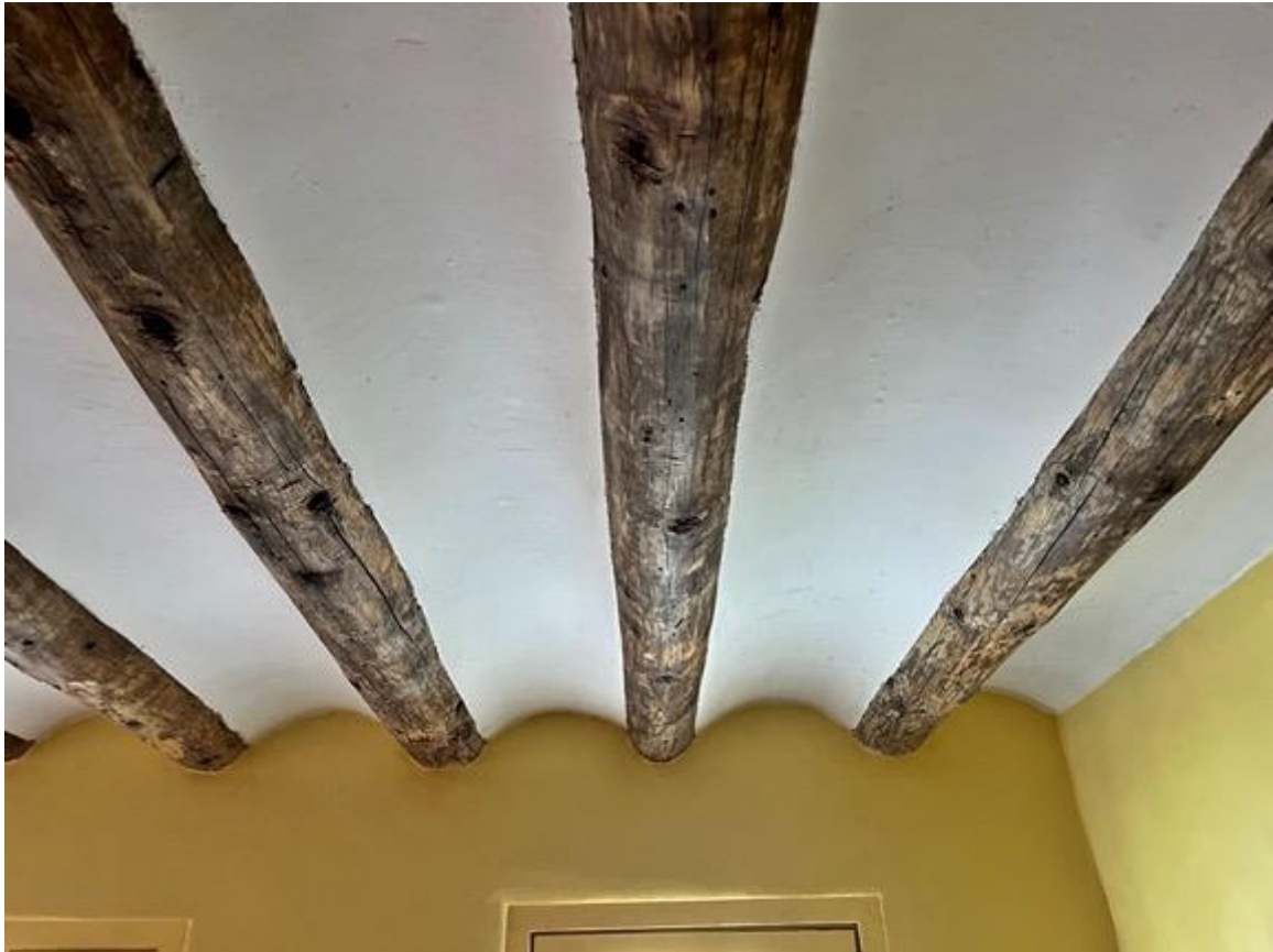
Photo 14: Room 2. Interior, ceiling.
