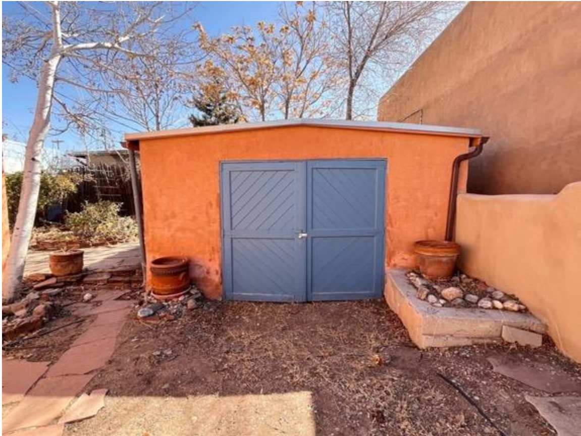
Photo 31: Garage. West elevation. Camera facing east.
