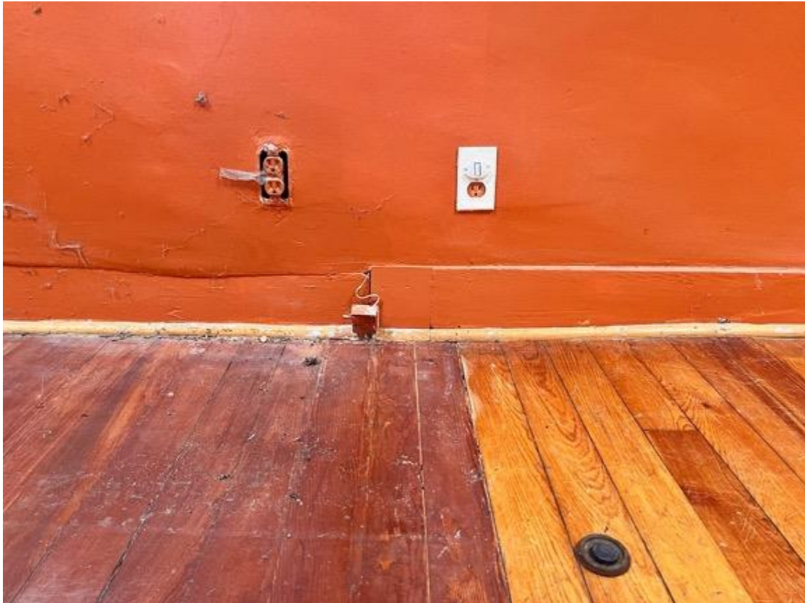
Photo 23: Room 3. Interior, change of floor coloring and shoe molding.
