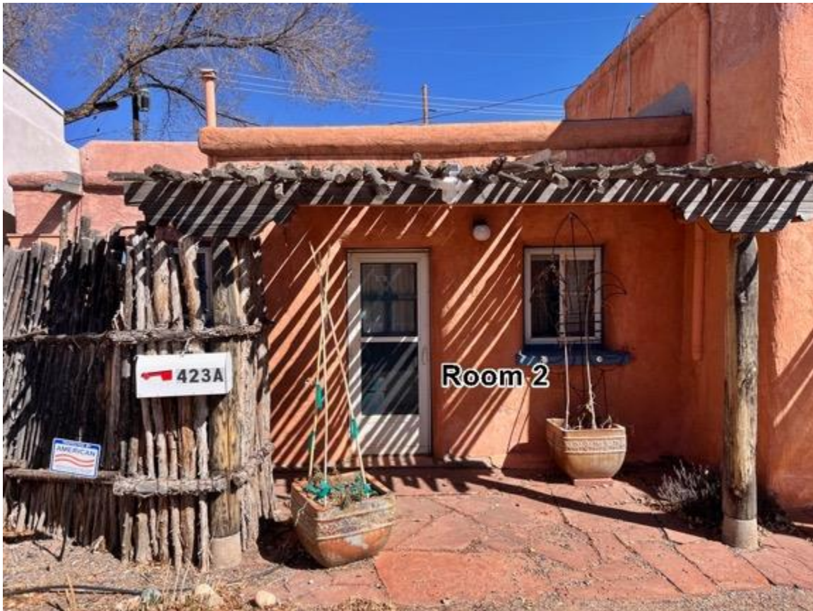
Photo 10: Room 2. Camera facing north.
