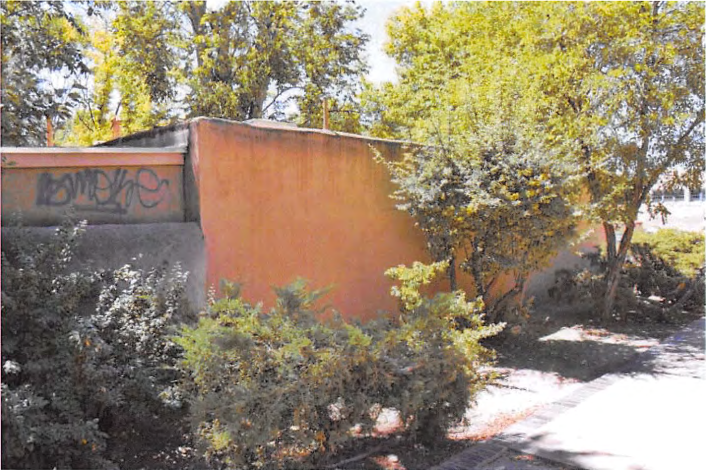
Photo 3: North elevation, concrete walkway at right corner. Camera facing southwest.
