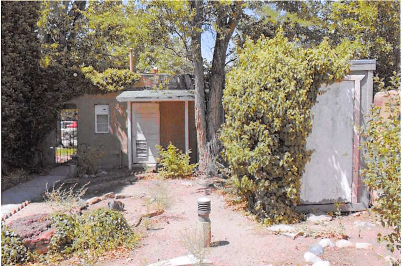
Photo 4: East elevation, shed addition in foreground. Camera facing west.
