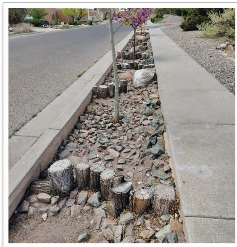
Figure 73: Check Dams Made from Wood
