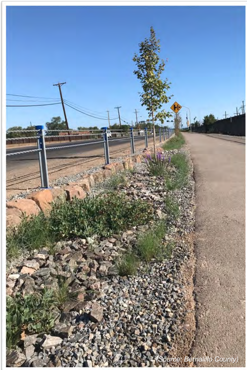
Figure 63: Bioretention Basin Constructed Along 2nd Street Trail
