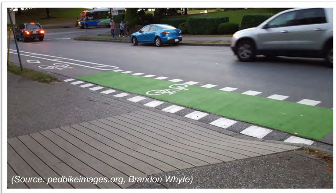
Figure 22: Raised Bike Lane
