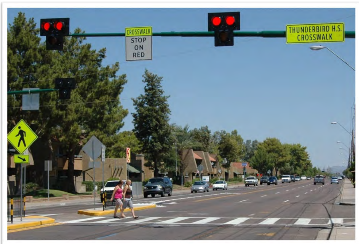
Figure 41: HAWK Beacon and Crossing
