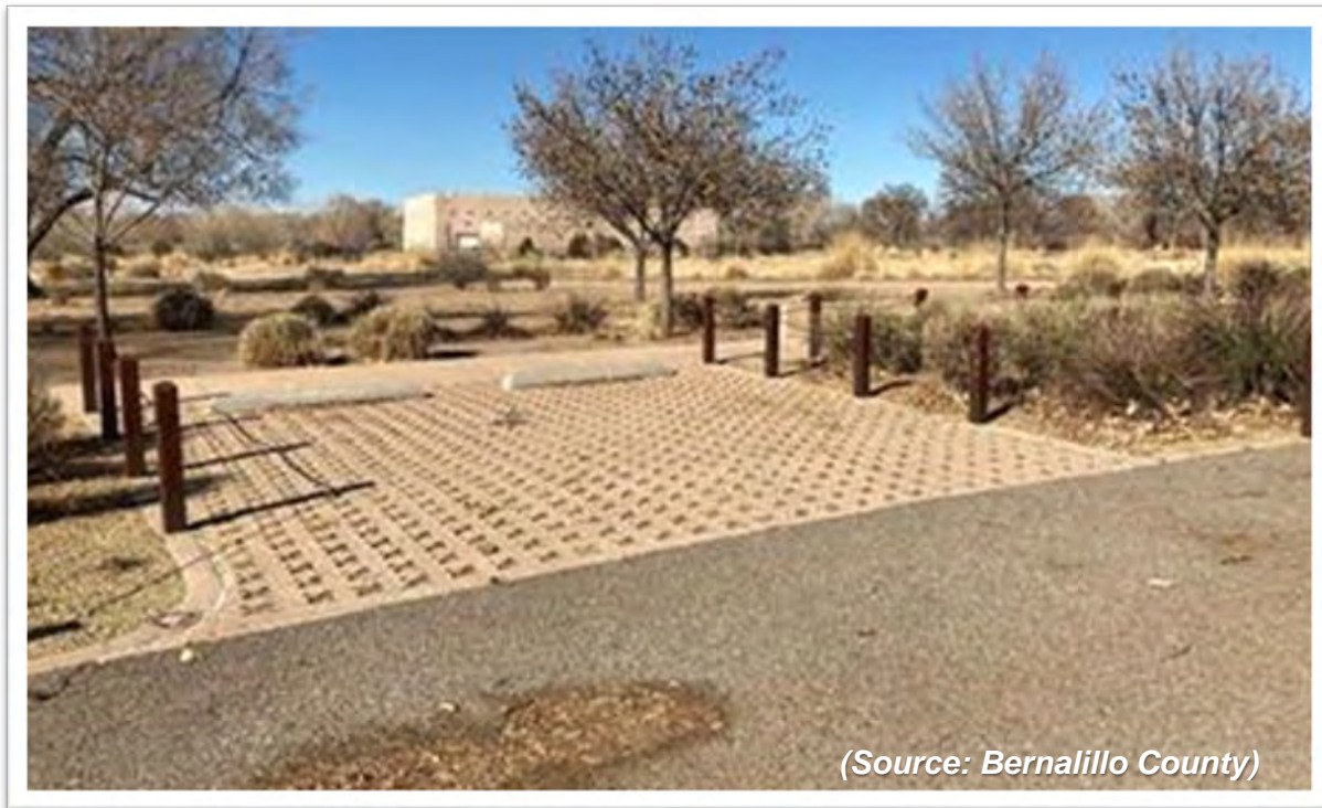
Figure 67: Permeable Pavers at Bachechi Open Space in Albuquerque
