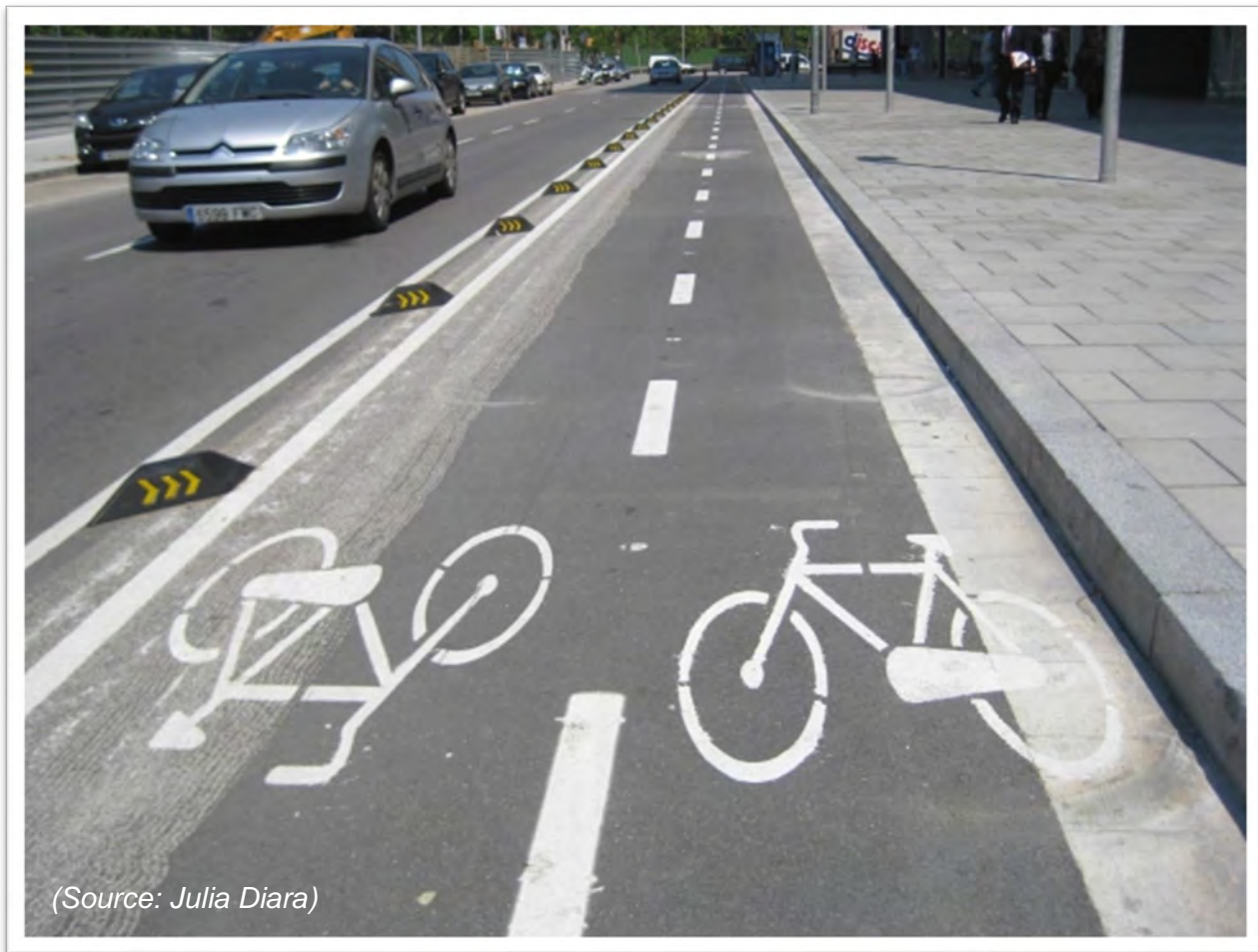
Figure 24: Rubber Barriers on a Two-Way Cycle Track
