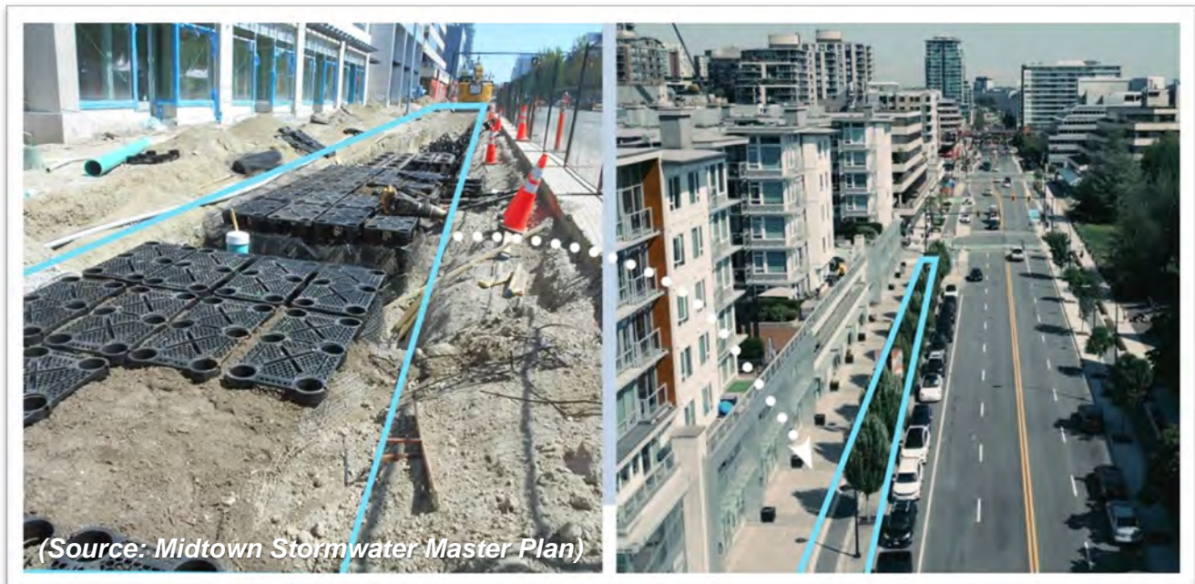
Figure 69: Narrow Streetscape Planters Using Suspended Pavement Can Facilitate Successful Inclusion of Trees
