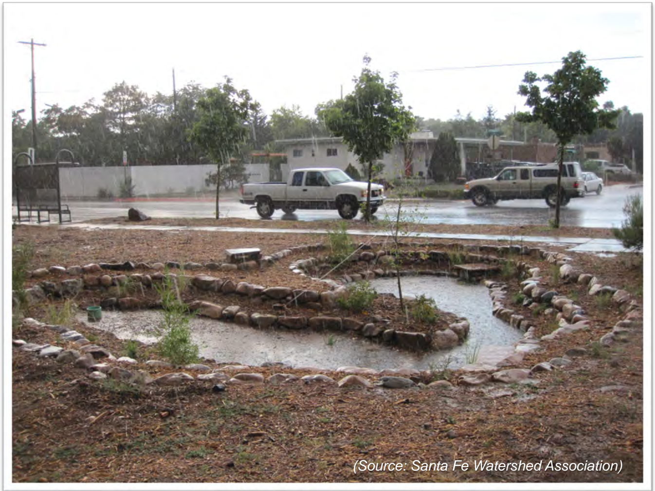
Figure 64: Bioretention Basin, also known as a Rain Garden, along West Alameda in Santa Fe
