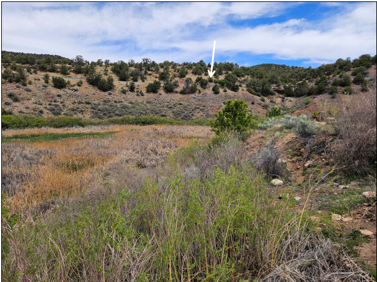
Figure 7. View to the north of the outcrop along the north side of the pond. Fault is situated nearly parallel to the metal retaining wall (arrow points to retaining wall).
