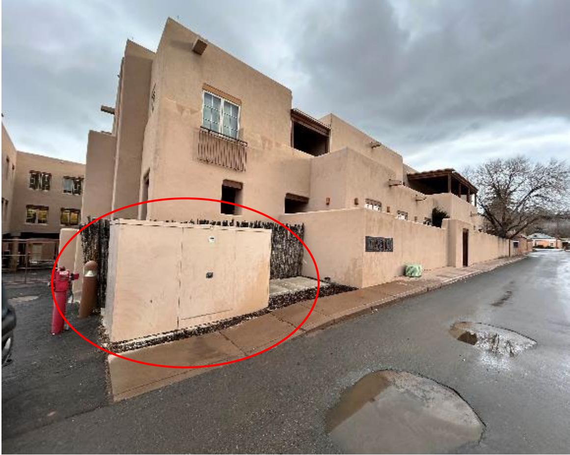
El Castillo Life Plan Community fire service Hot Box painted to match stucco of building
