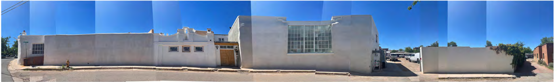
206 McKenzie Street McKenzie Street / North Elevation
