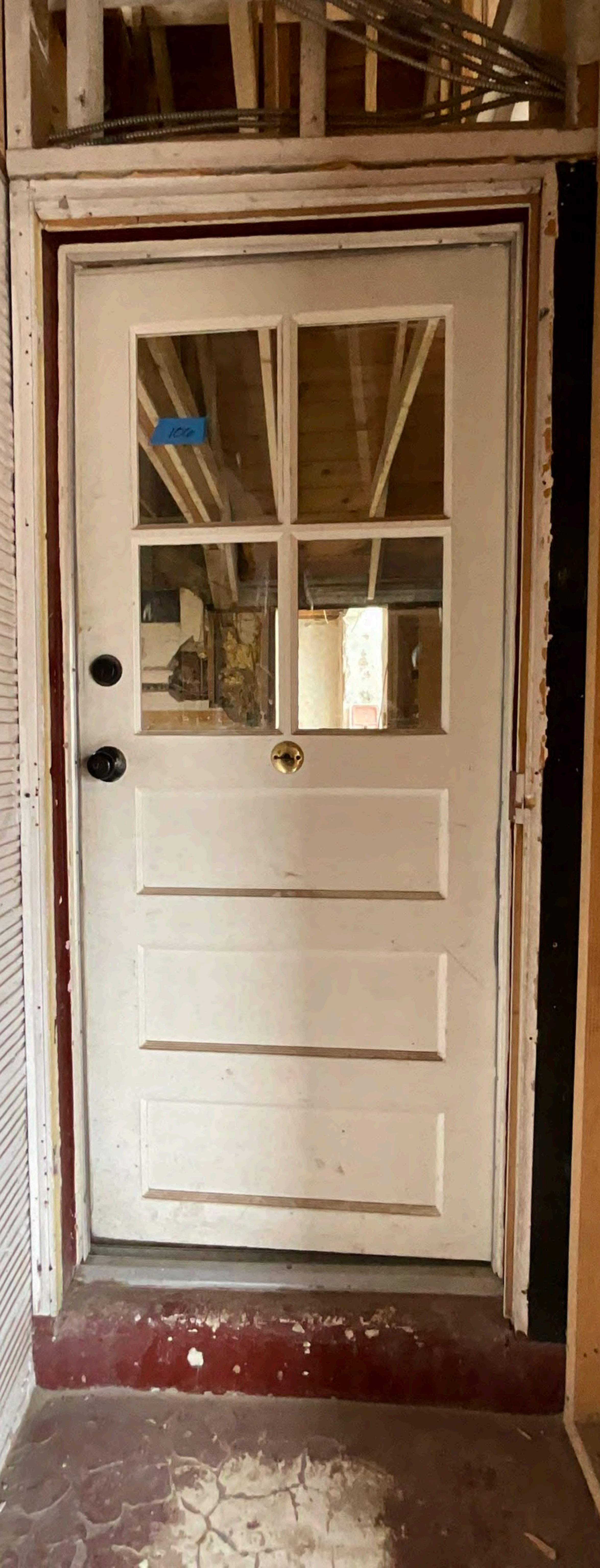
West Elevation Door #3
