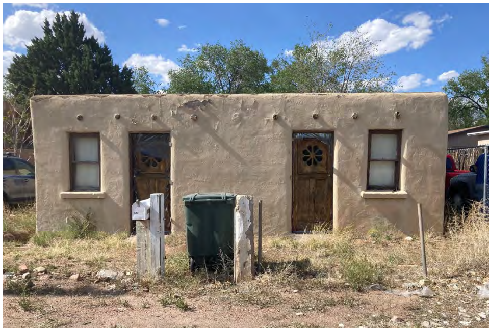
South façade – looking north – May 2025
