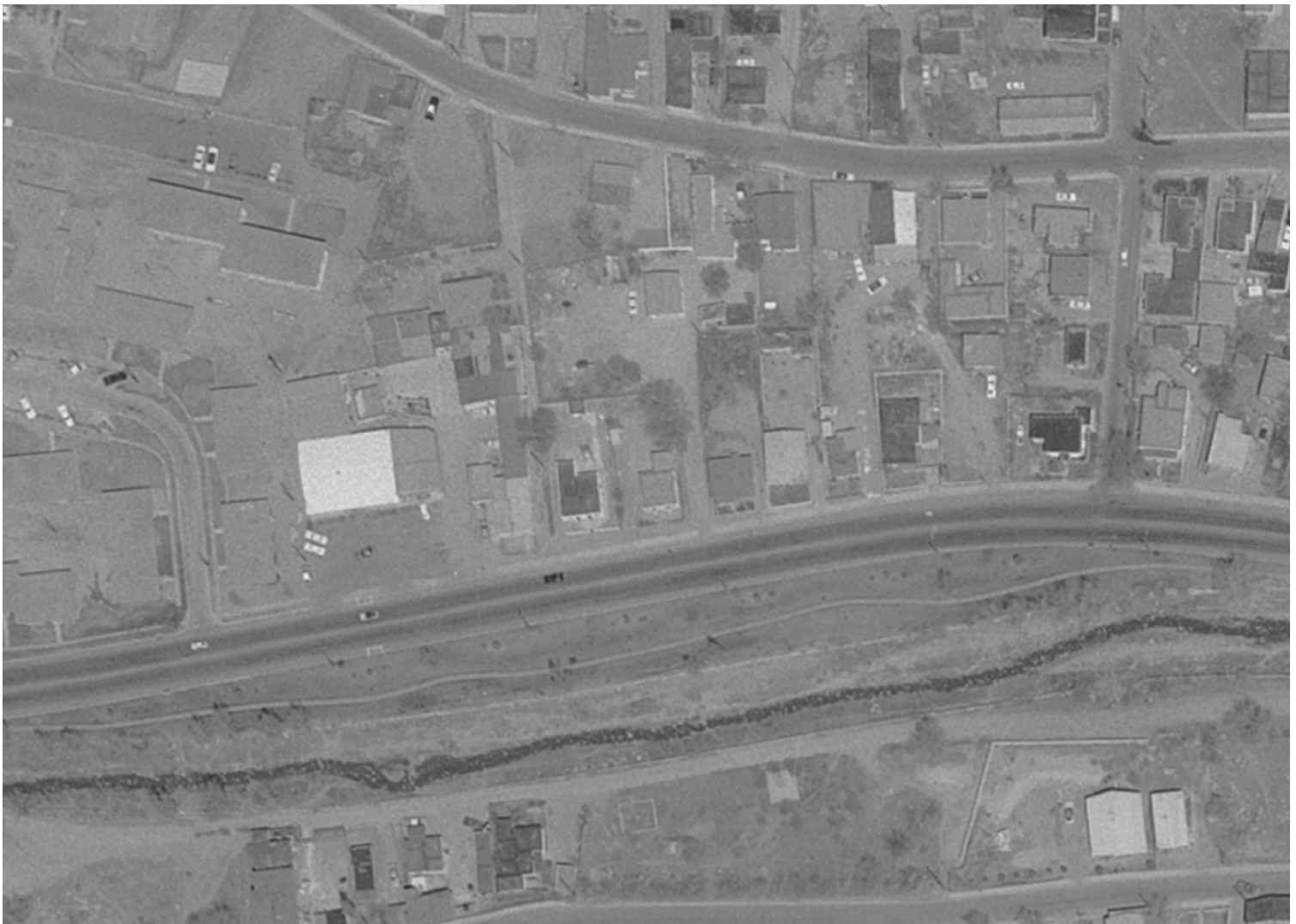
Aerial view – 1975 – clearly shows the third addition
