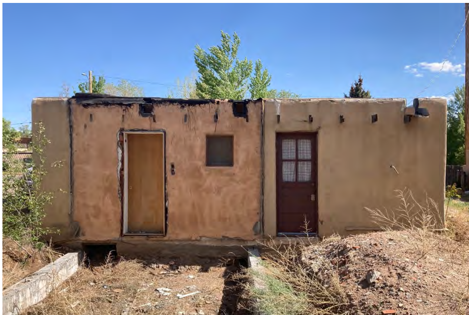
North façade – looking south – May 2025
