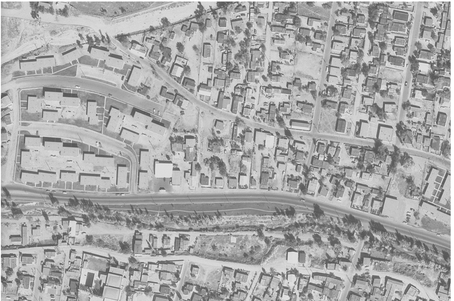
Aerial view - 1967 - clearly shows a square building
