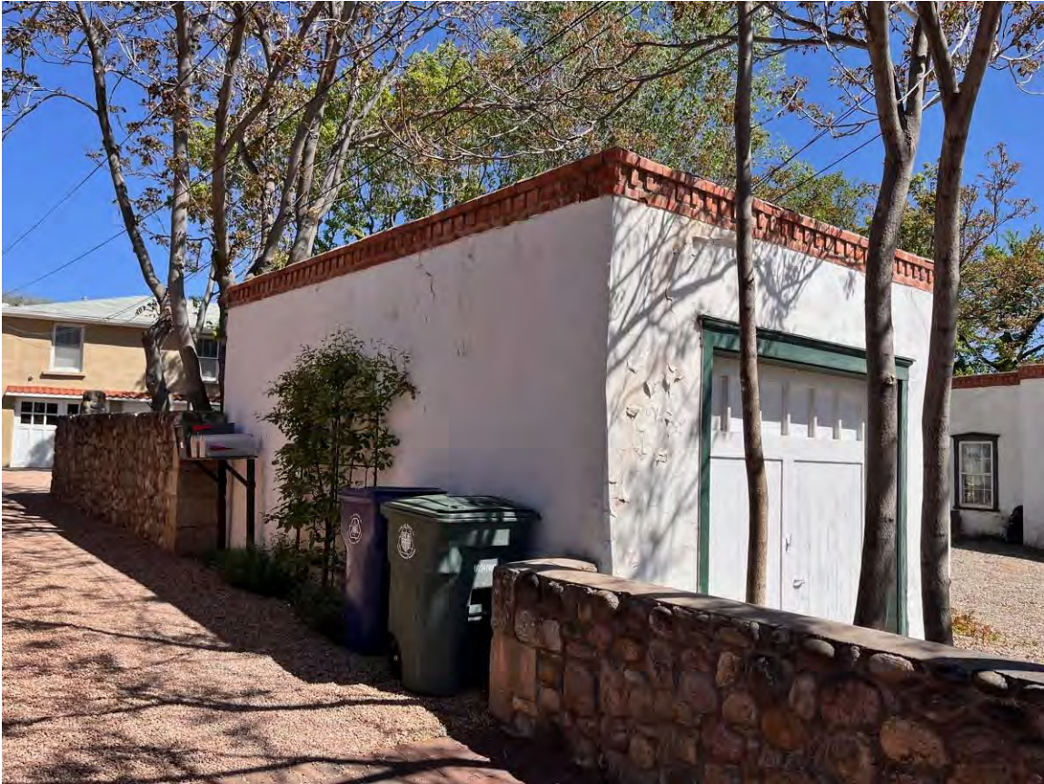
Photo 23: Garage. North elevation and cobblestone property wall. Camera facing southeast.
