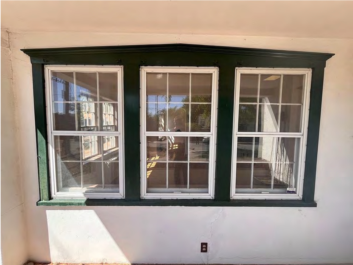
Photo 5: South (front) elevation. Porch section. Grouped windows. Camera facing north.
