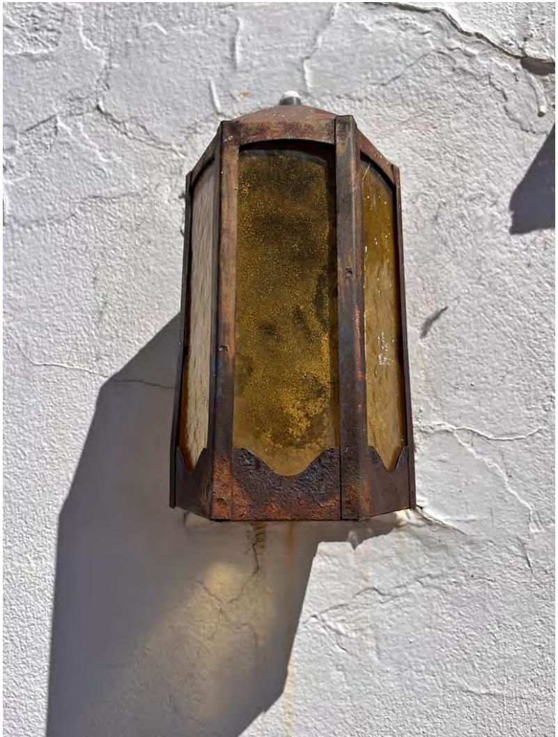
Photo 13: West elevation. Wall sconce. Camera facing east.
