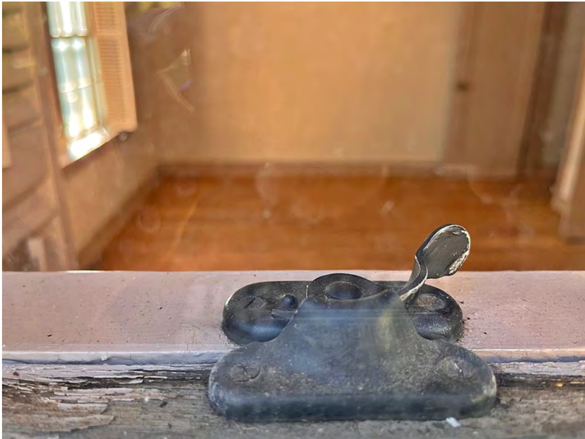
Photo 7: Window detail of sash lock.
