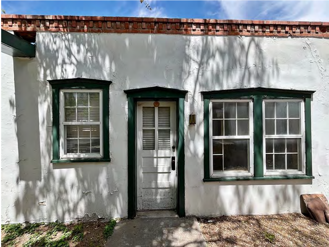
Photo 18: East elevation. Windows and doors. Camera facing west.
