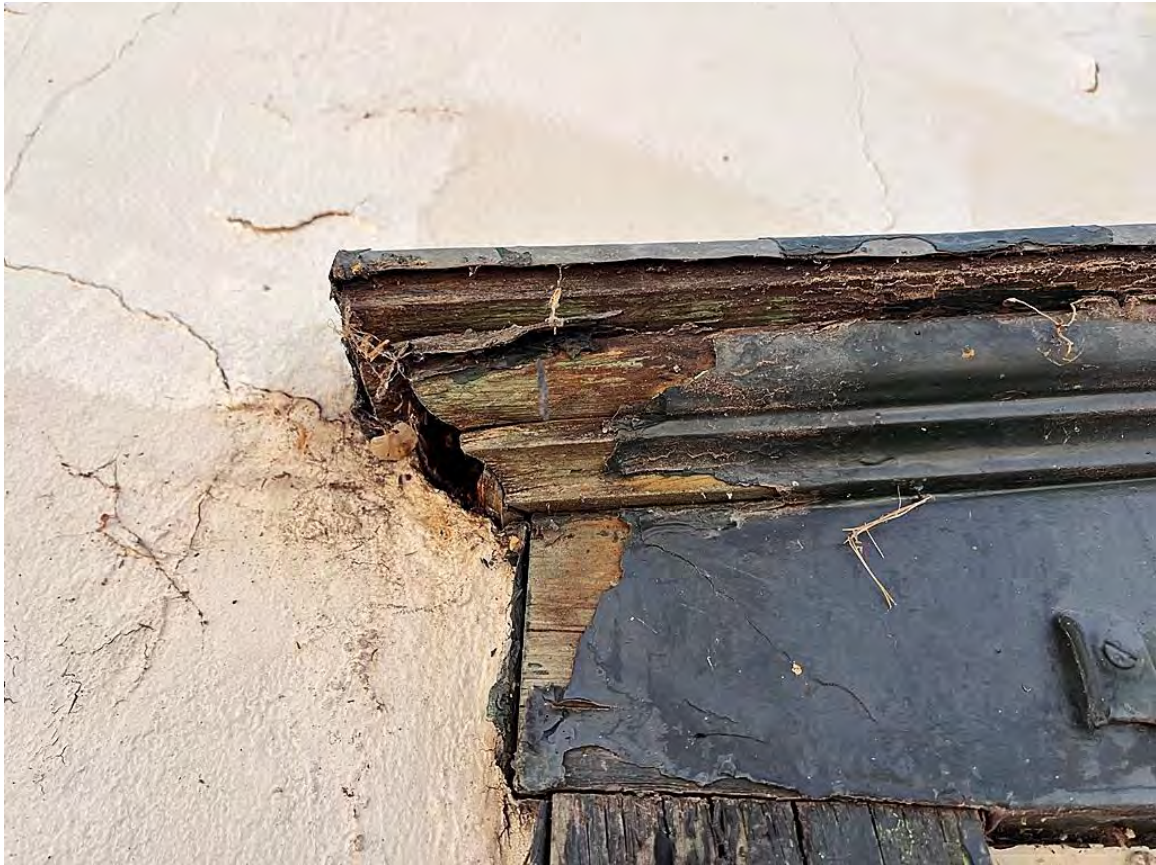
Photo 8: Window detail of pedimented head.
