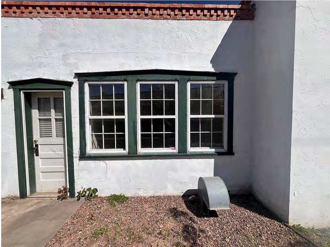
Photo 12: West elevation. Windows and doors. Camera facing east.
