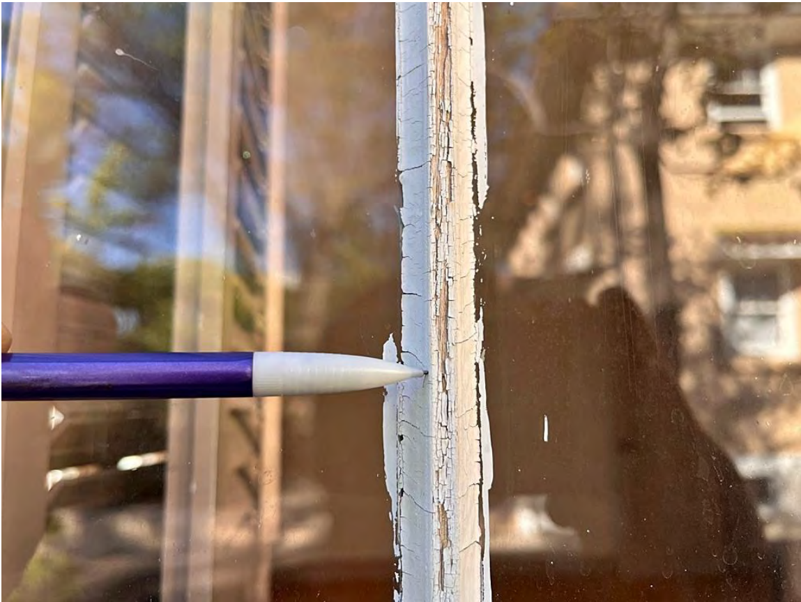
Photo 6: Window detail of 1/8" muntin profile tip.
