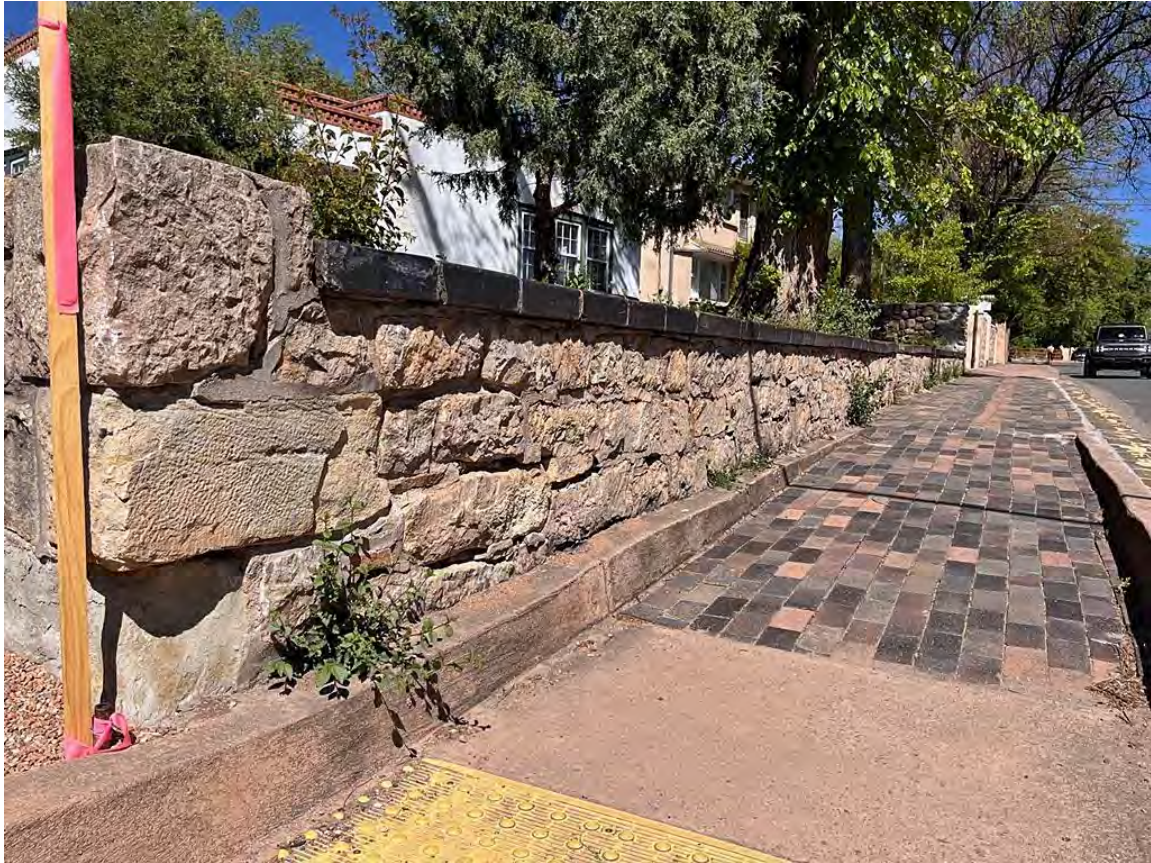
Photo 24: South (front) retaining wall. Camera facing northeast.
