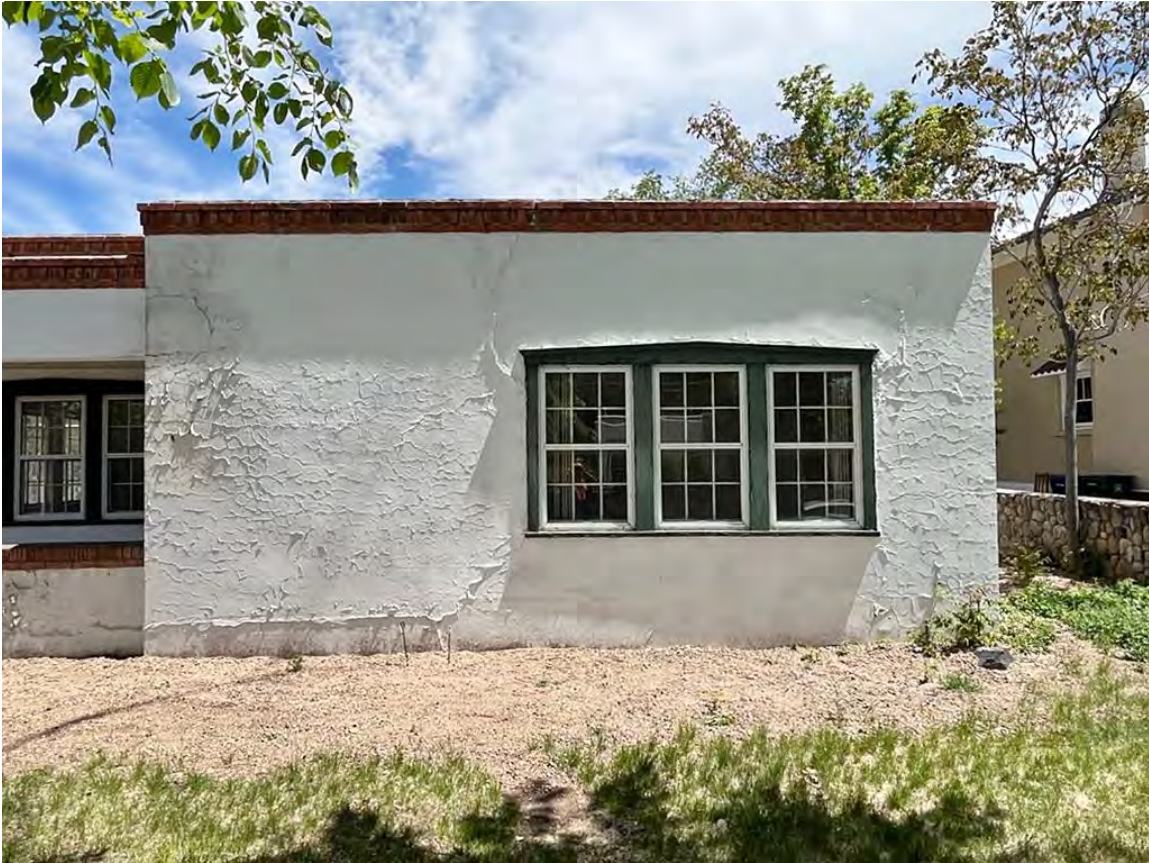
Photo 10: South (front) elevation. East section. Camera facing north.
