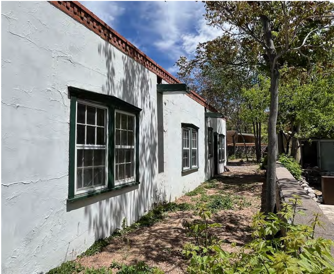
Photo 17: East elevation. Camera facing north.
