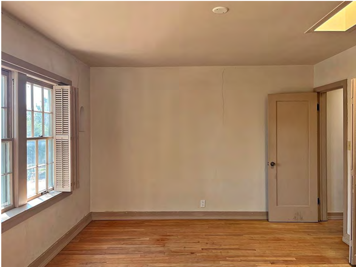
Photo 21: Former bedroom. Camera facing south.
