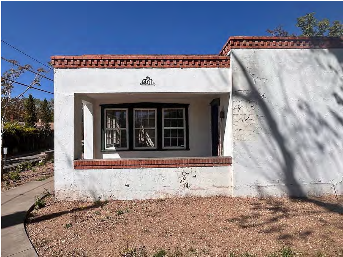
Photo 3: South (front) elevation. Porch section. Camera facing north.
