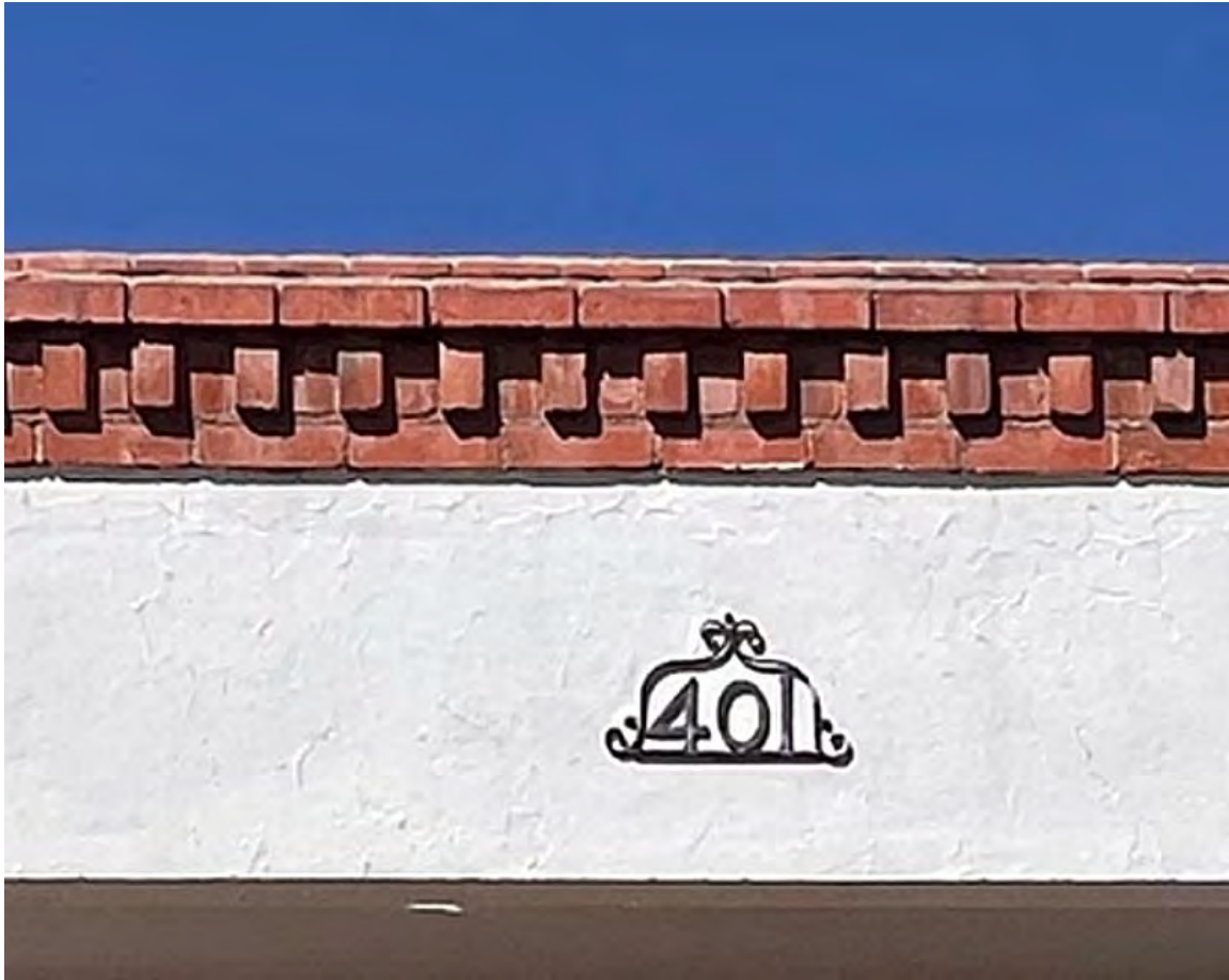
Photo 9: Detail of brick coping pattern.
