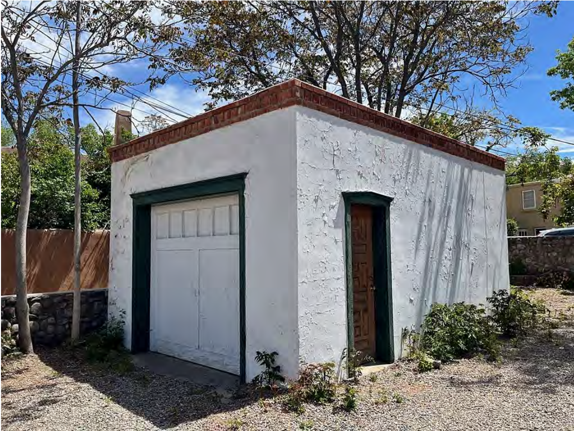
Photo 22: Garage. West and south elevations. Camera facing north.
