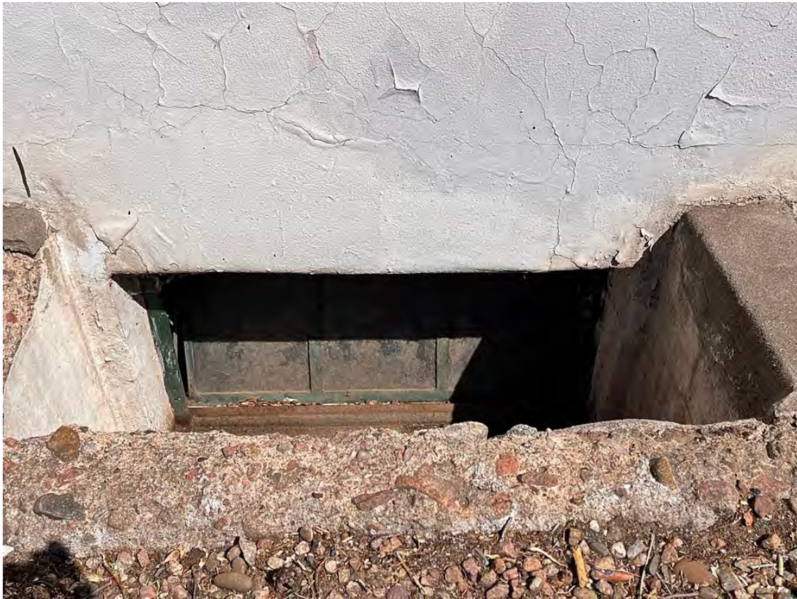
Photo 14: West elevation. Basement window.
