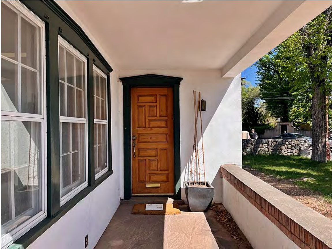
Photo 4: South (front) elevation. Porch section. Camera facing east.
