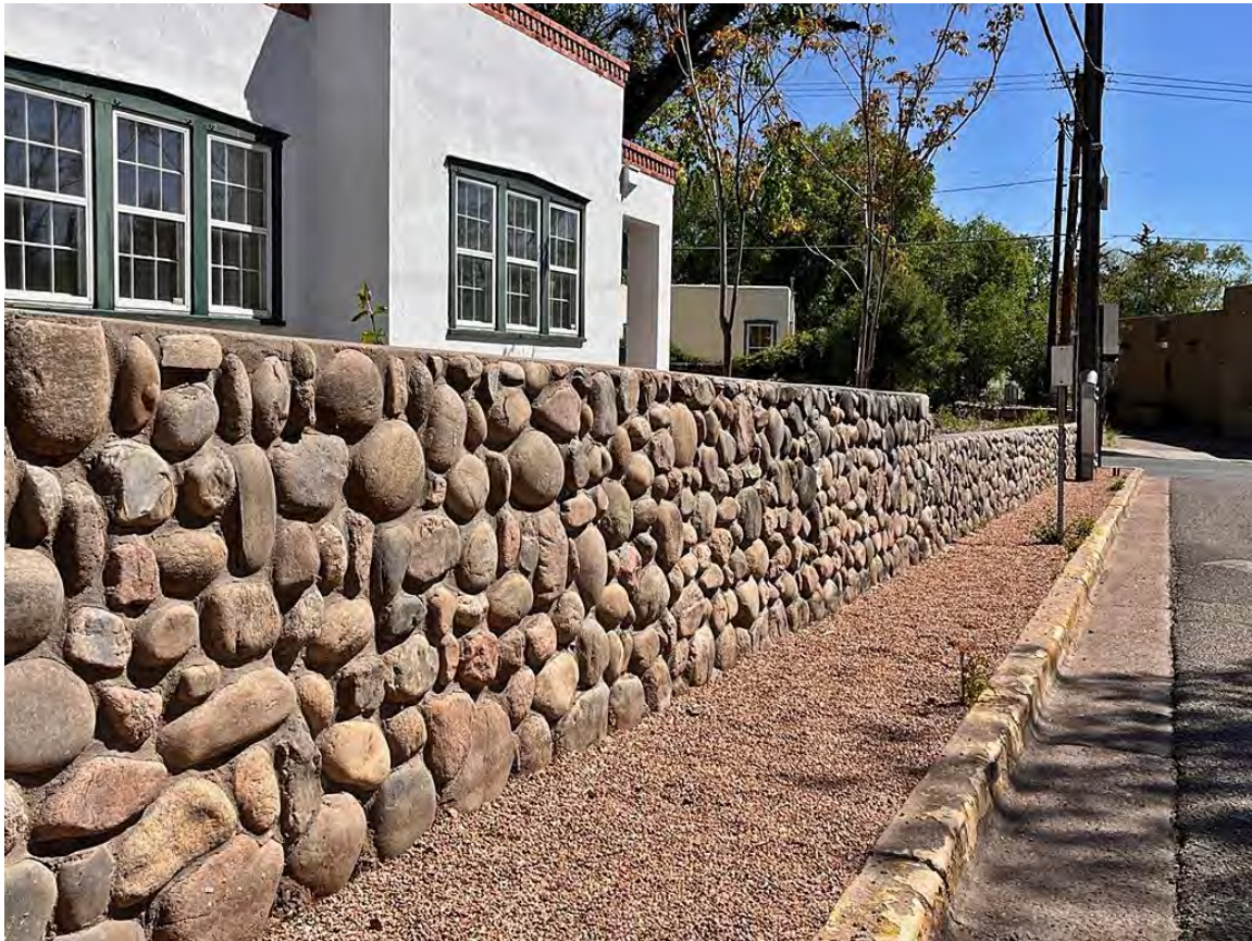
Photo 26: West retaining wall. Camera facing southeast.
