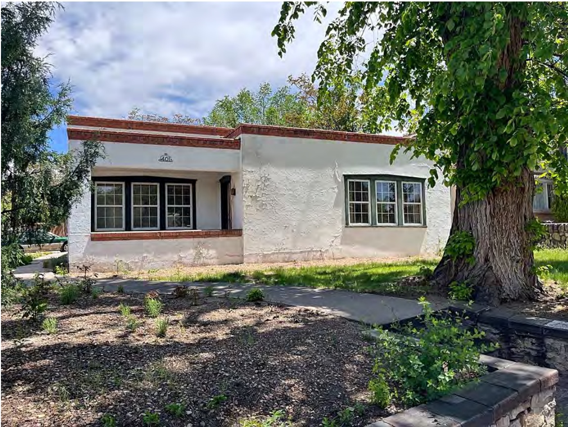
Photo 2: South (front) elevation. Camera facing northeast.
