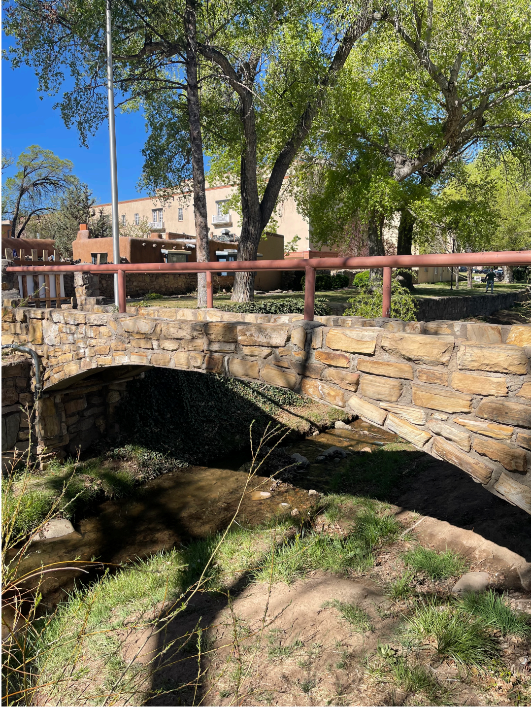
Figure 3. Shelby Street Footbridge, east elevation, view west/southwest.
