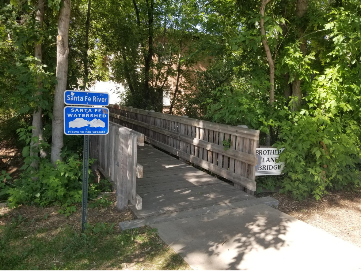
Figure 5. Bridge Style 2, wooden rails with tight spacing between the pickets and a wooden deck.
