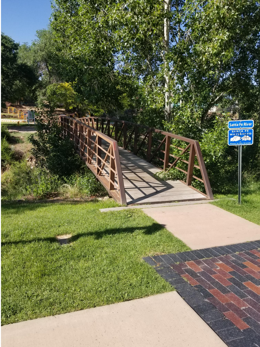
Figure 6. Bridge Style 3, metal prefab bridge with wood decking.
