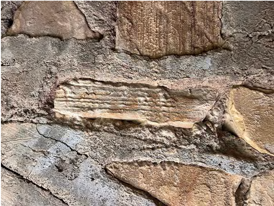
Photo 5: Interior stonework of false spandrel wall.
