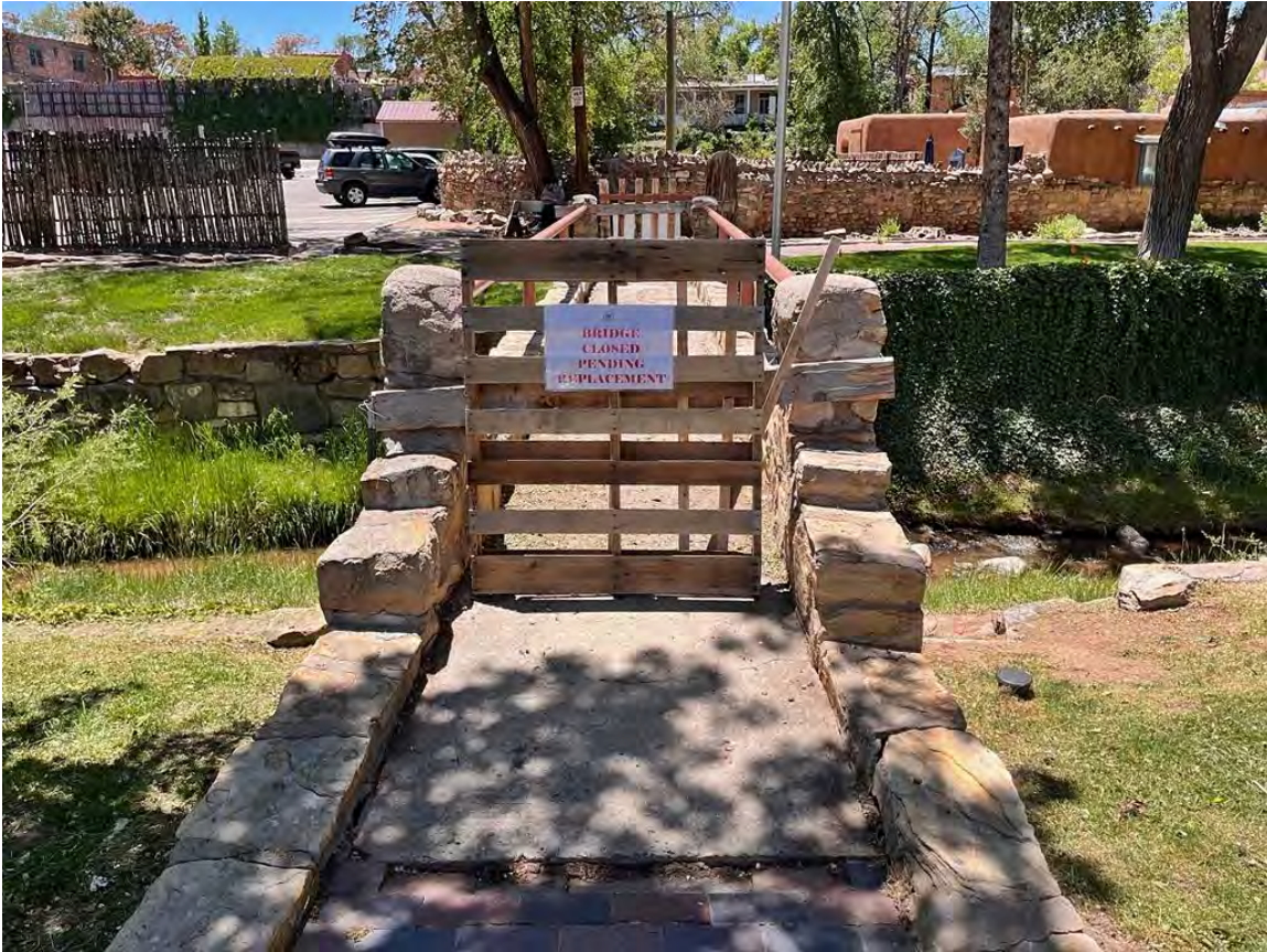
Photo 10: North approach. Camera facing south.
