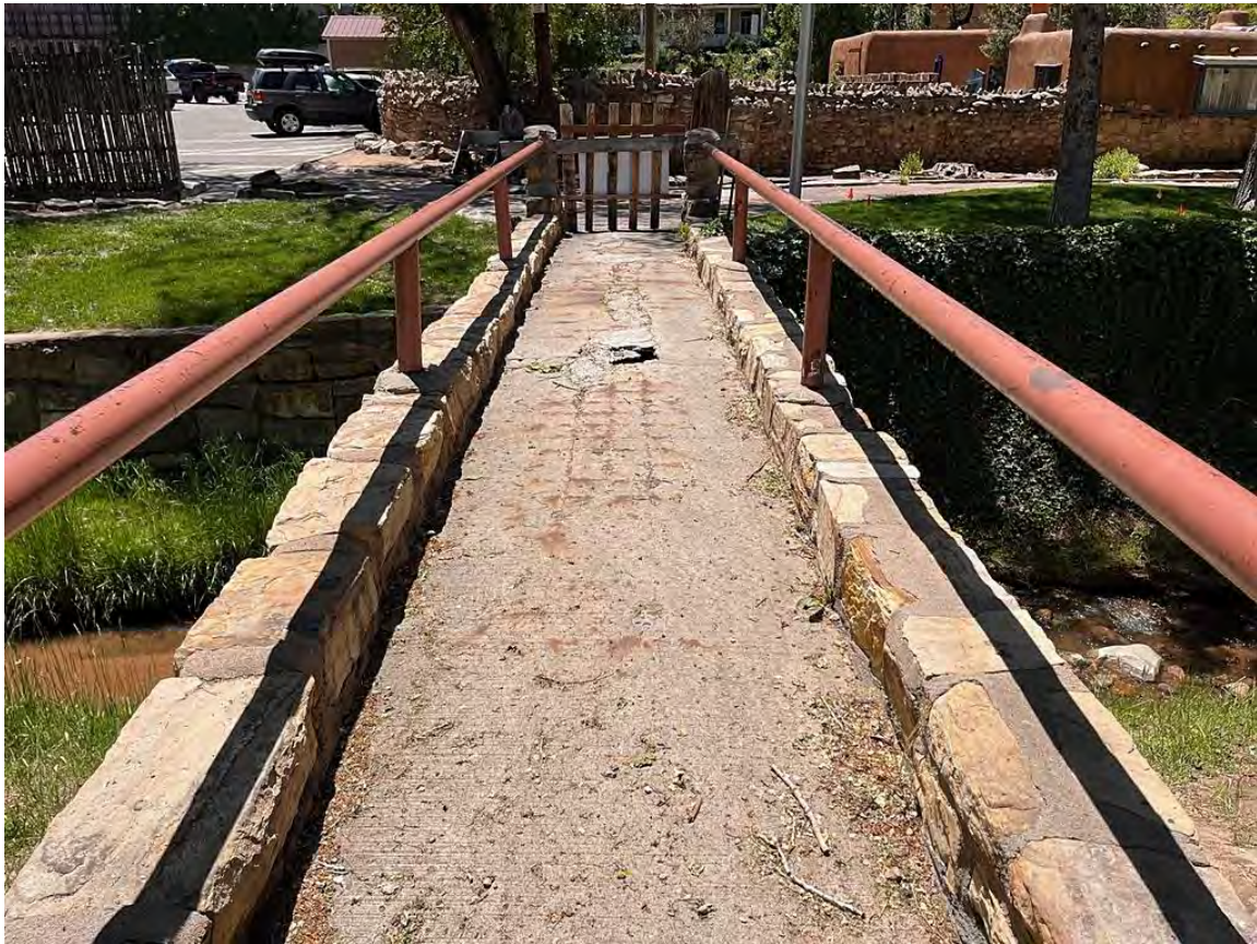
Photo 9: Deck and railing. Camera facing south.
