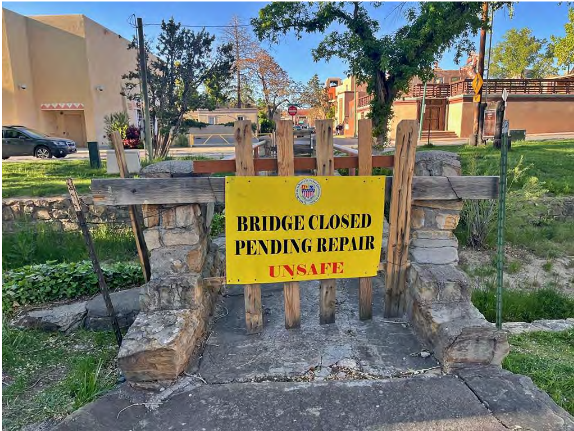
Photo 2: South approach. Camera facing north.
