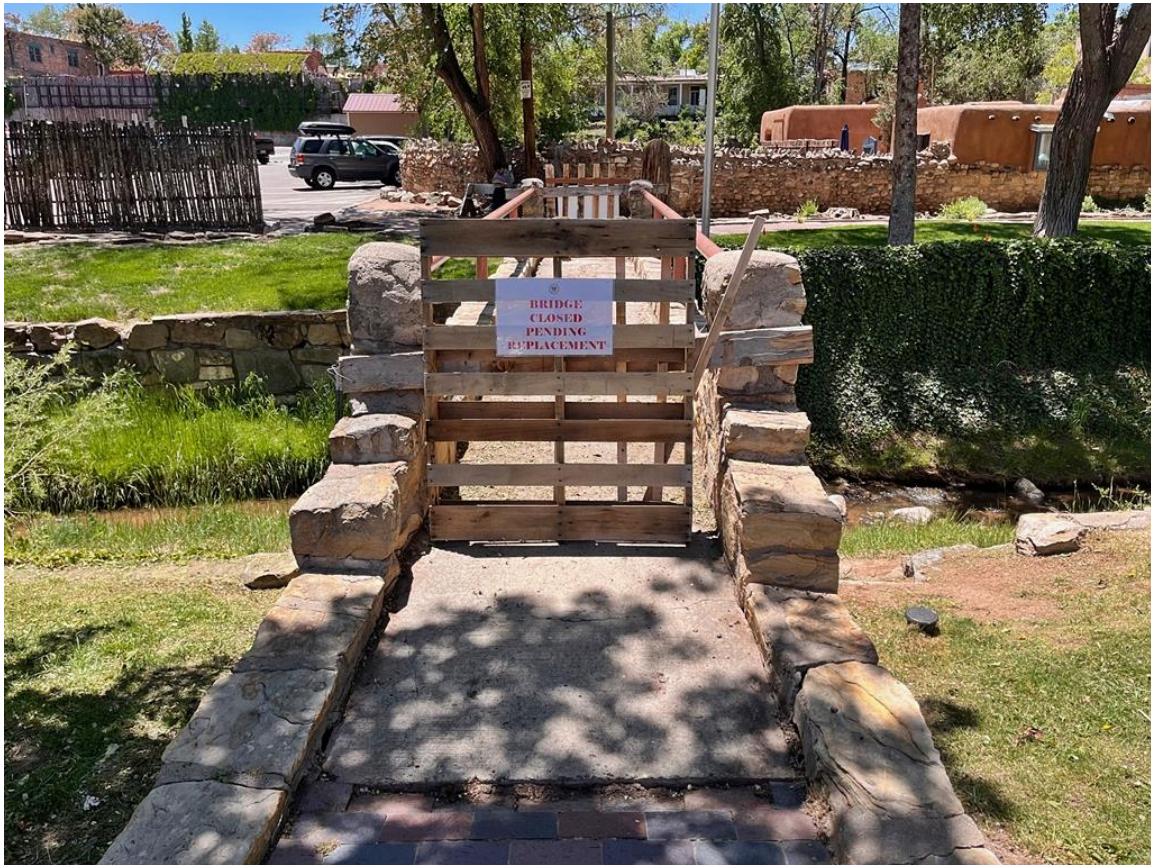
Photo 10: North approach. Camera facing south.
