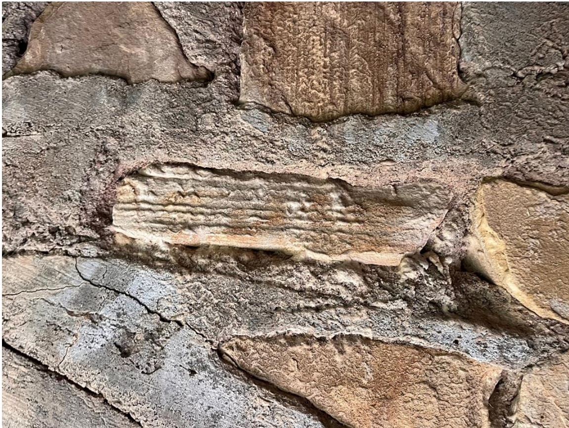
Photo 5: Interior stonework of false spandrel wall.
