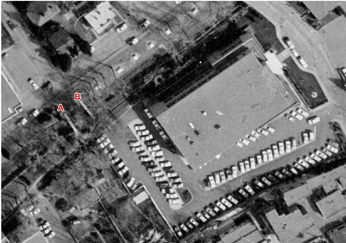
Figure 5: February 2, 1968, aerial photograph showing two bridges at the Shelby Street crossing. A. is the bridge erected 1968; B. is likely the CCC -constructed built in 1934.
