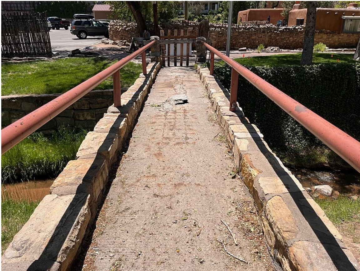
Photo 9: Deck and railing. Camera facing south.
