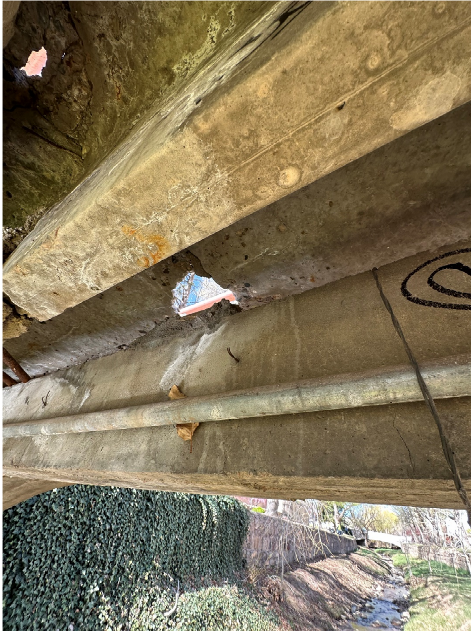
Figure 5 – Underside of flange damage
