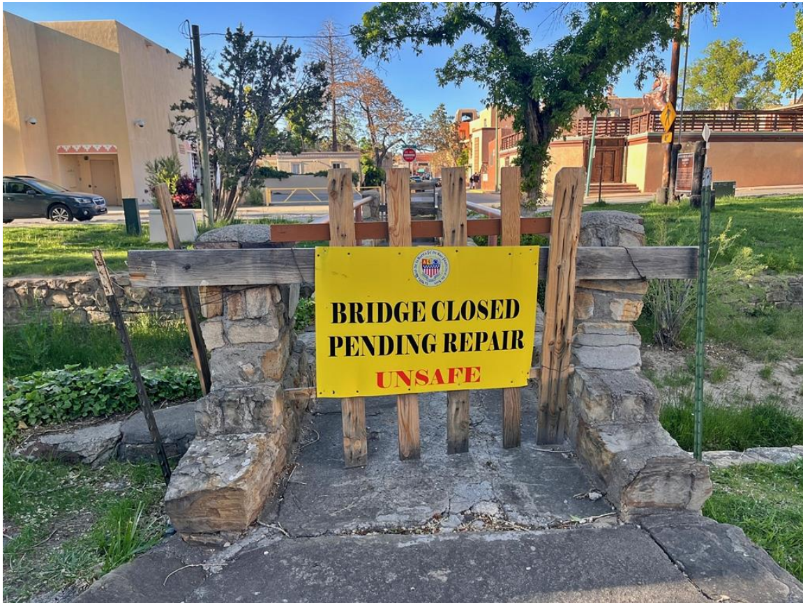
Photo 2: South approach. Camera facing north.
