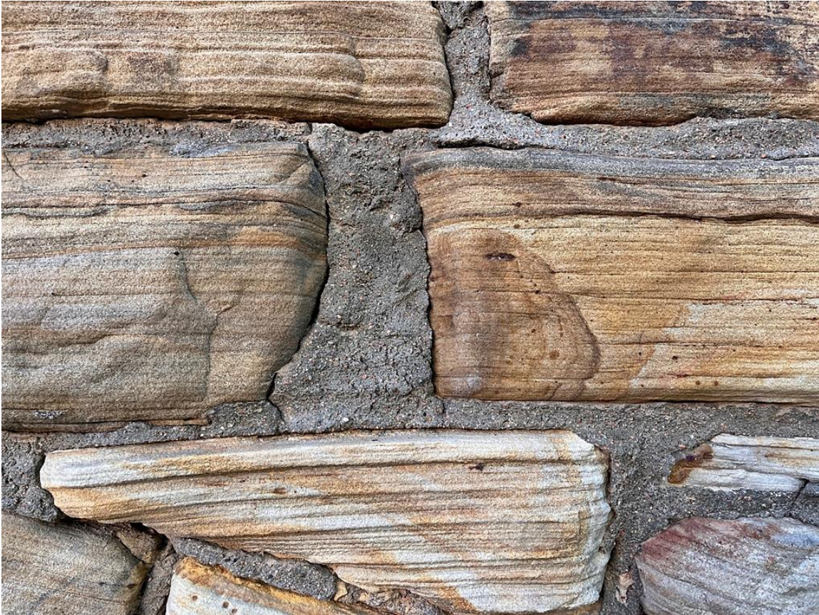
Photo 6: Exterior stonework of false spandrel wall.
