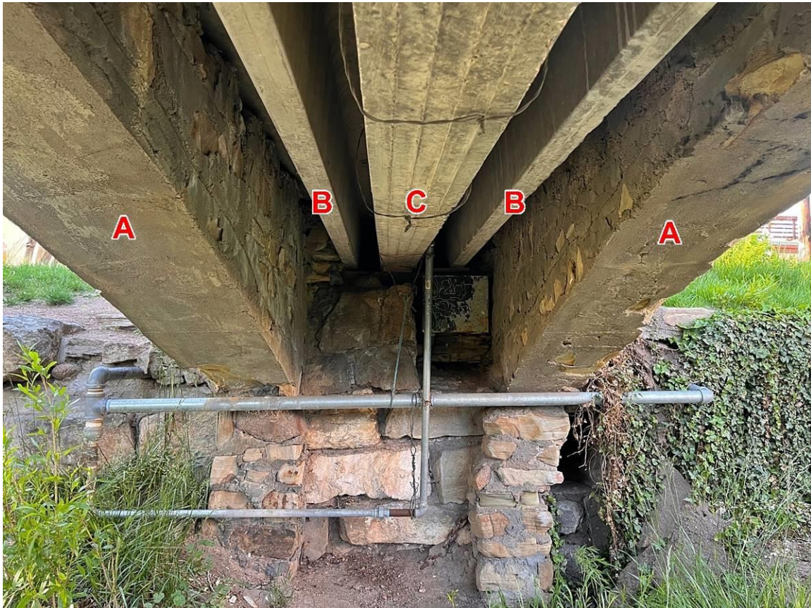
Photo 4: Bridge superstructure: A: exterior false spandrel walls, B. girder-slab beams C. reinforced center beam. Camera facing north.
