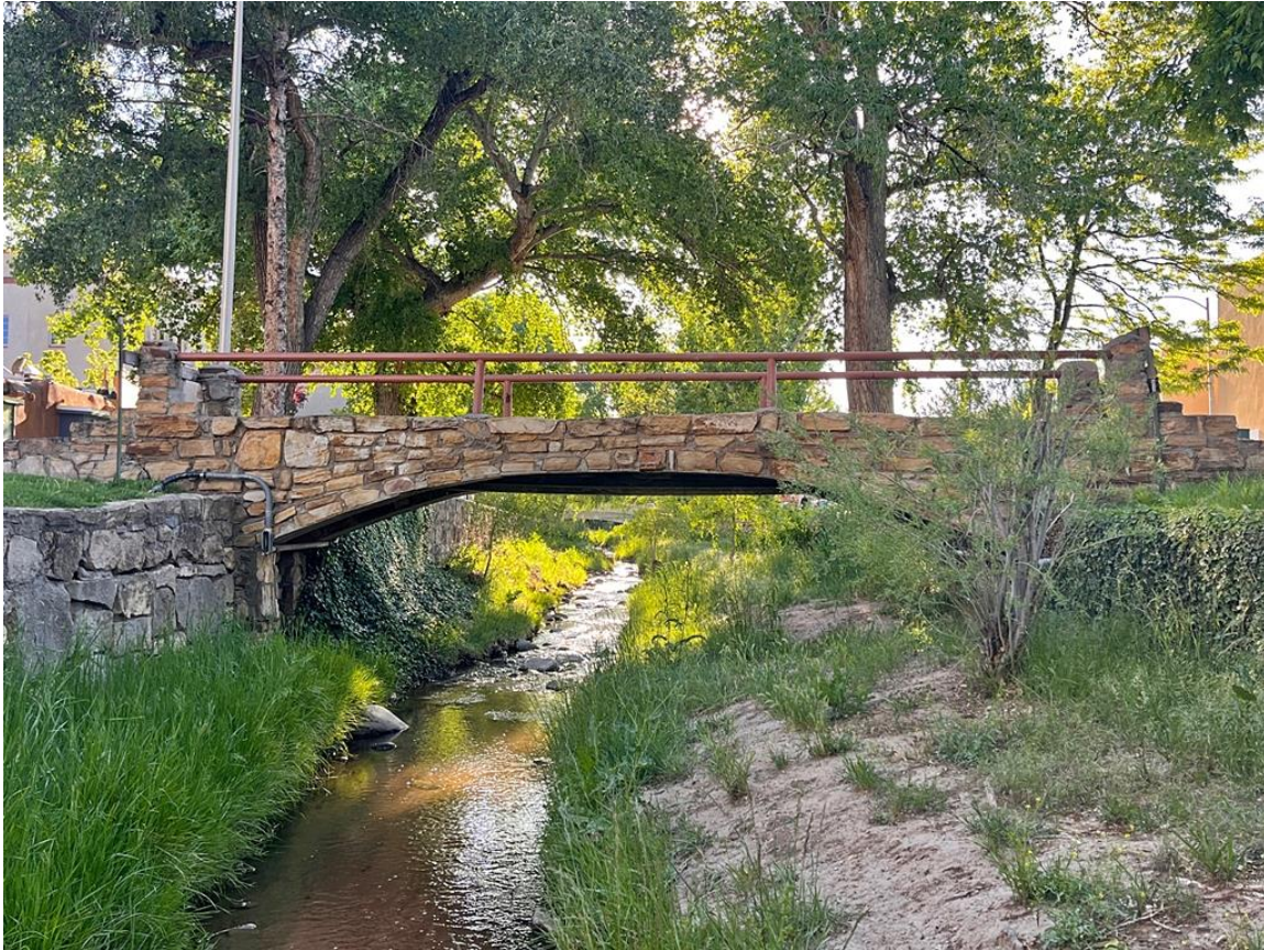
Photo 3: River and channel context. Camera facing west.
