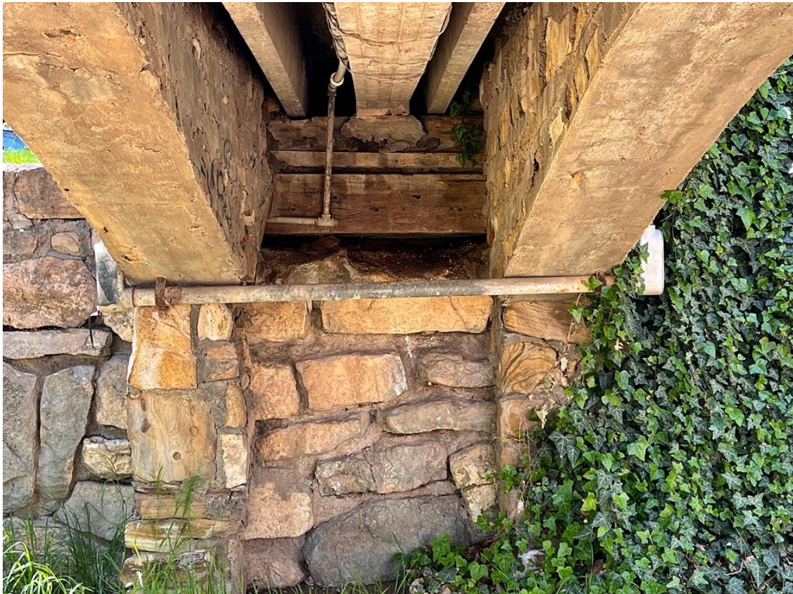
Photo 8: Substructure at south embankment stone abutment and bridge seat, and what appears to be timber support. Camera facing south.
