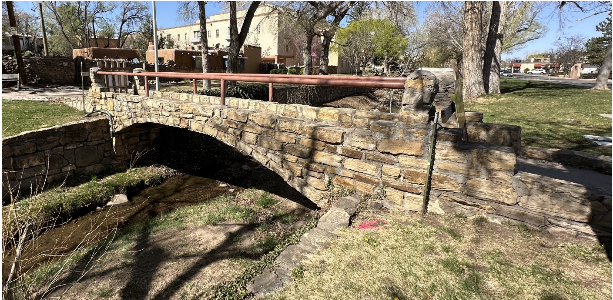
Figure 2 – Bridge elevation view
