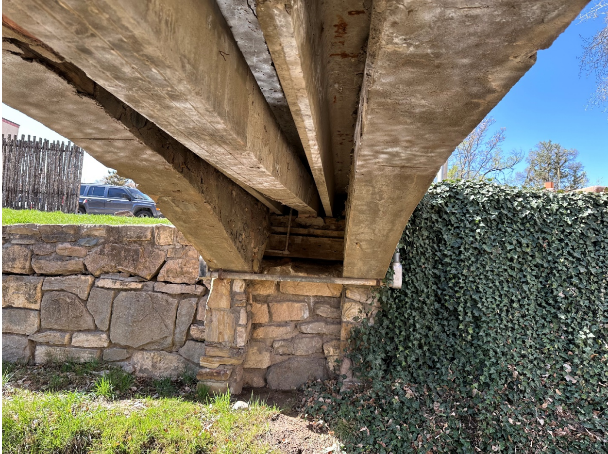
Figure 3 – Bridge superstructure configuration
