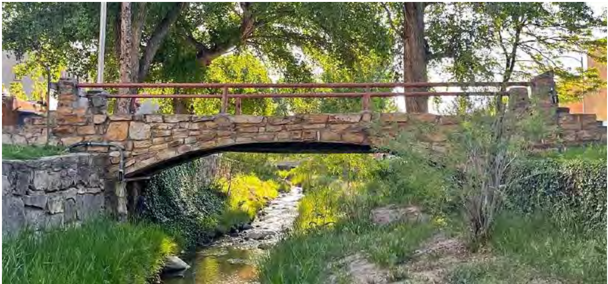
Figure 2: Side view of Shelby Street Footbridge
