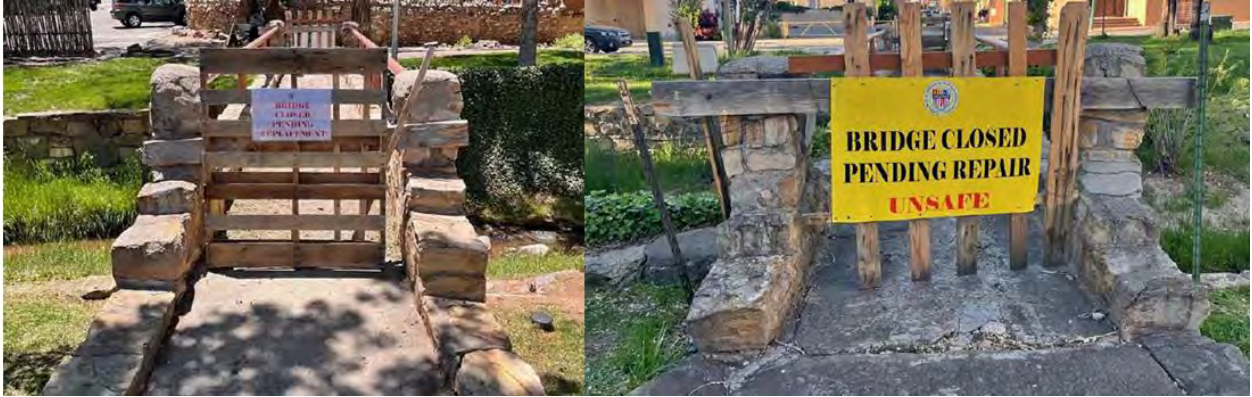
Figure 3: North and South Entrances to Shelby Street Footbridge.
