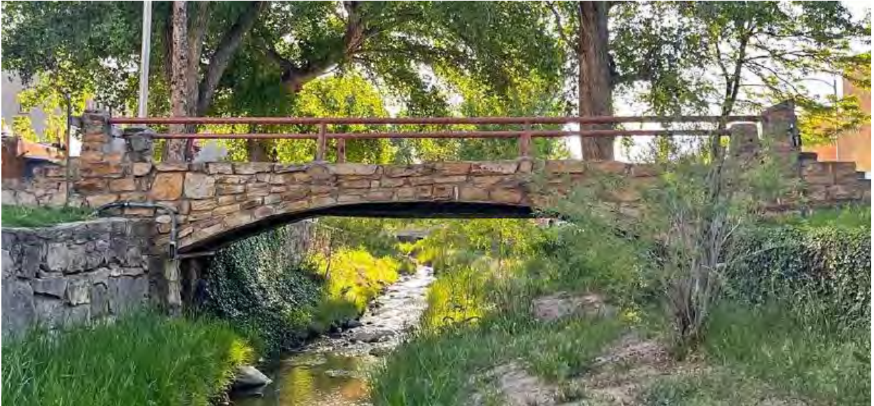
Figure 2: Side view of Shelby Street Footbridge
