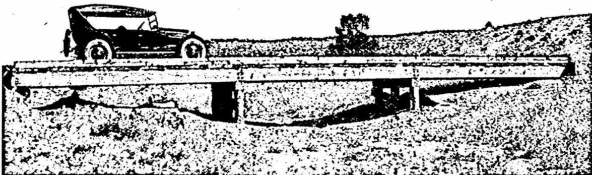
Fig. 1. Timber Bridge Construction by the New Mexico State Highway Department ( N.M. Highway Journal , November 1923)
