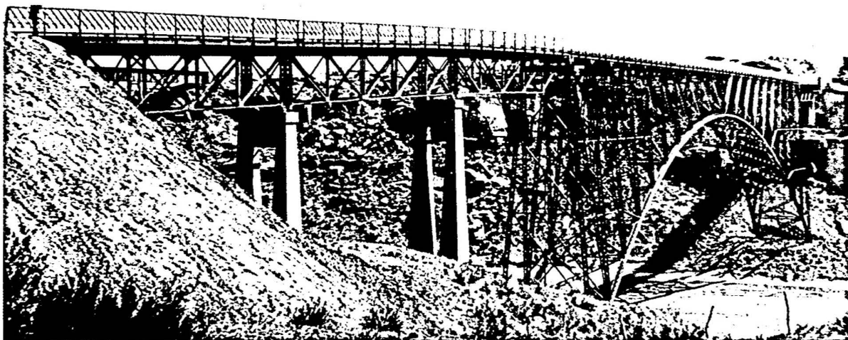
Fig. 13. Canadian River Bridge at Logan. This steel arch bridge was completed in 1922 as an early Federal-Aid Project. (Highway Department Bridge Files, Inactive)
