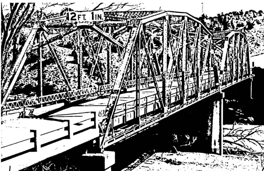
Fig. 35. San Francisco River Bridge (No. 599)
