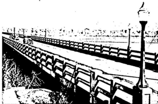
Fig. 24. Barelvas Bridge Across the Rio Grande at Albuquerque. Completed in 1928, the Barelvas Bridge included timber pilings, steel floor beams and a concrete deck. (Highway Department Bridge Files, Inactive)
