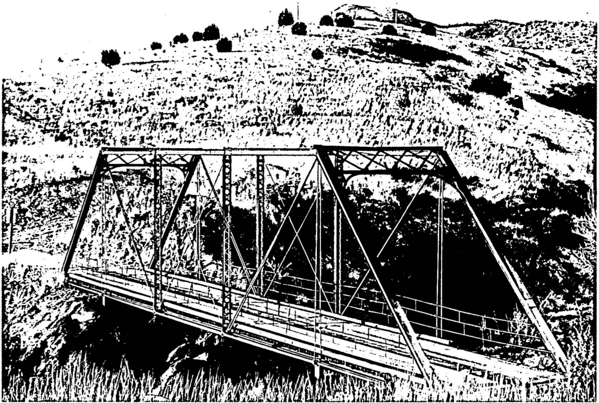
Fig. 31. Cold Spring Canyon Bridge (No. 1894)
