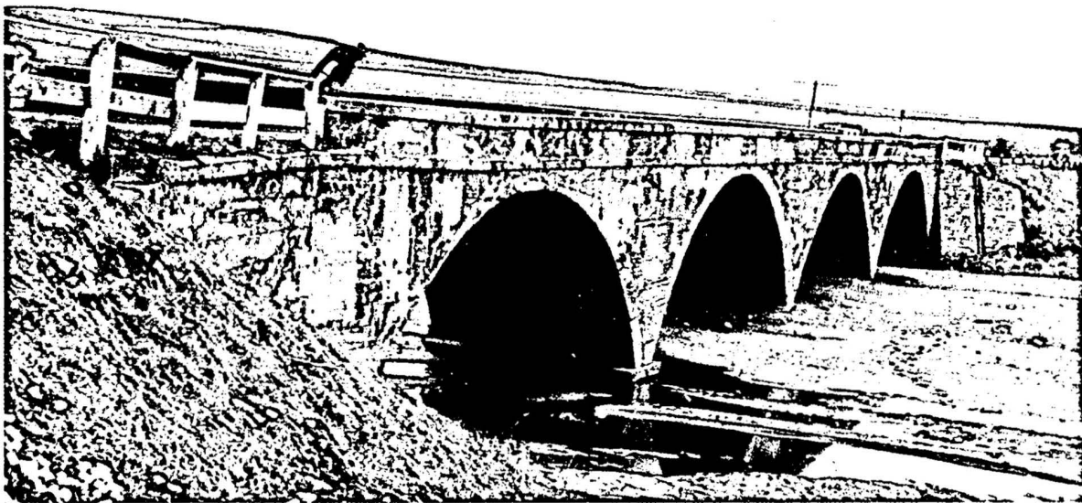
Fig. 11. Canadian River Bridge near Springer. Completed prior to 1916, this bridge was typical of the concrete arch construction used at several locations in the state. (Highway Department Bridge Files, Inactive)
