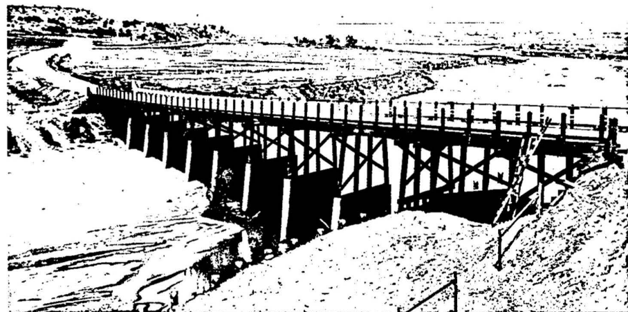
Fig. 20. Revuelto Creek Bridge East of Tucumcari. This bridge was completed on US 66 in 1931 using treated timber construction. (Highway Department Bridge Files, Inactive)
