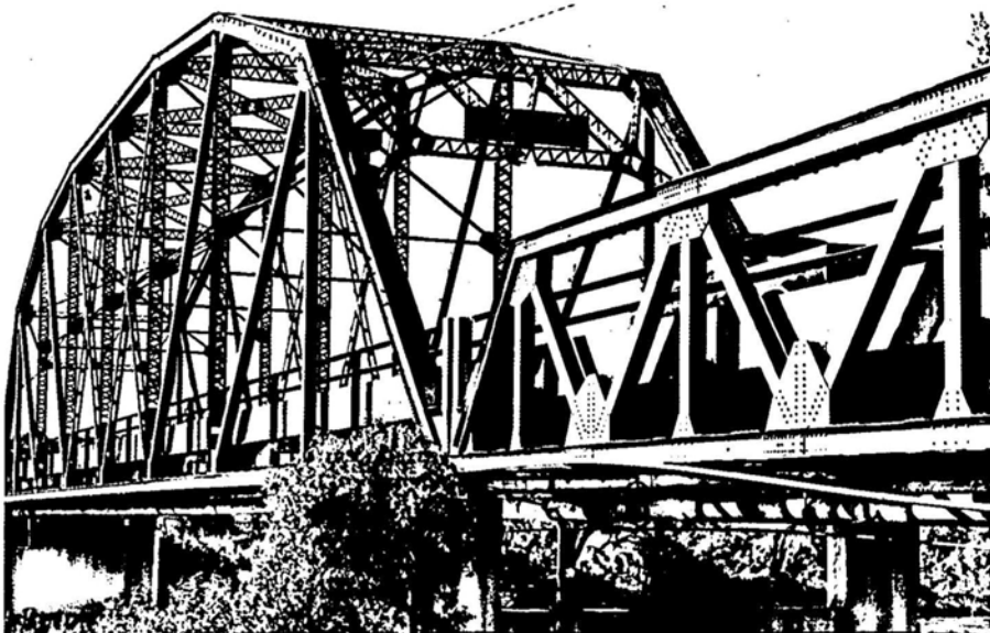
Fig. 36. Animas River Bridge at Aztec (No. 119)
