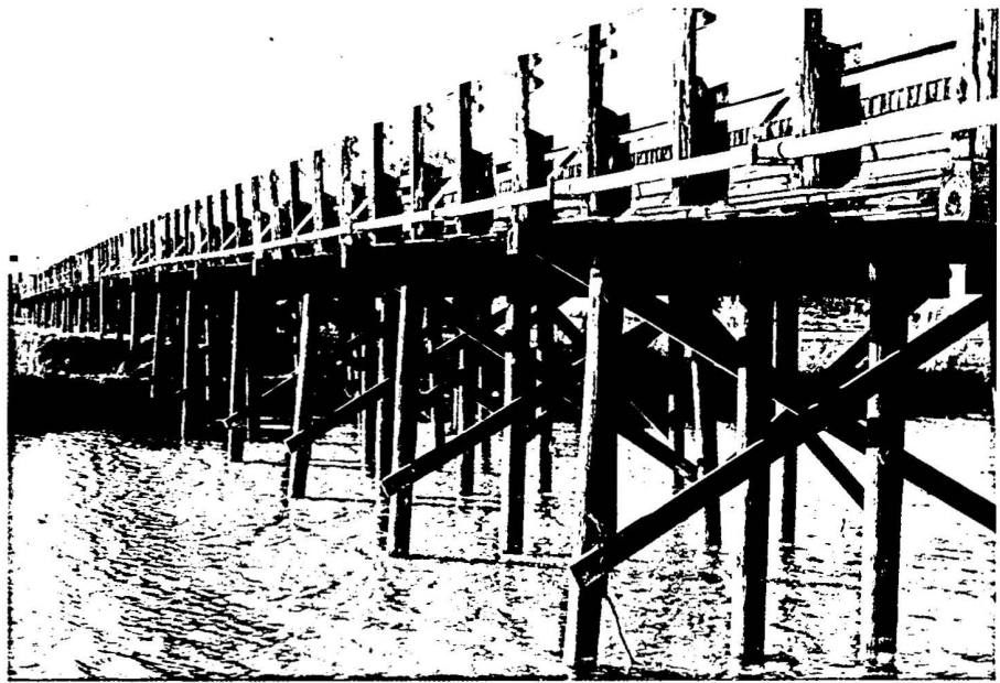
Fig. 60. Rio Grande Bridge near Arrey (No. 1669)
