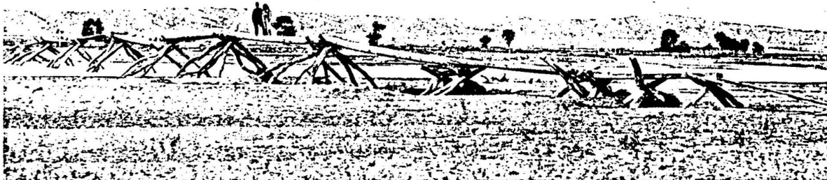
Fig. 6. Timber Footbridge Across the Rio Grande at Santo Domingo Pueblo in 1880. (Photograph by George C. Bennett, Courtesy of the Museum of New Mexico, Negative No. 2140)
