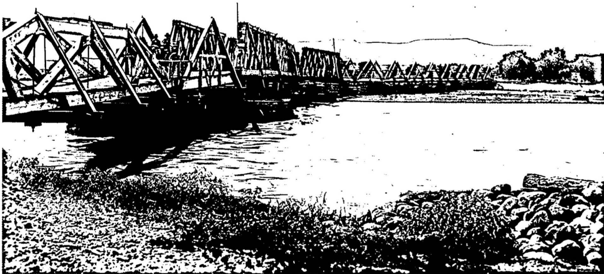
Fig. 8. Timber Truss Across the Rio Grande at Espanola About 1912. (Photograph Courtesy of the Museum of New Mexico, Negative No. 61684)
