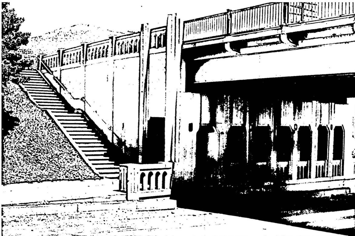
Fig. 62. North 1st Street Underpass, Raton (No. 5445)
