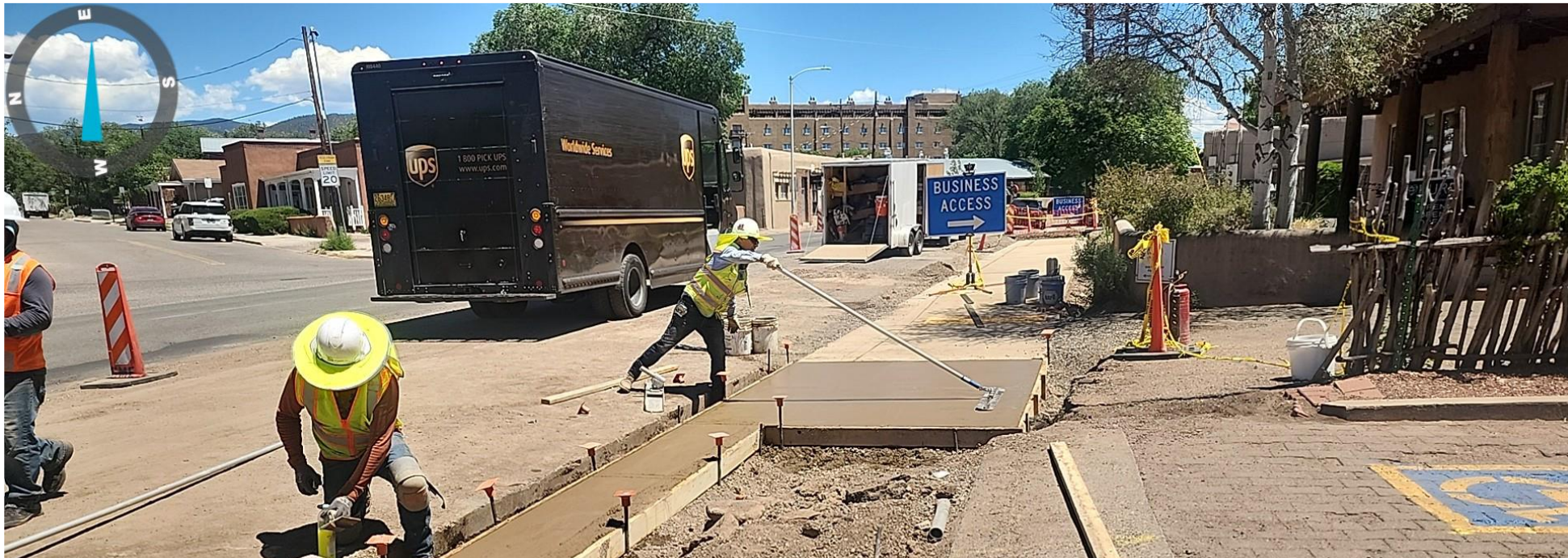
Road users navigating traffic controls through construction site.
