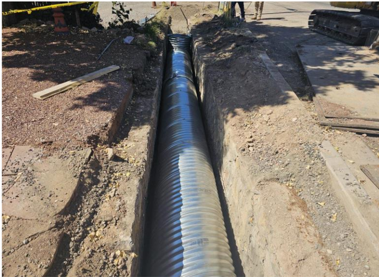
New storm water drainpipe
