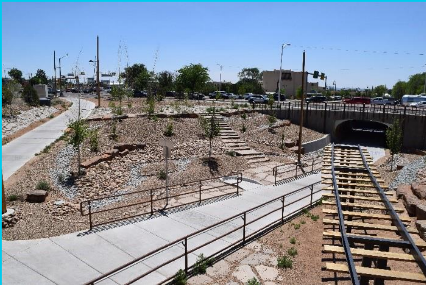
Green Infrastructure along Acequia Trail Underpass (Built 2017)
