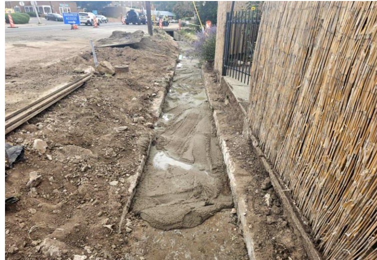
New concrete foundation
