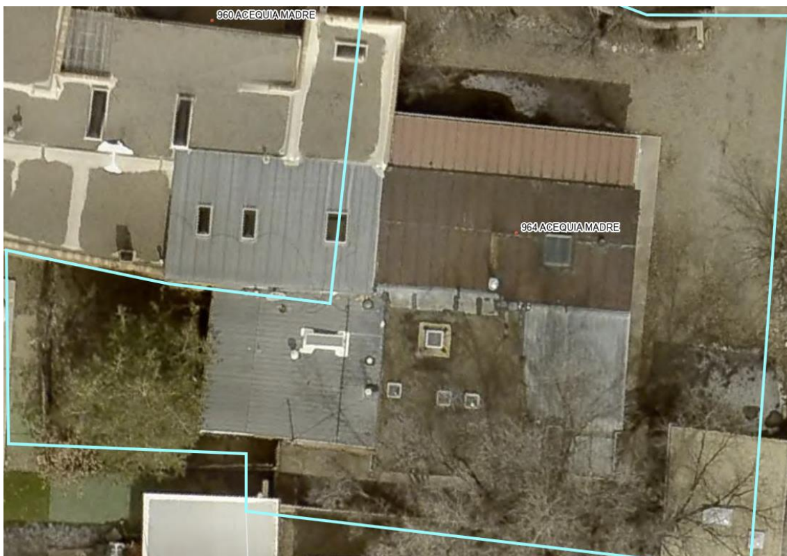
Figure 2. Current roof condition.
