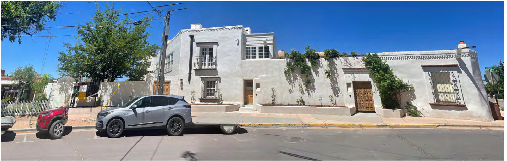
206 McKenzie Street Griffin Street / East Elevation
