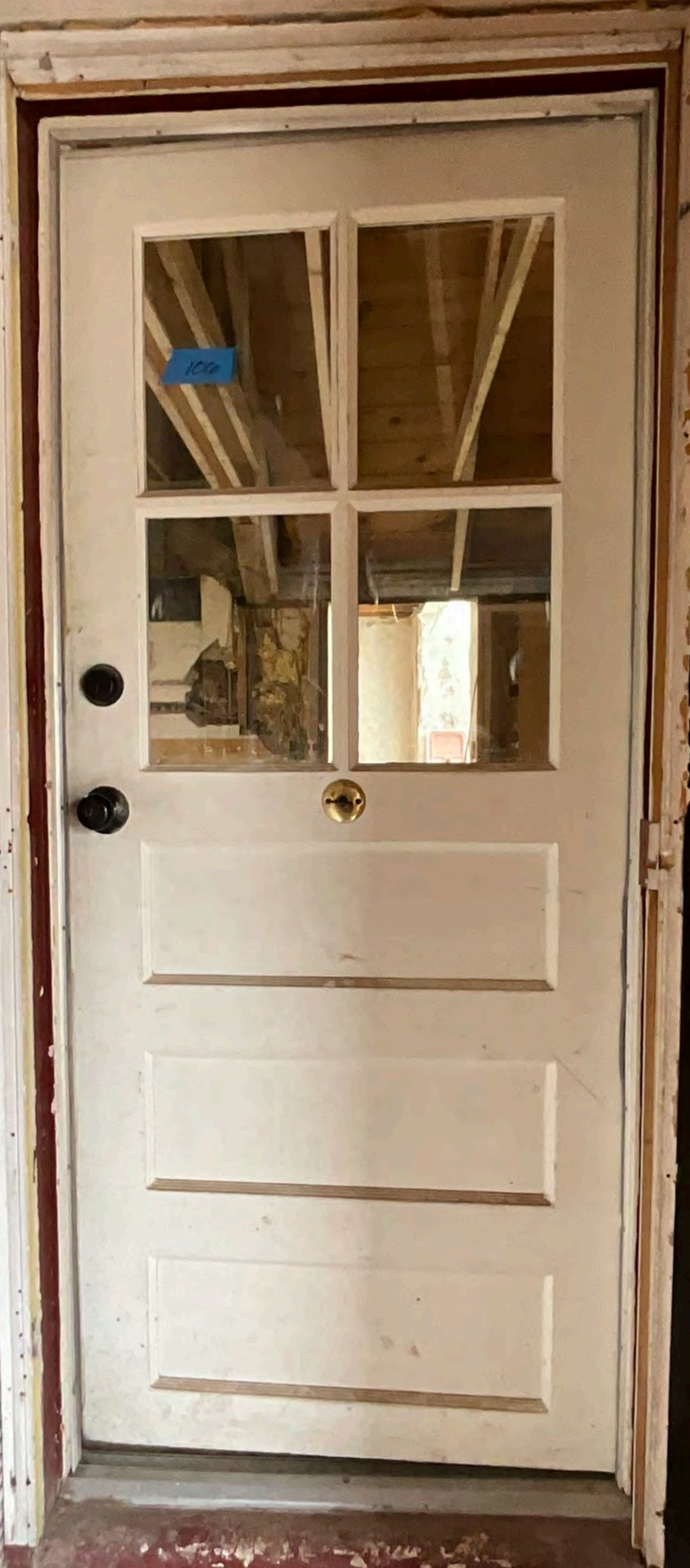
West Elevation Door #3
