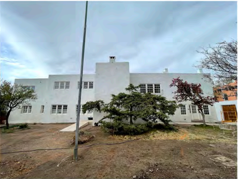
206 McKenzie St. South Elevation
