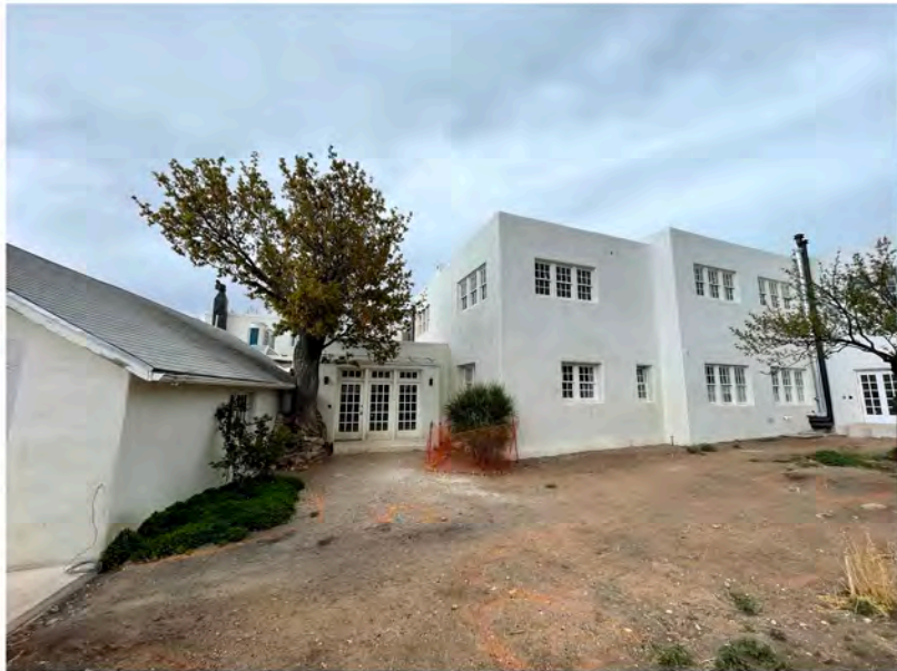
(Left side of South Elevation)
