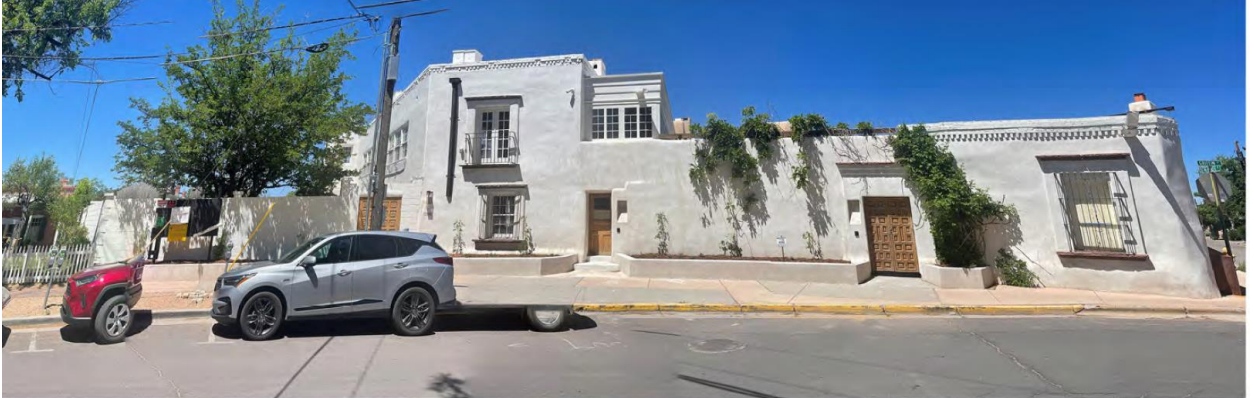
206 McKenzie Street Griffin Street / East Elevation
