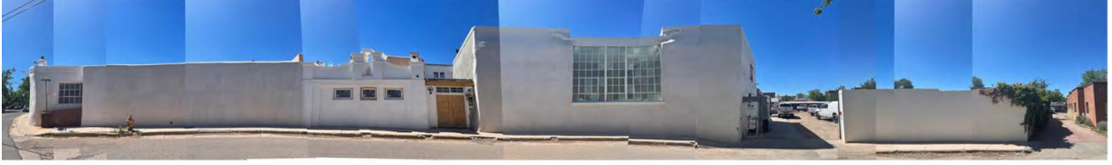
206 McKenzie Street McKenzie Street / North Elevation
