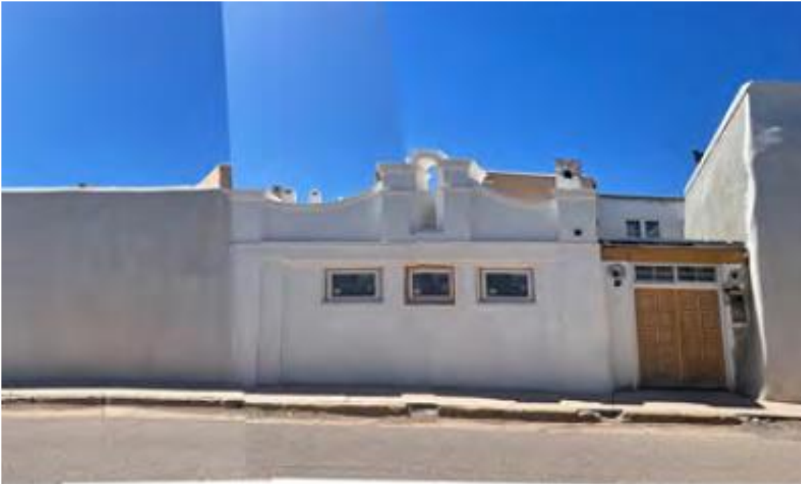
Figure 4. North Primary Facade.
