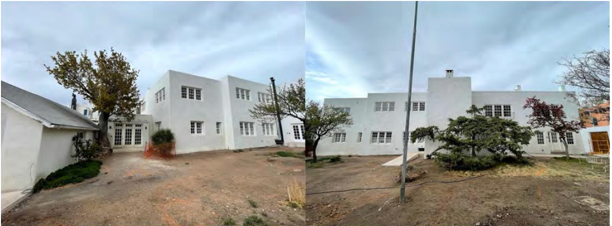
(Left side of South Elevation)
