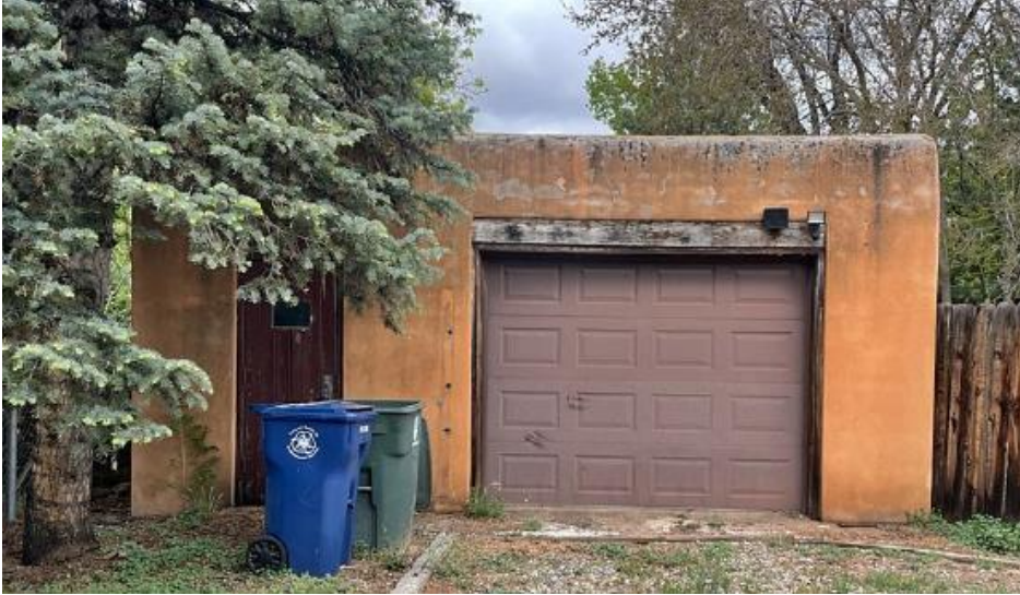
Figure 4: South Elevation of Accessory Structure
