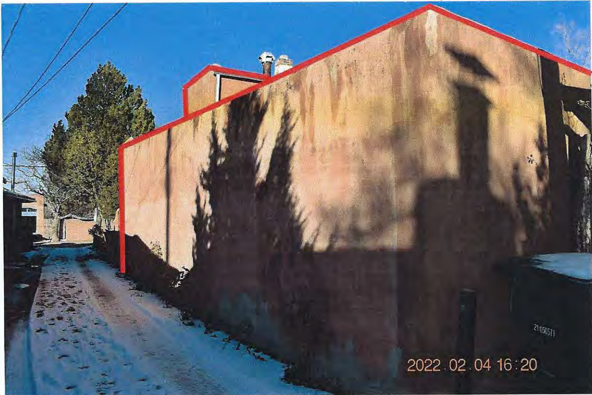
Photo 7: West elevation and portion of south exterior wall. Camera facing northeast.
