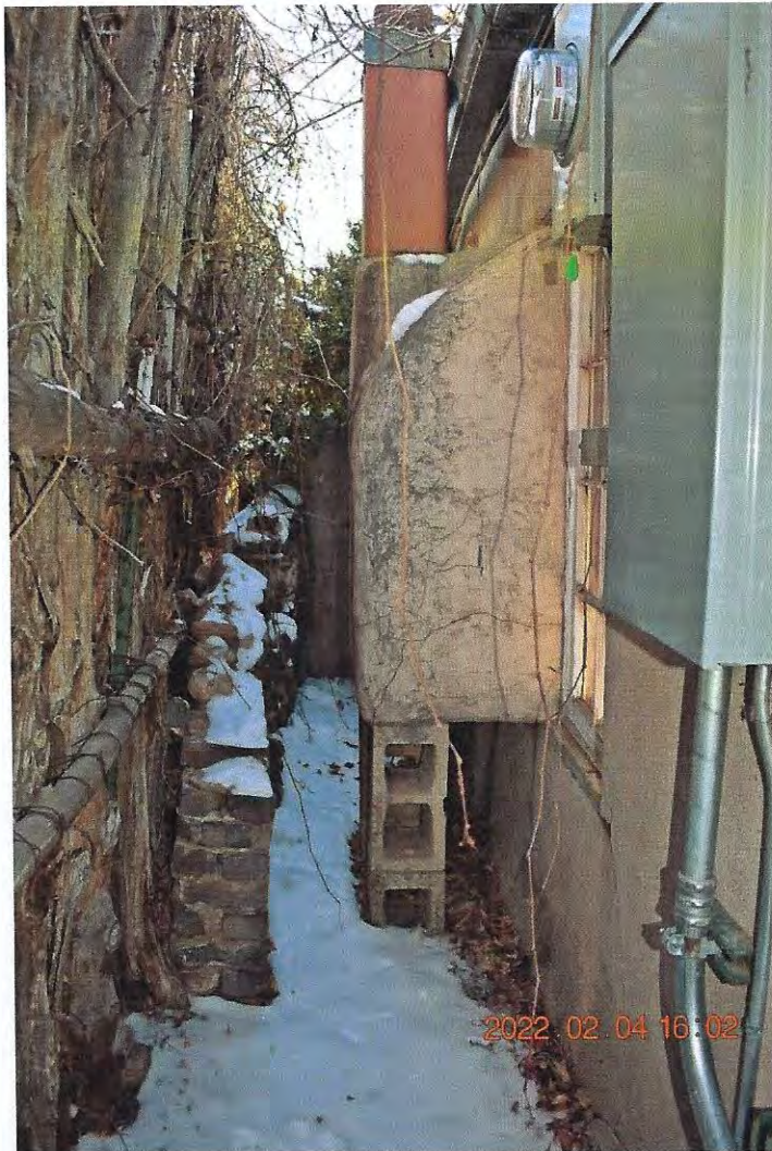
Photo 12: East elevation. Stovepipe and window. Camera facing south.
