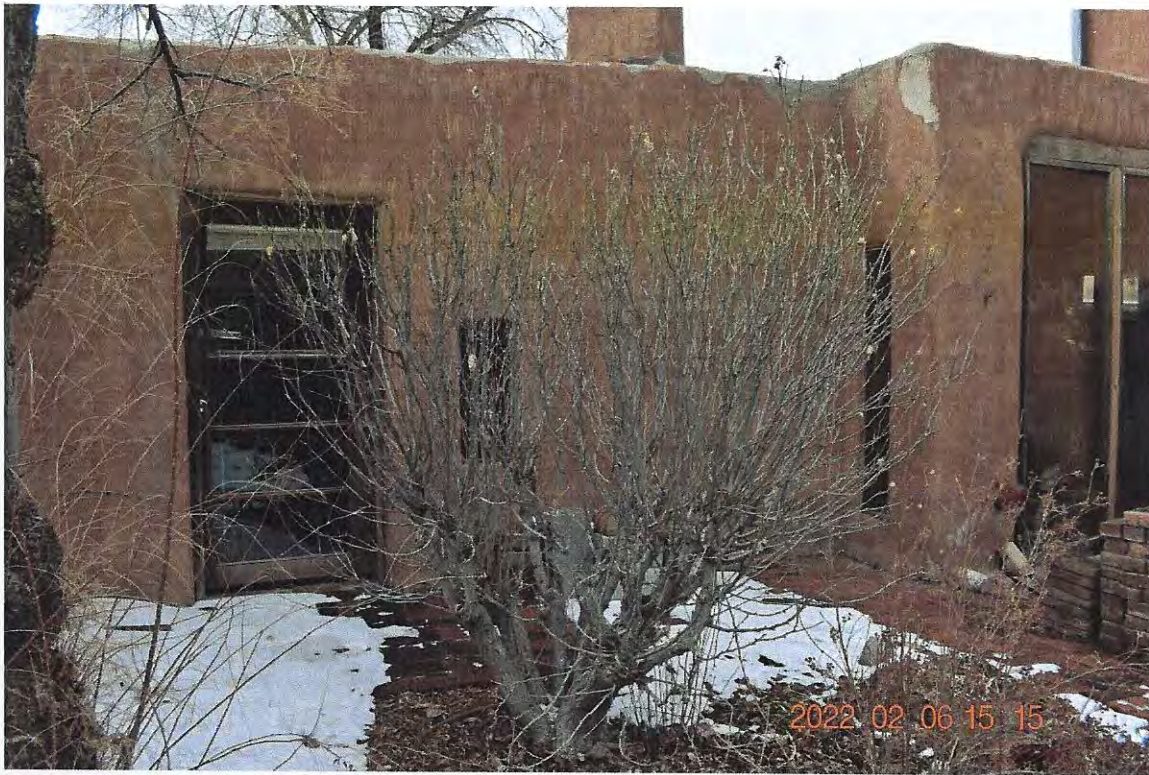
Photo 10: Courtyard - partial east elevation. Storage room entry. Camera facing west.
