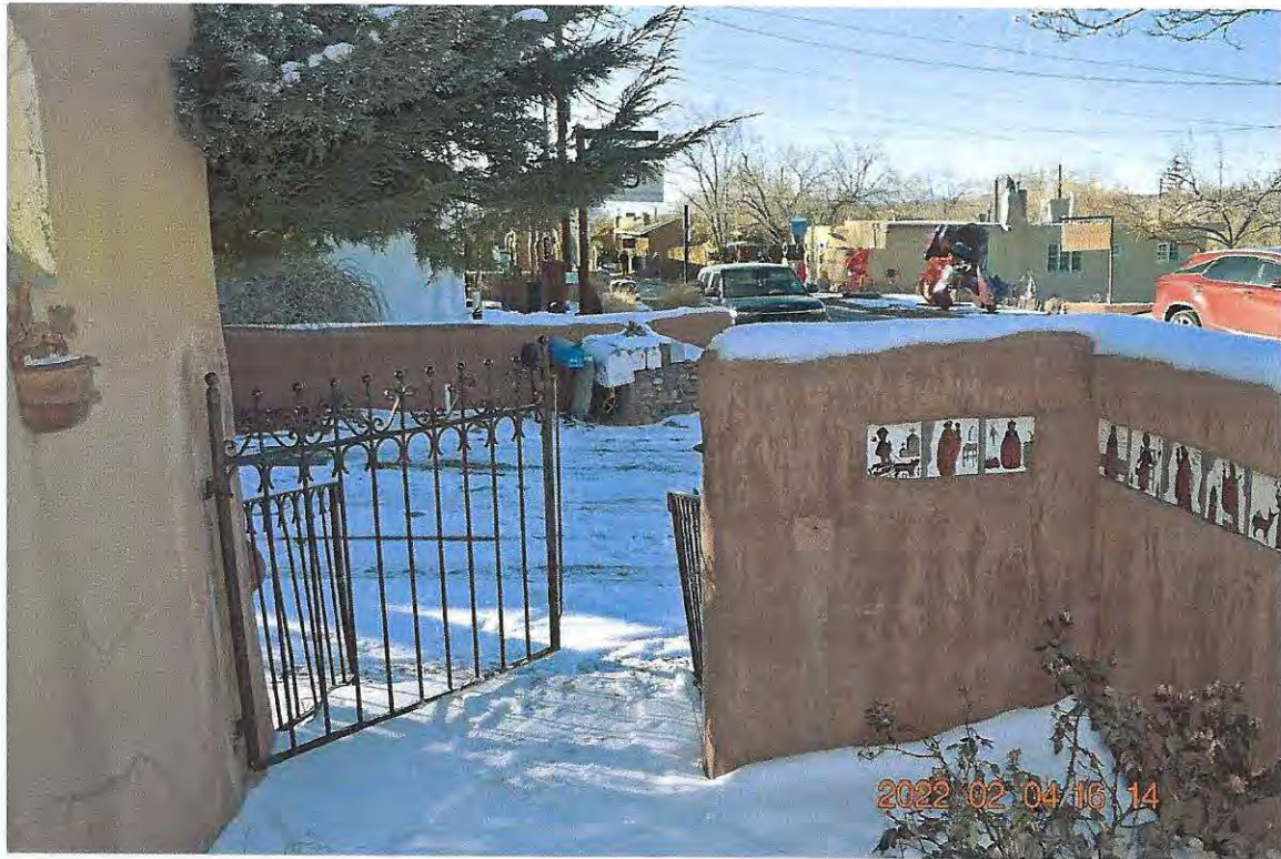
Photo 13: Front Courtyard Wall. Camera facing northwest.
