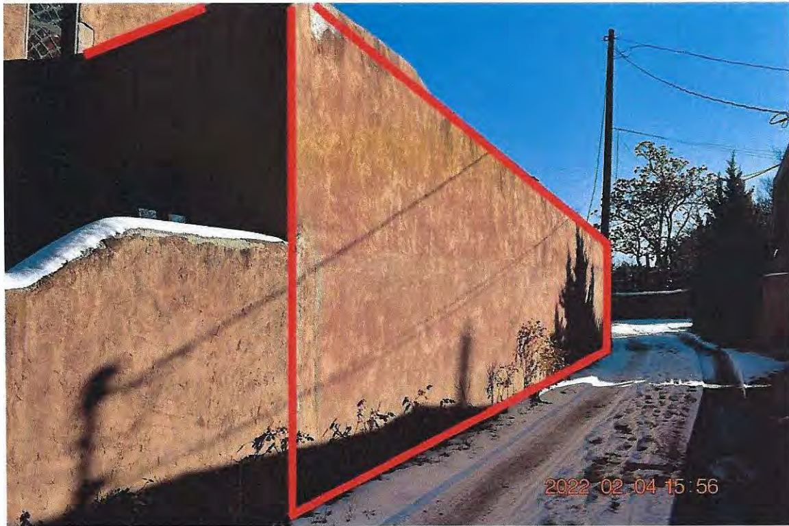
Photo 6: West elevation, 1968 addition. Camera facing south.
