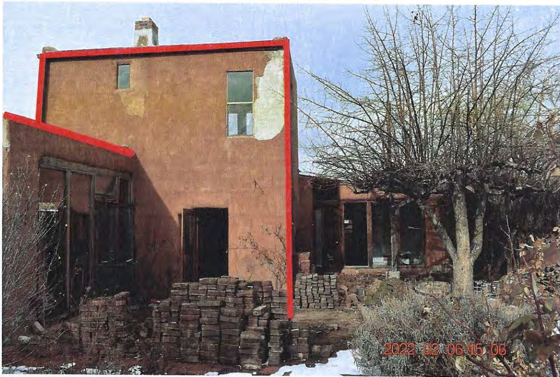
Photo 8: Courtyard - partial east and south elevations. Red indicates 1968 addition. Camera facing north.
