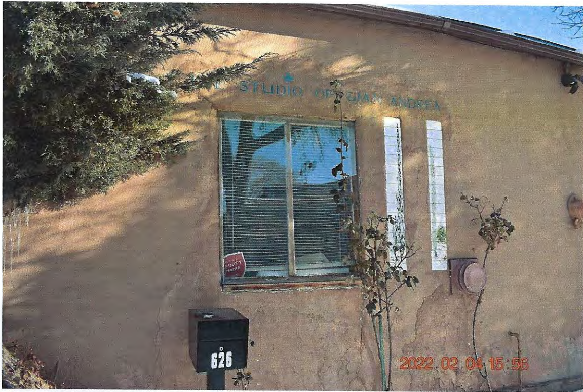
Photo 3: West elevation. Older portion, north end. Camera facing southeast.
